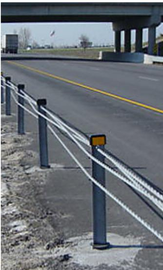
Although several different high-tension cable barrier types exist, they all use the same cable that consists of 3/4-inch-diameter galvanized steel cable with 3x7 (21 wires) construction.
