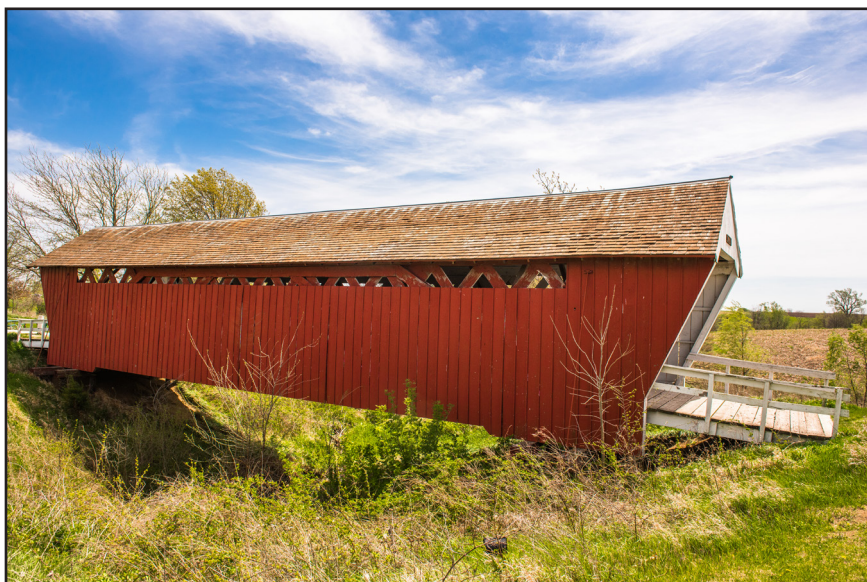
Imes Covered Bridge (1870-1871)
