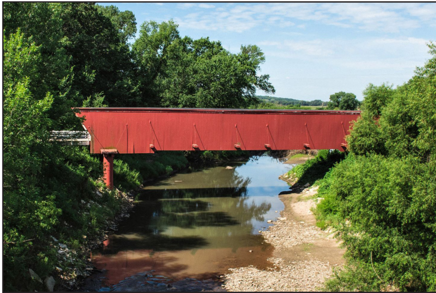
Holliwell Covered Bridge (1880)
