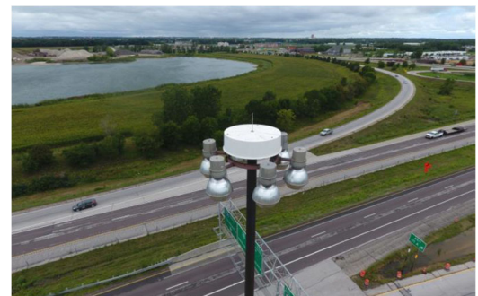
Figure 12. CCTV Camera Installation
