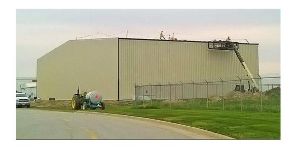
George C. Ford/The Gazette Construction of a 12,000-square-foot hangar for Kinze Manufacturing at The Eastern Iowa Airport is scheduled for completion by July 31. Three walls have been completed, and the roof has been installed. On May 31, Eastern Iowa Excavating will begin constructing a taxiway connector and apron.
