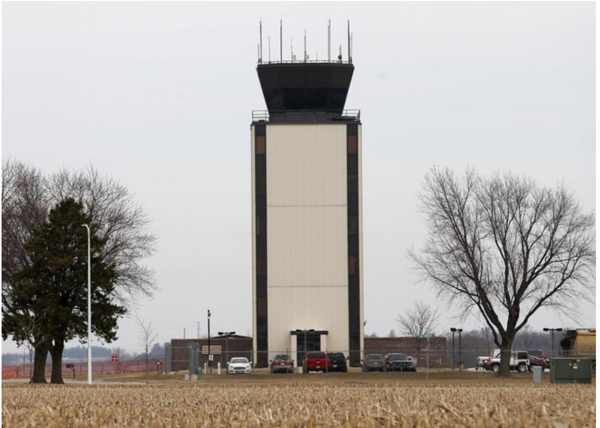
Waterloo Regional Airport air traffic control tower as shown Thursday.
