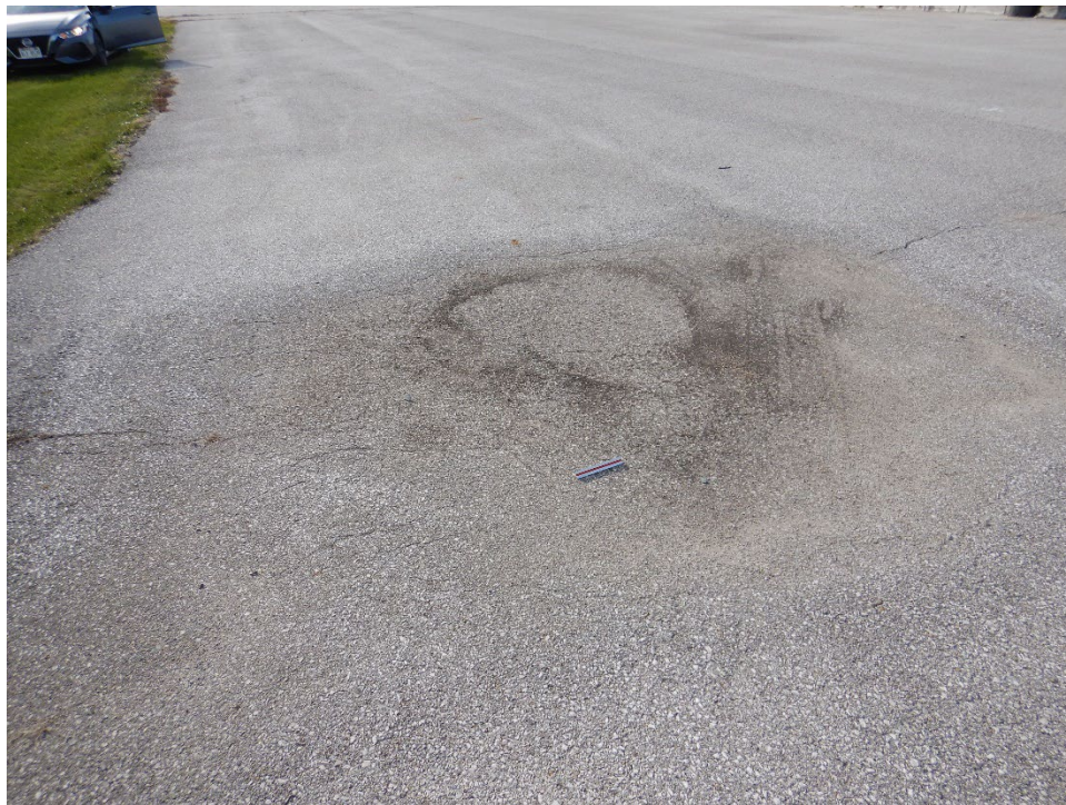
A01AL-03. Depression (Sample Unit No. 02).
