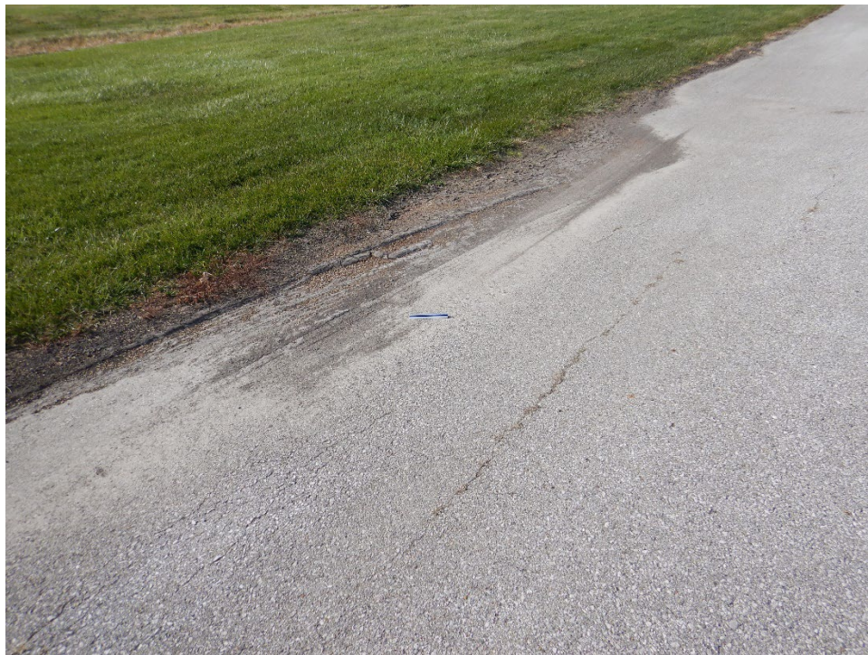
A01AL-02. Depression (Sample Unit No. 01).
