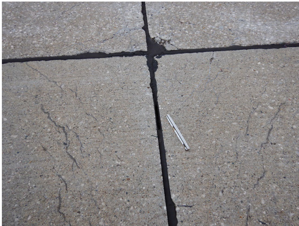
T02AN-01. ASR (Sample Unit No. 03) (2).
