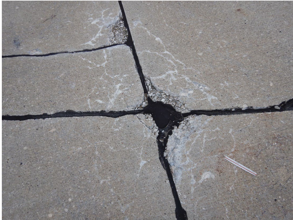
R18AN-01. ASR (Sample Unit No. 81).
