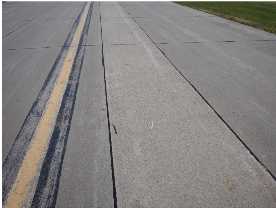
T06AN-01. Large Patching (Sample Unit No. 15).
