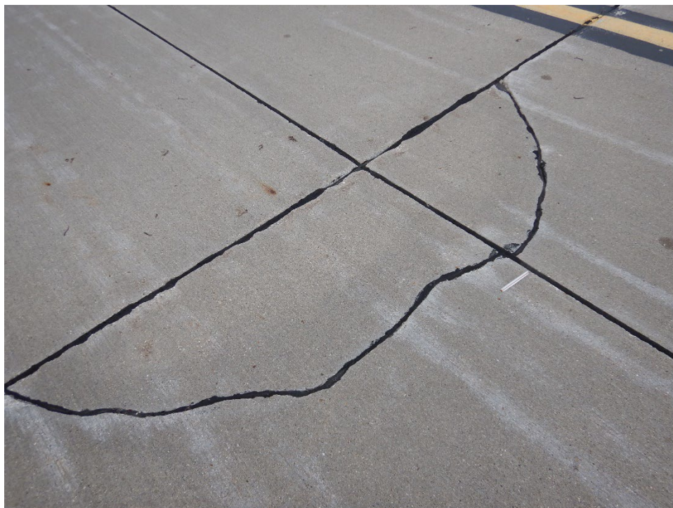
T07AN-01. Corner Break (Sample Unit No. 04).
