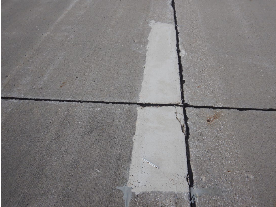
T08AN-01. Small Patching (Sample Unit No. 04).
