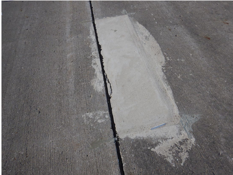
T09AN-01. Large Patching (Sample Unit No. 07).
