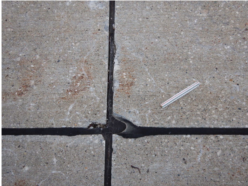
R18AN-01. ASR (Sample Unit No. 27).
