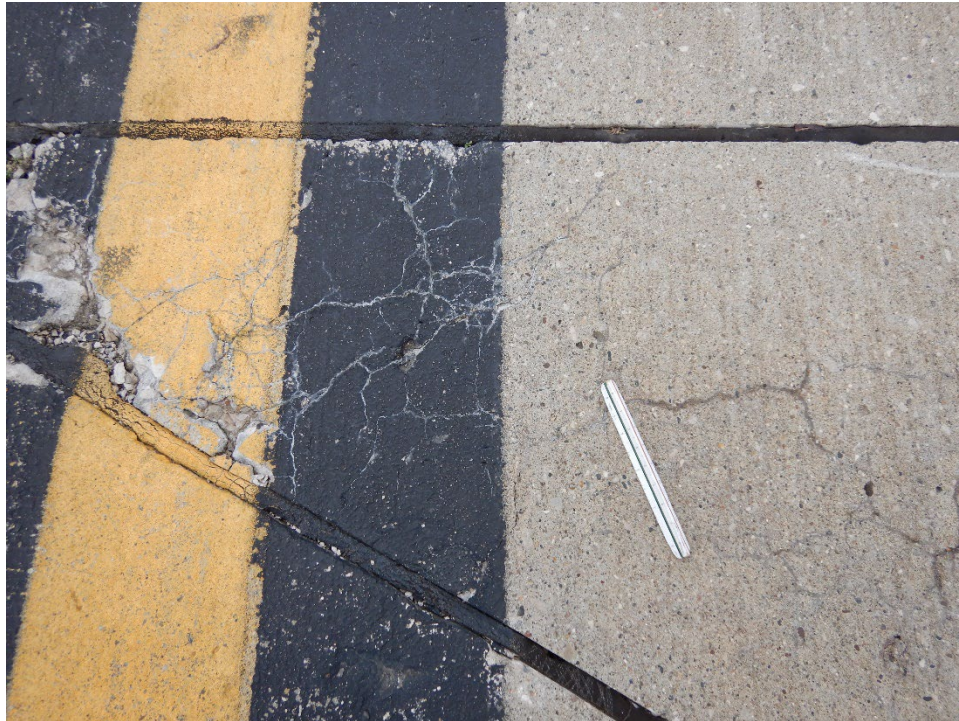
T02AN-01. ASR (Sample Unit No. 03) (1).
