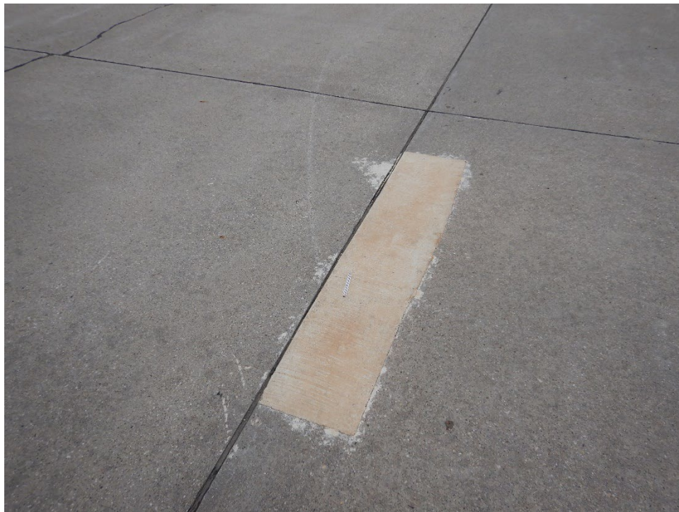
TH01AN-02. Large Patching (Sample Unit No. 18).
