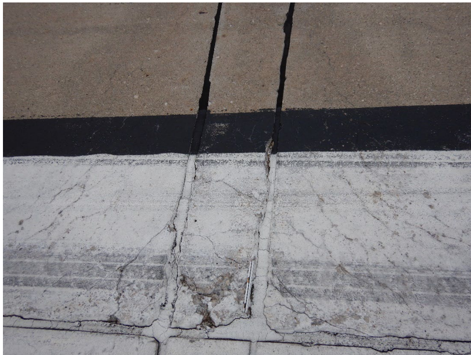
R18AN-01. ASR (Sample Unit No. 09).
