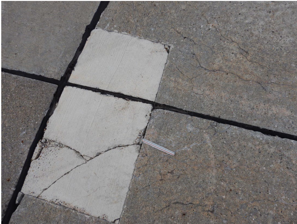
T03AN-01. Small Patching (Sample Unit No. 02).
