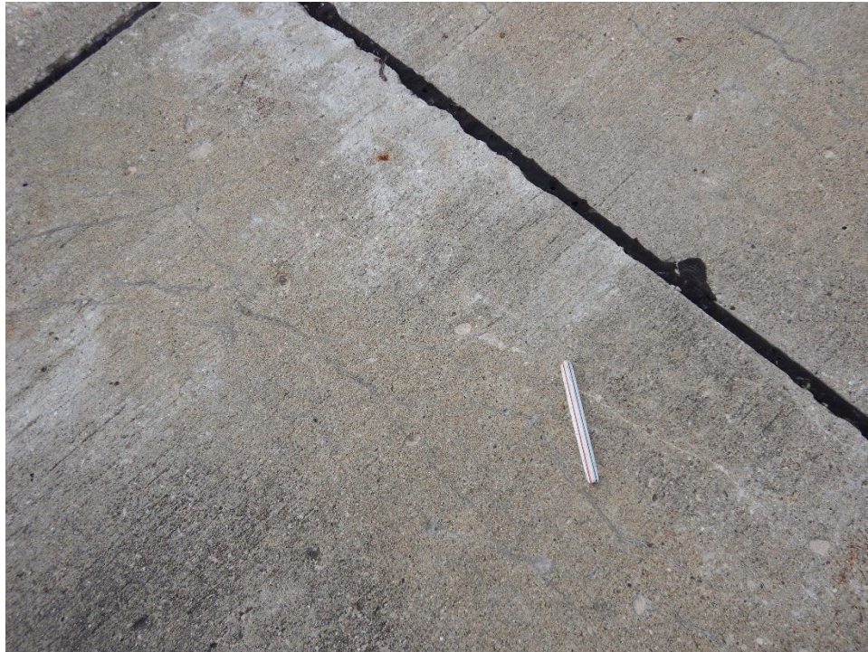
T05AN-01. ASR (Sample Unit No. 05).
