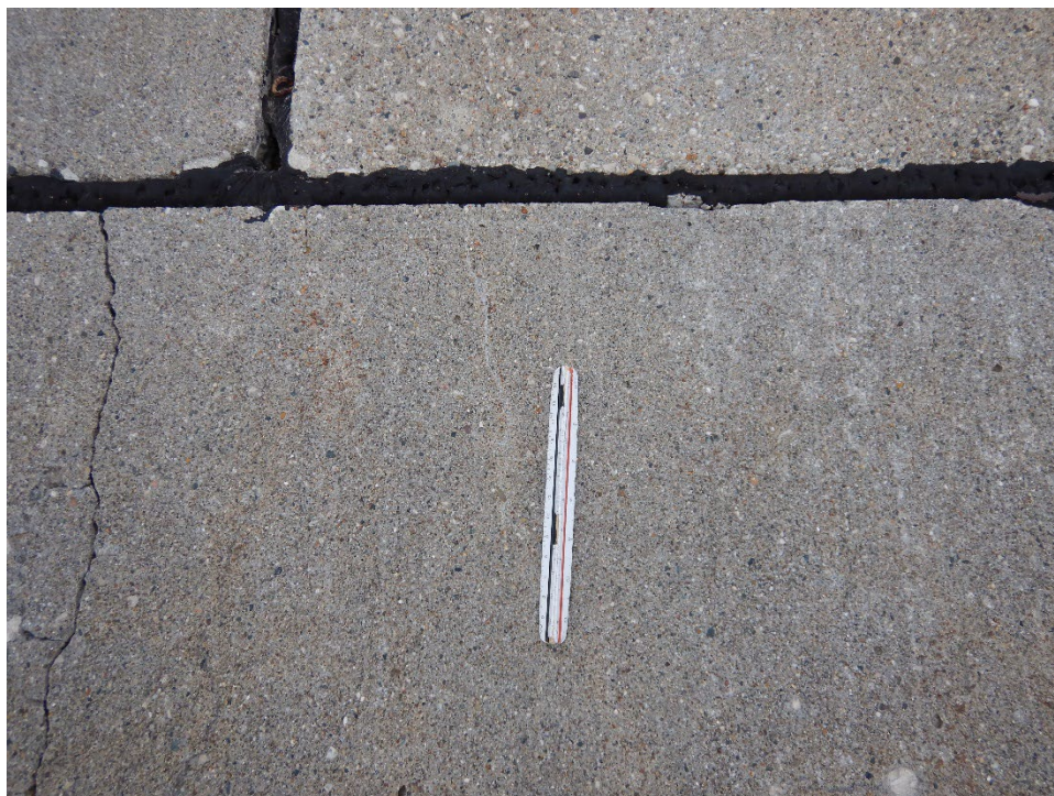
T06AN-01. ASR (Sample Unit No. 15).
