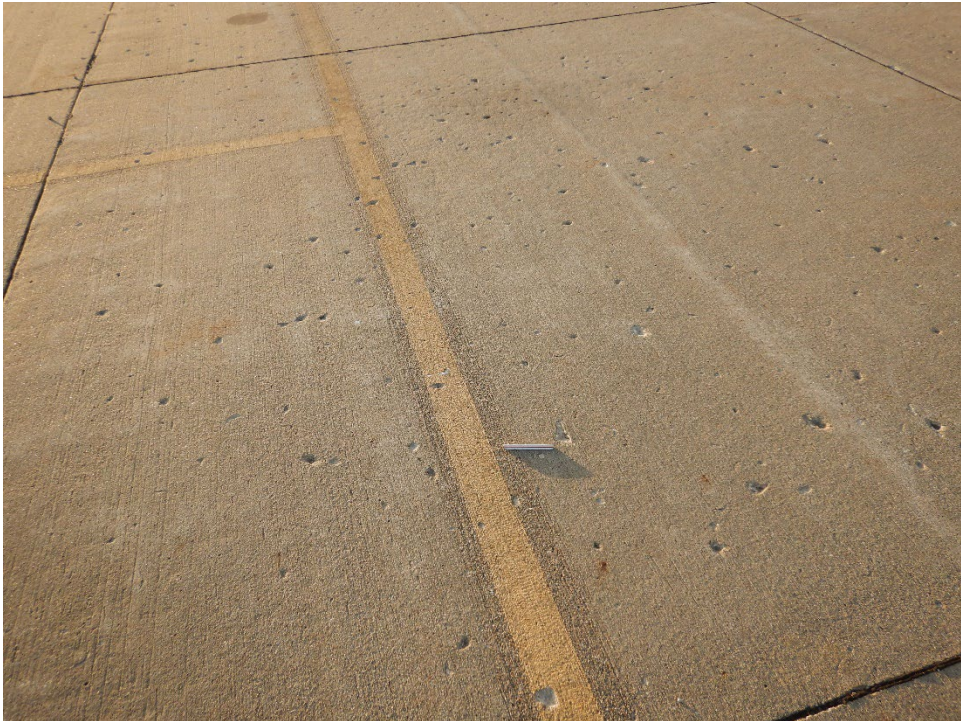
A01AN-02. Popouts (Sample Unit No. 12).
