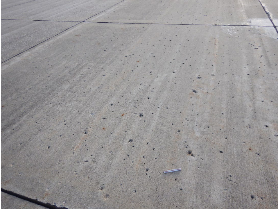
R04AN-02. Popouts (Sample Unit No. 04).
