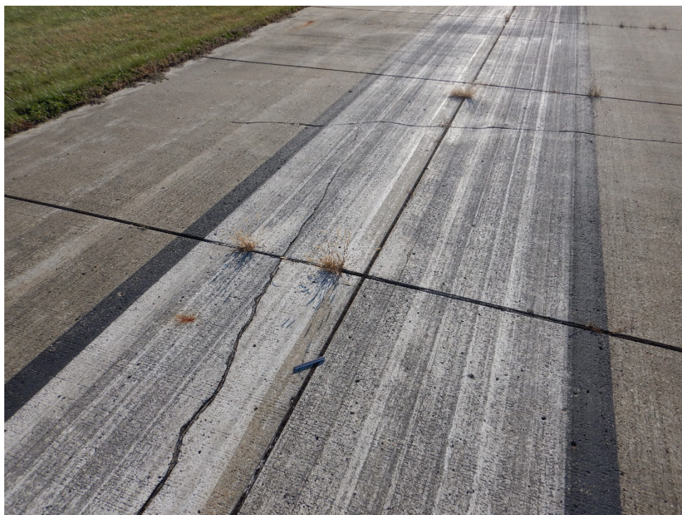
R14AU-02. LTD Cracking (Sample Unit No. 14).
