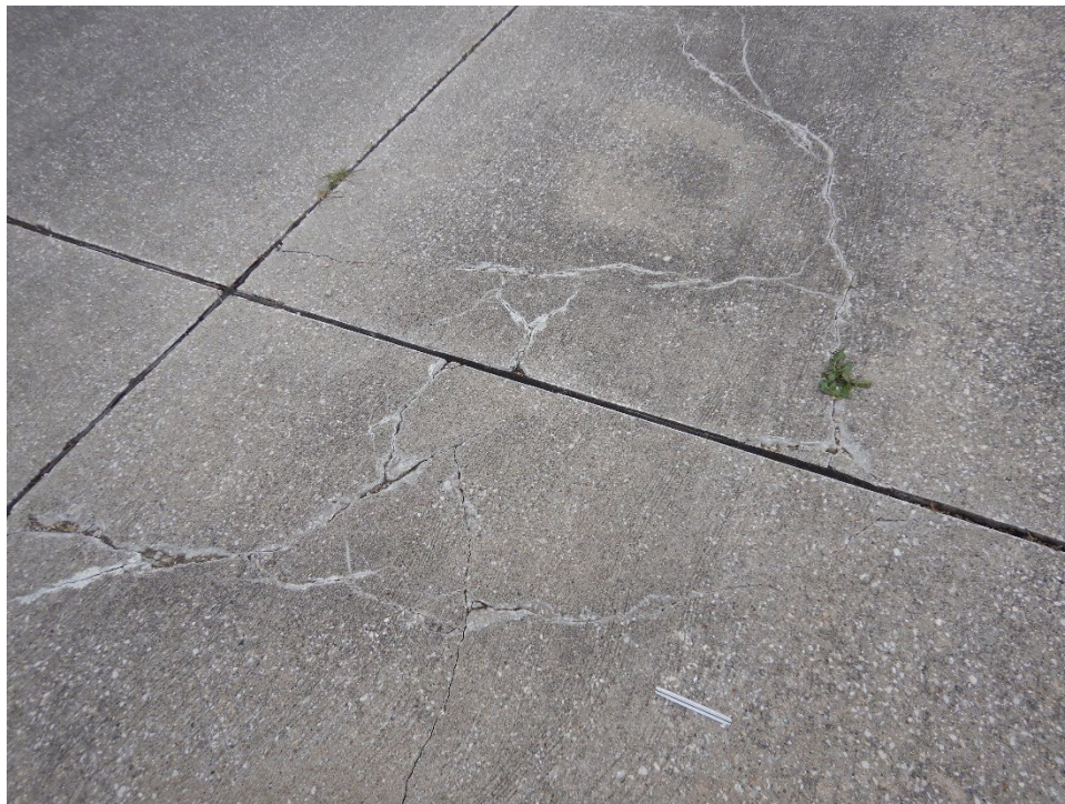
A01BP-01. Shattered Slab (Sample Unit No. 14).
