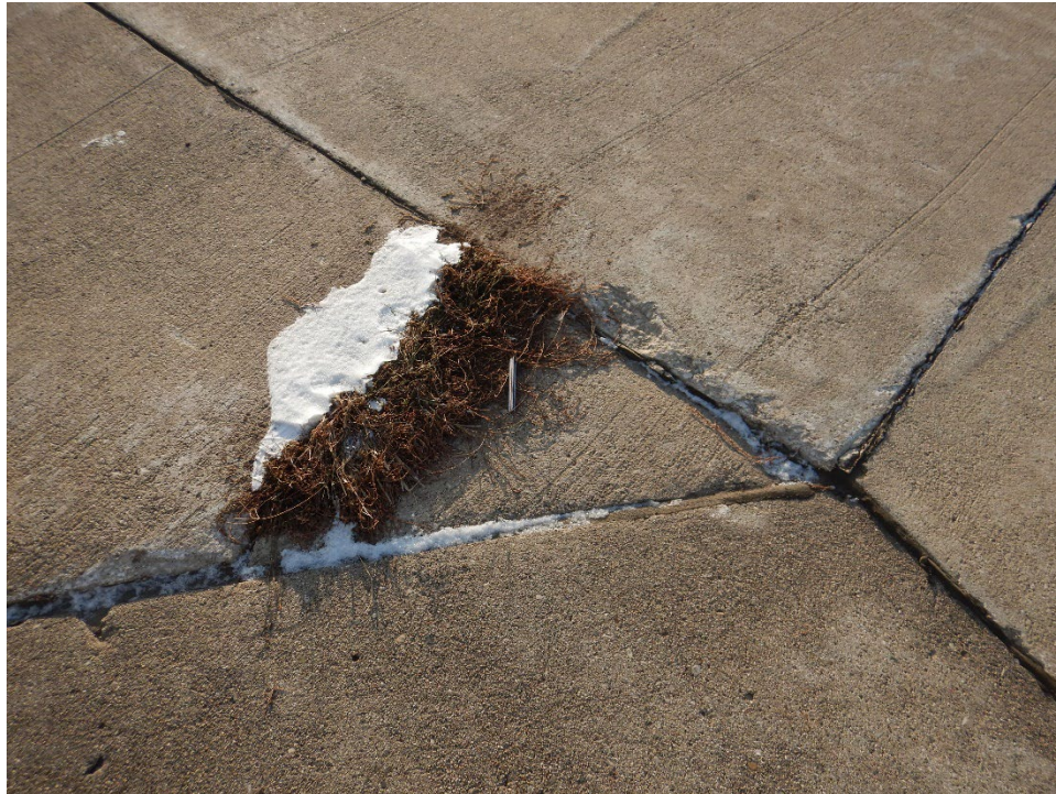
TH01CK-01. Corner Break (Sample Unit No. 03).
