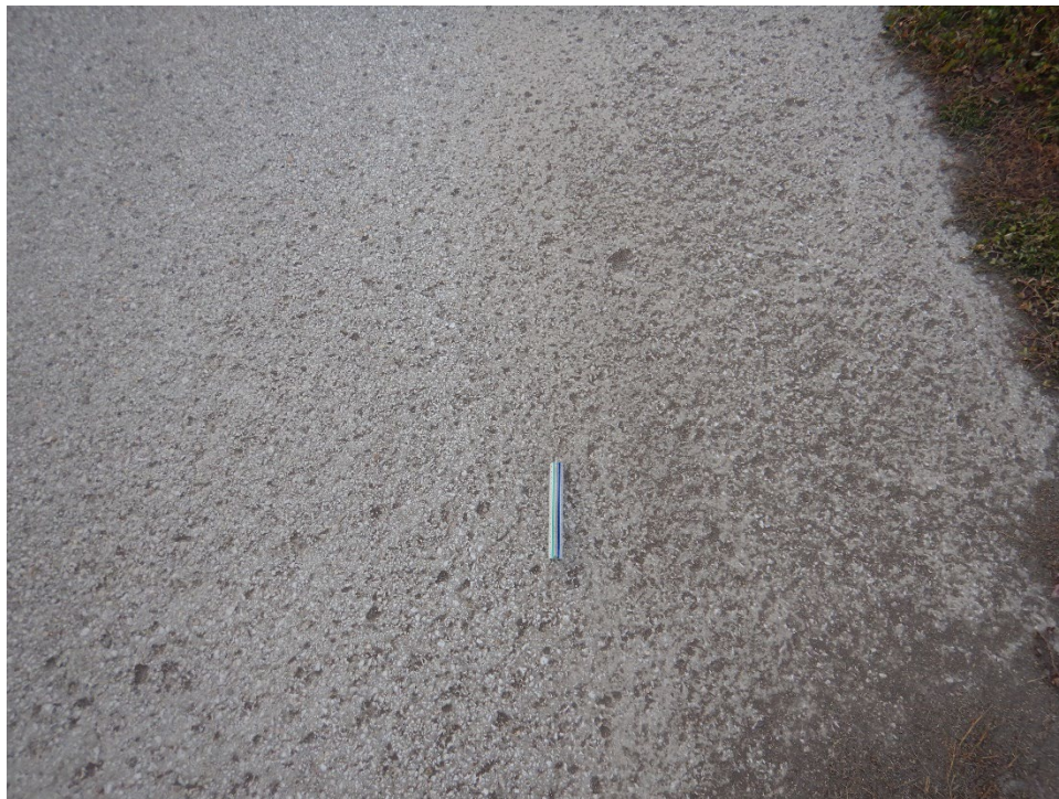
TH01CD-01. Raveling (Sample Unit No. 04).
