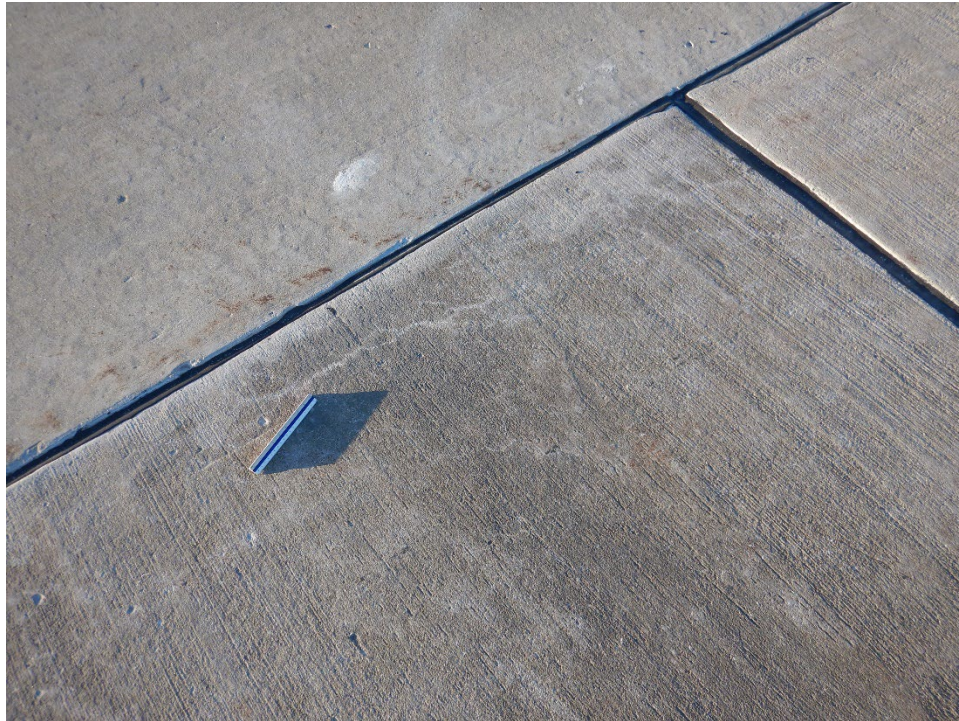
T01CD-01. ASR (Sample Unit No. 07).
