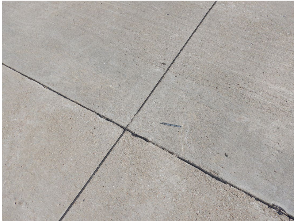
A02CB-01. ASR (Sample Unit No. 22).
