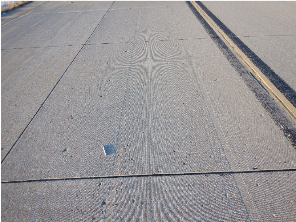
T03CB-02. Popouts (Sample Unit No. 17).
