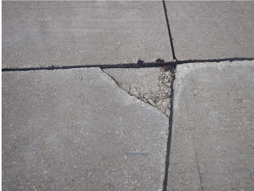
TH01DE-01. Corner Break (Sample Unit No. 04).
