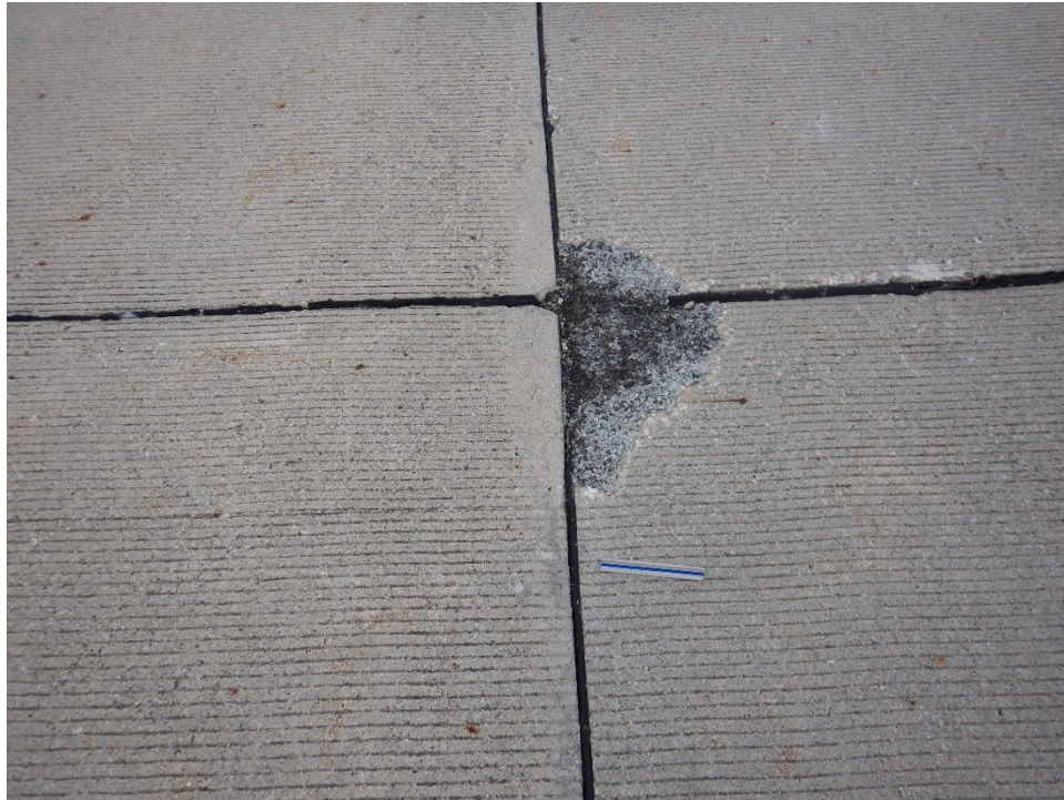
R12DN-01. Small Patching (Additional Sample Unit No. 36).
