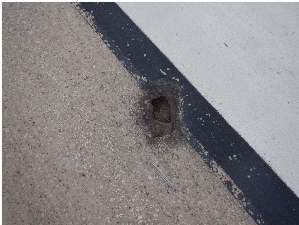
R18FA-01. Small Patching (Additional Sample Unit No. 173).
