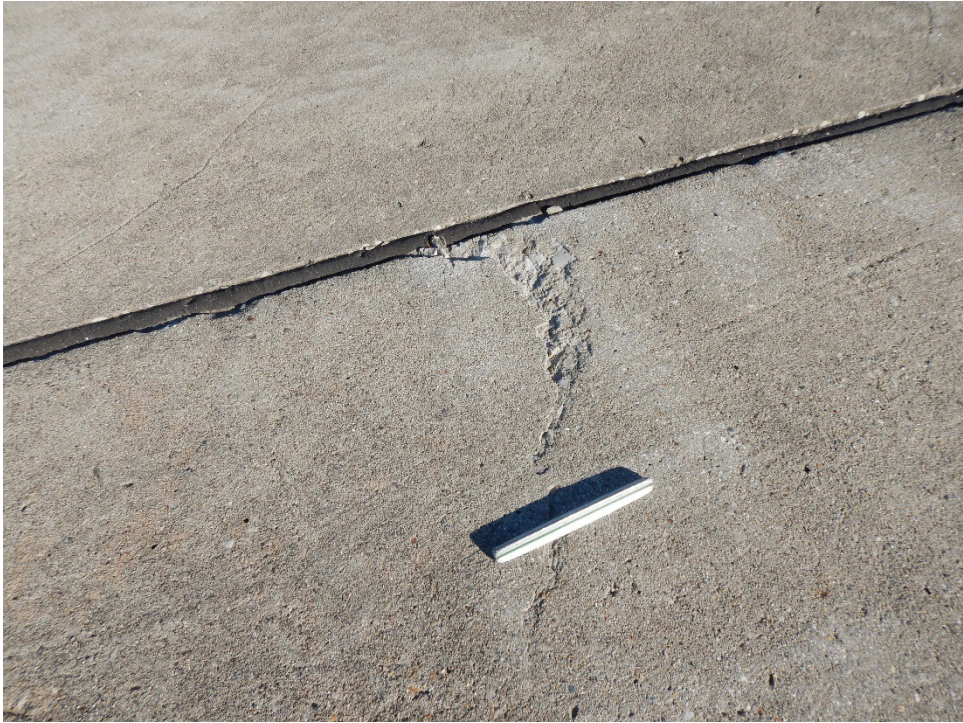
TH01FA-03. Scaling (Sample Unit No. 01).
