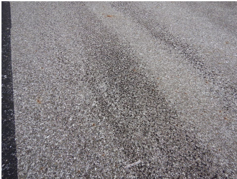
T02FC-01. Bleeding (Sample Unit No. 02).
