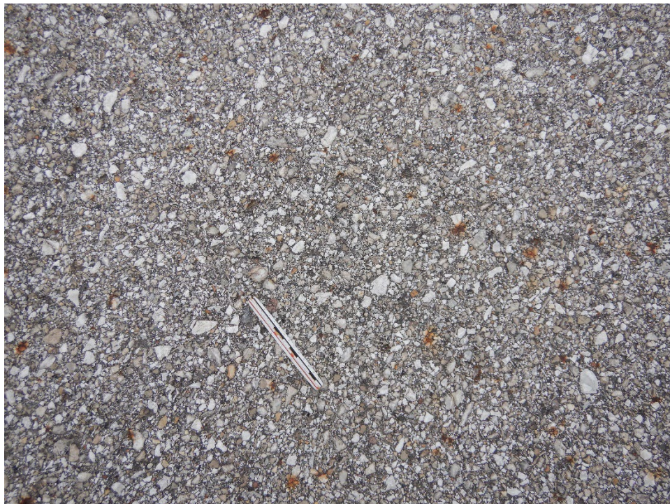
TH01FC-03. Weathering (Sample Unit No. 03).
