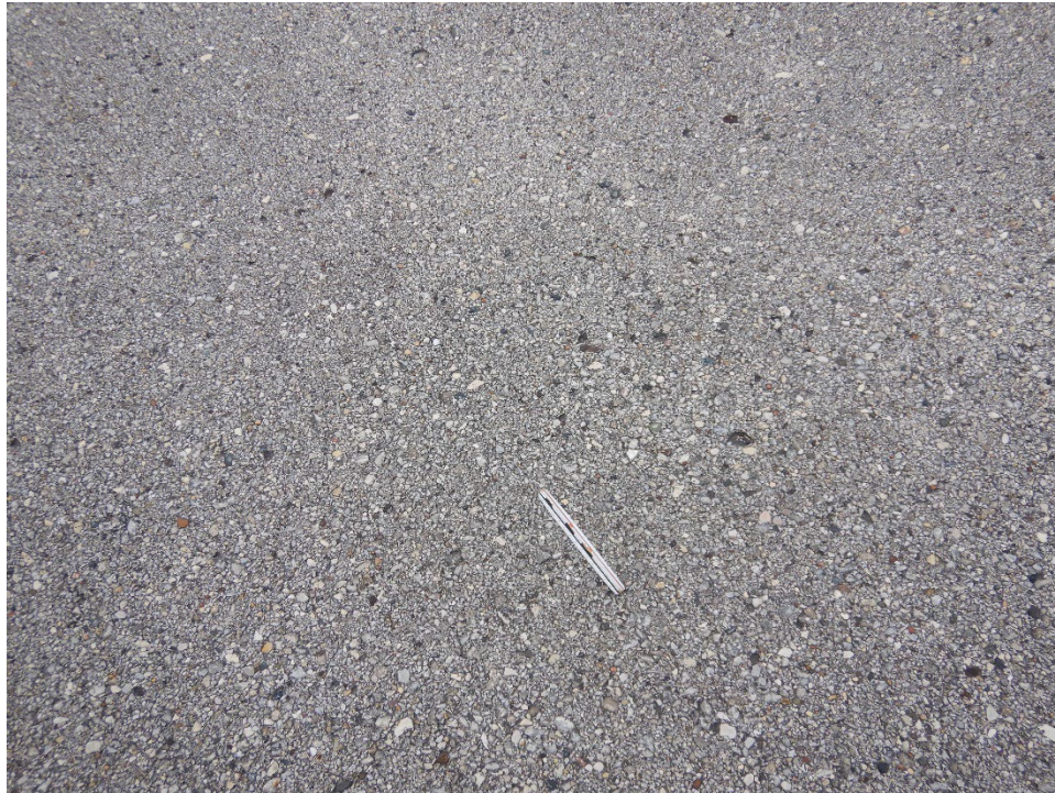
R15FC-01. Raveling (Sample Unit No. 05).
