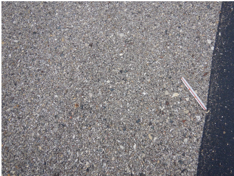
R09FC-01. Weathering (Sample Unit No. 01).
