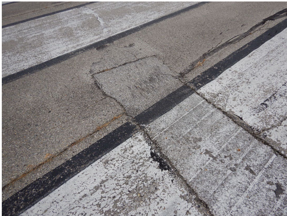
R15FC-02. Patching (Sample Unit No. 49).
