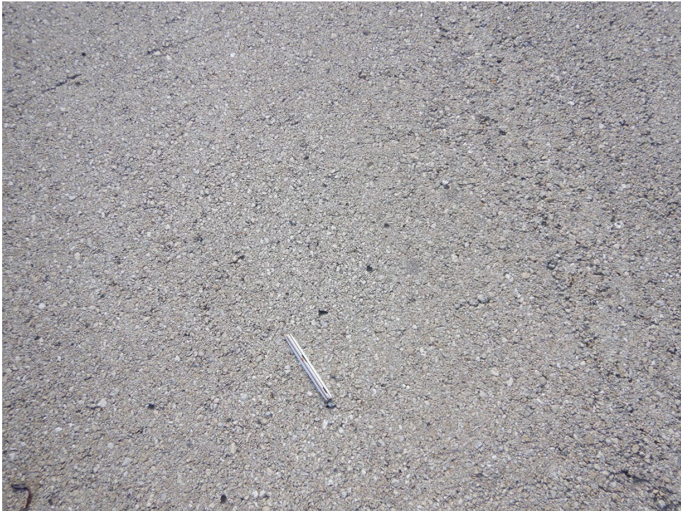
T02MT-01. Weathering (Sample Unit No. 05).
