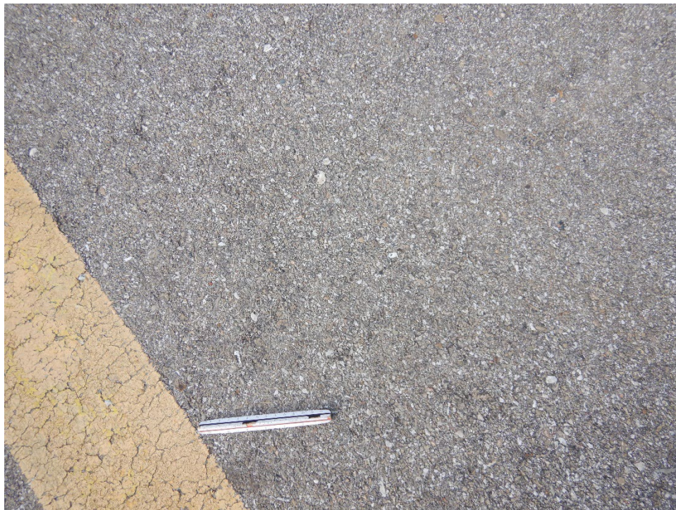
T01MT-01. Weathering (Sample Unit No. 02).
