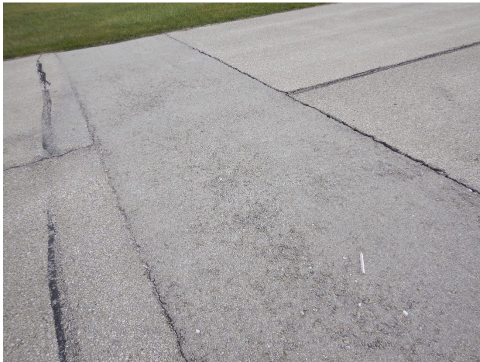
R18MT-02. Patching (Sample Unit No. 03).
