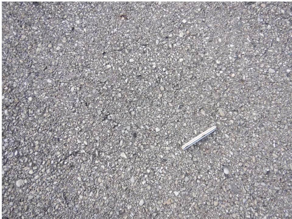
T03MT-02. Weathering (Sample Unit No. 01).
