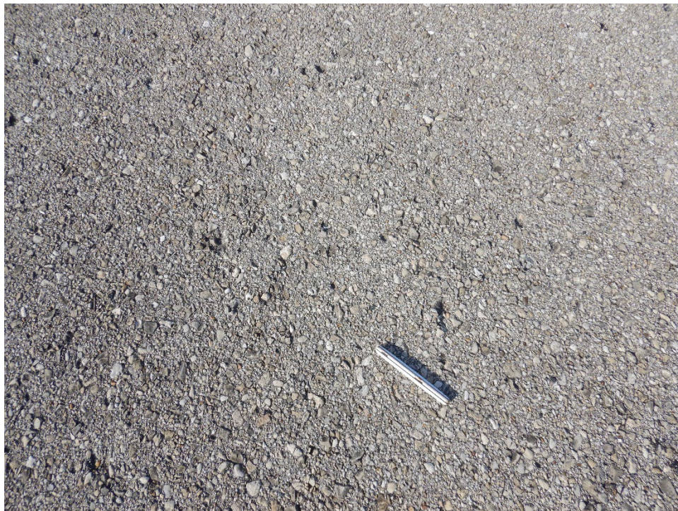
T04MT-01. Weathering (Sample Unit No. 11).
