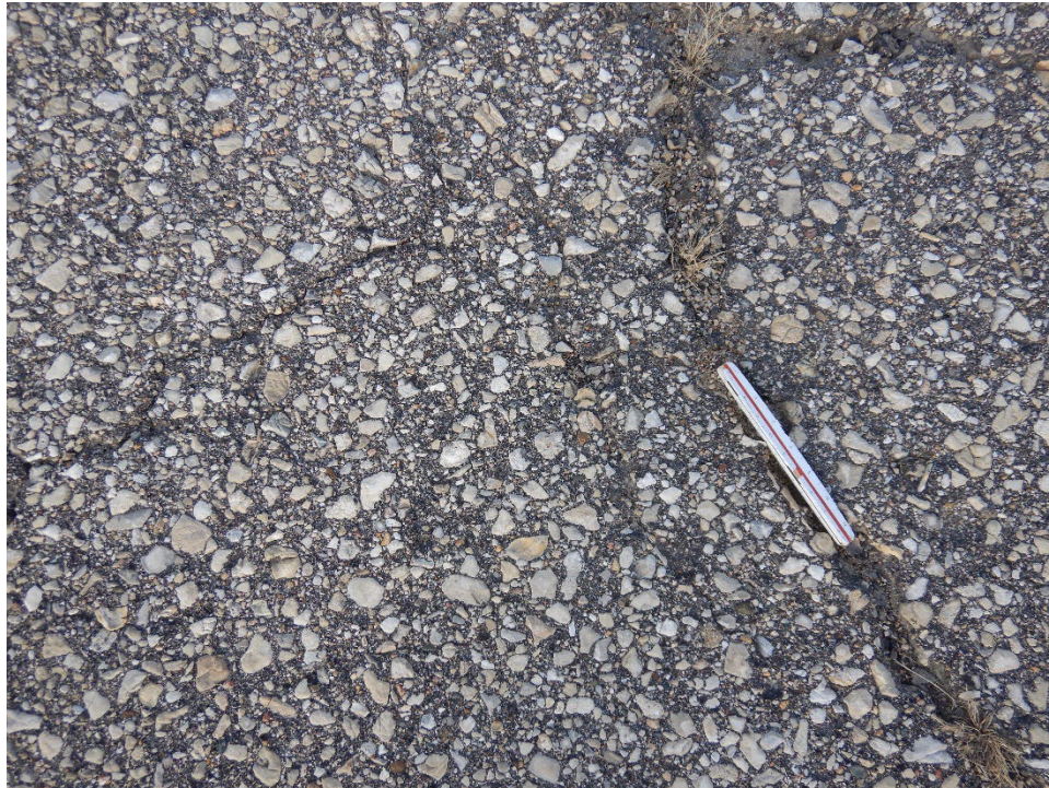
A02MT-02. Weathering (Sample Unit No. 02).
