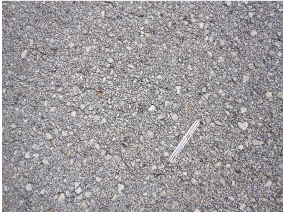
T03MT-01. Weathering (Sample Unit No. 03).
