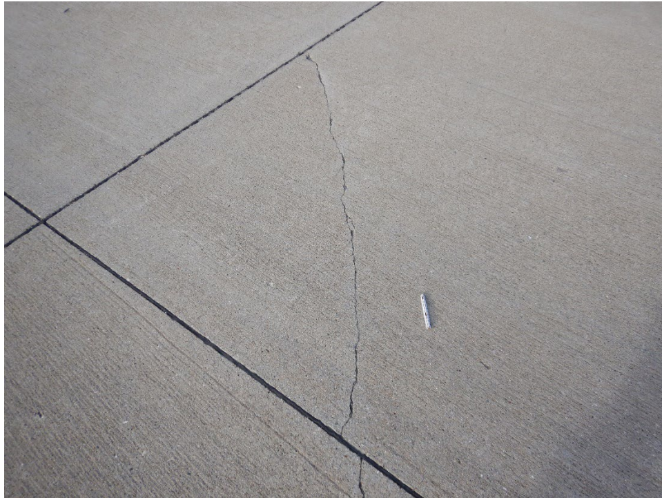
A02MT-01. Corner Break (Sample Unit No. 10).
