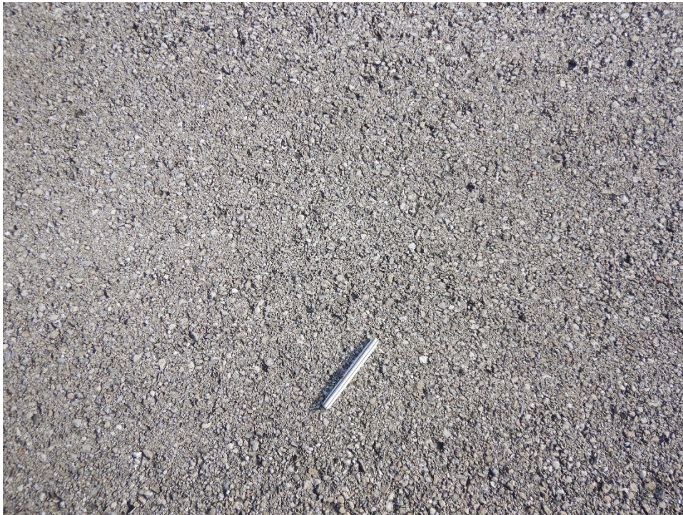
T02MT-02. Weathering (Sample Unit No. 01).
