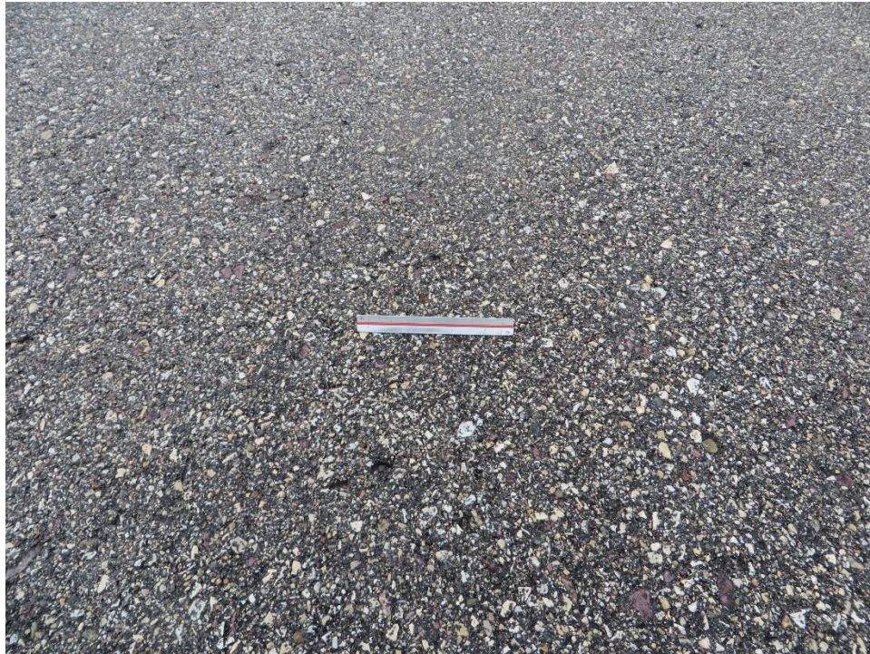
R09MD-02. Raveling (Sample Unit No. 03).
