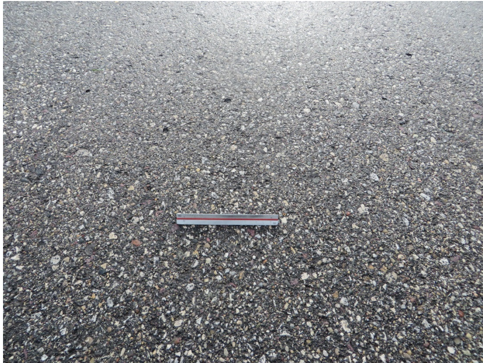
T01MD-01. Weathering (Sample Unit No. 02).
