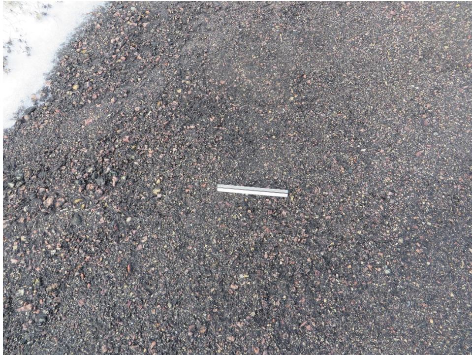
T01MD-02. Raveling (Sample Unit No. 01).
