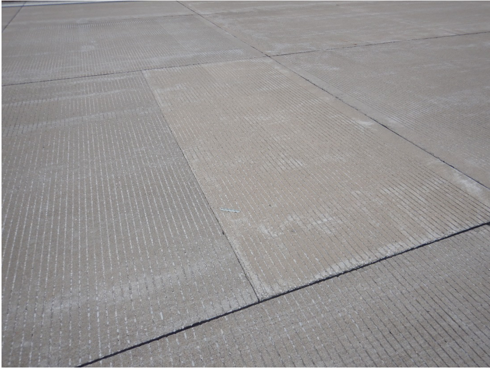
R06MU-01. Large Patching (Additional Sample Unit No. 063).
