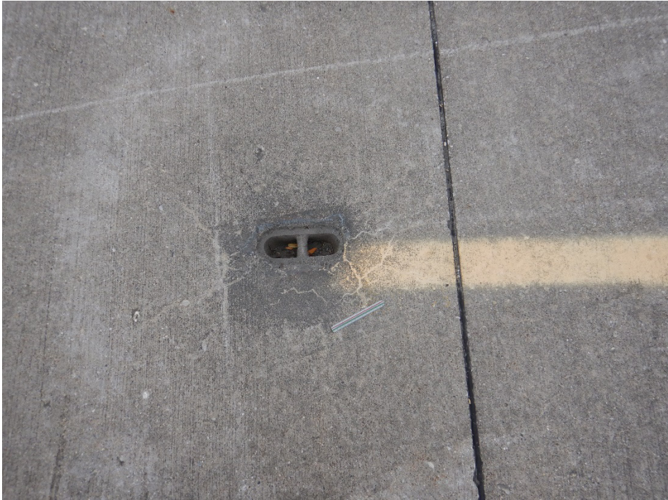
A01MU-01. ASR (Sample Unit No. 47).
