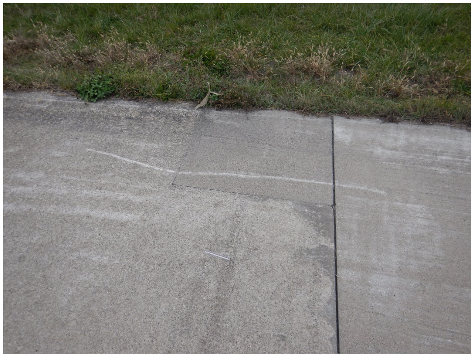
TB1MU-01. Large Patching (Sample Unit No. 04).
