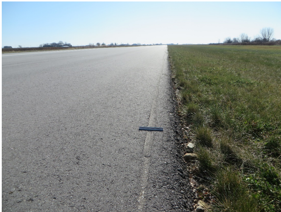
R17NH-01. Raveling (Sample Unit No. 06).
