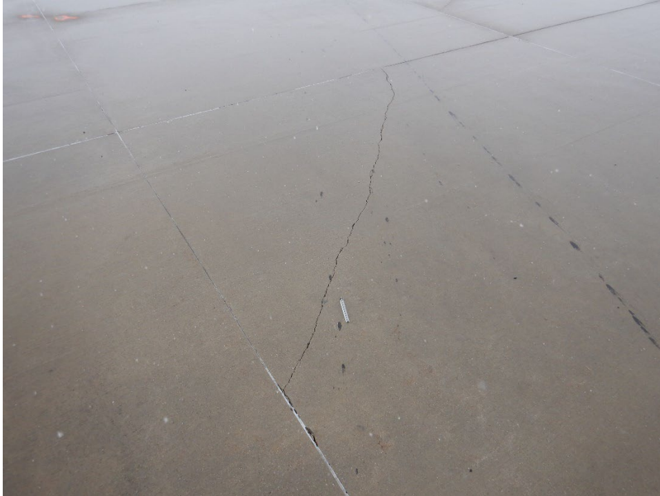
A01OT-08. Corner Break (Sample Unit No. 12).
