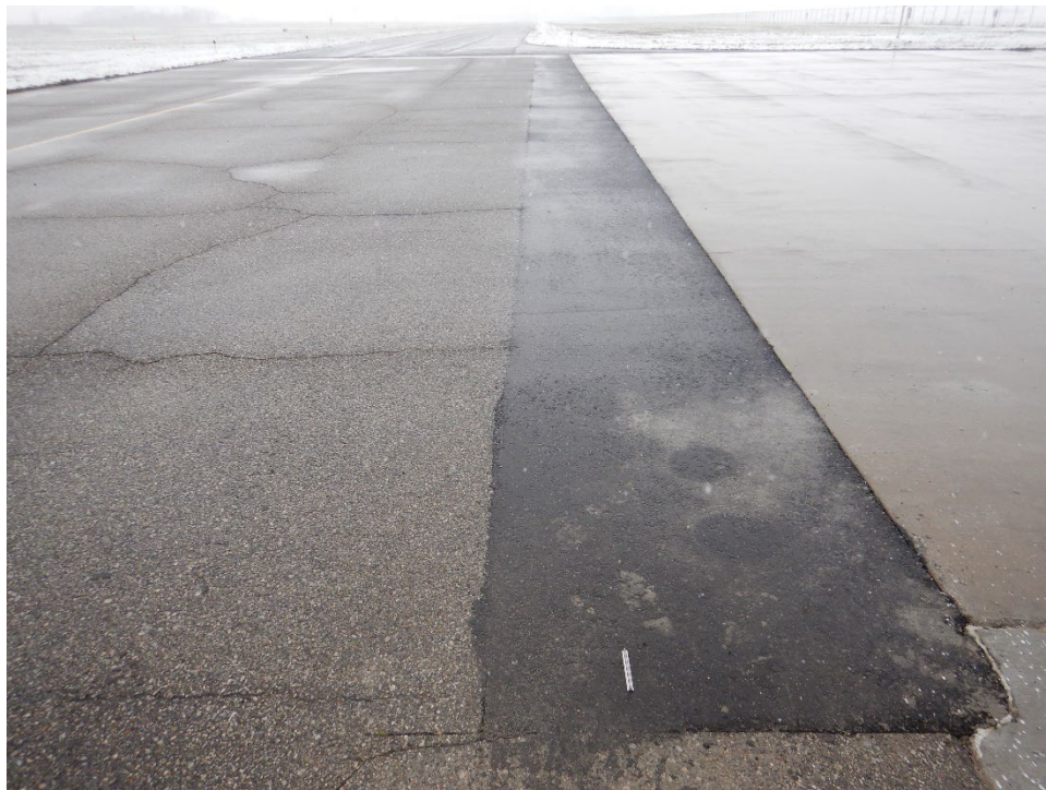
TBOT-06. Patching (Additional Sample Unit No. 01).
