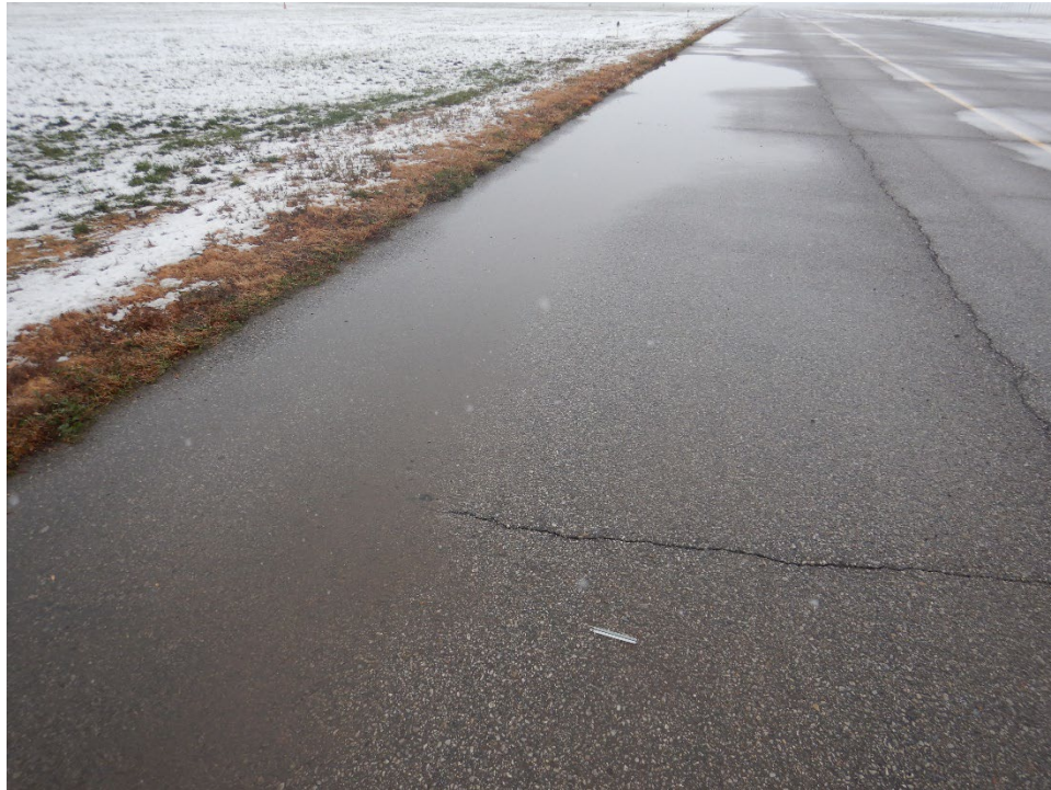
TBOT-06. Depression (Sample Unit No. 02).
