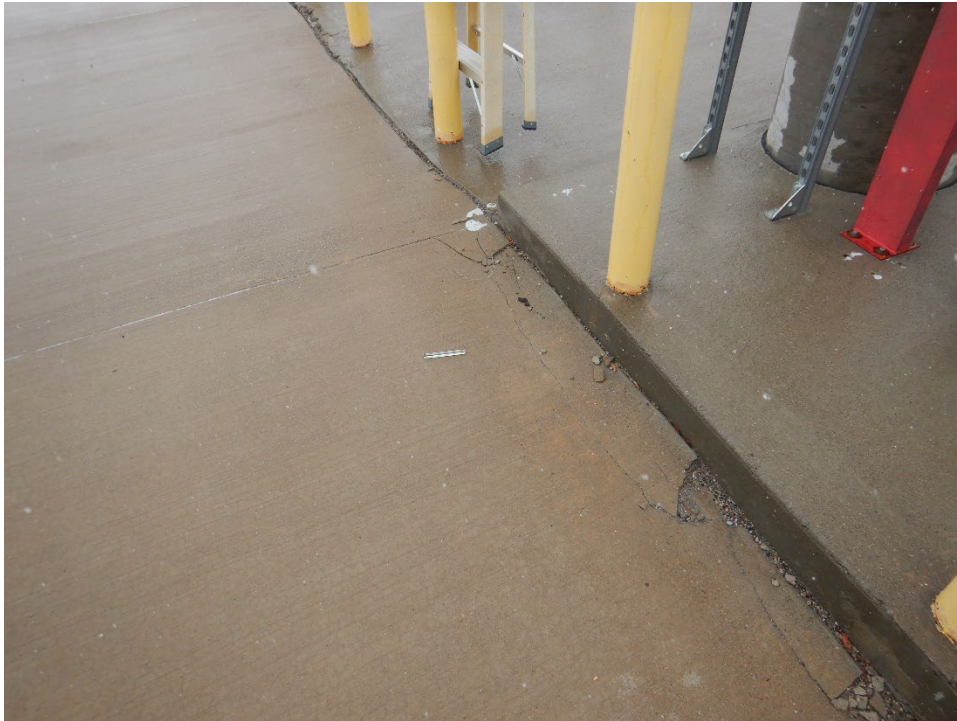
A01OT-06. Blow-Up (Sample Unit No. 12).
