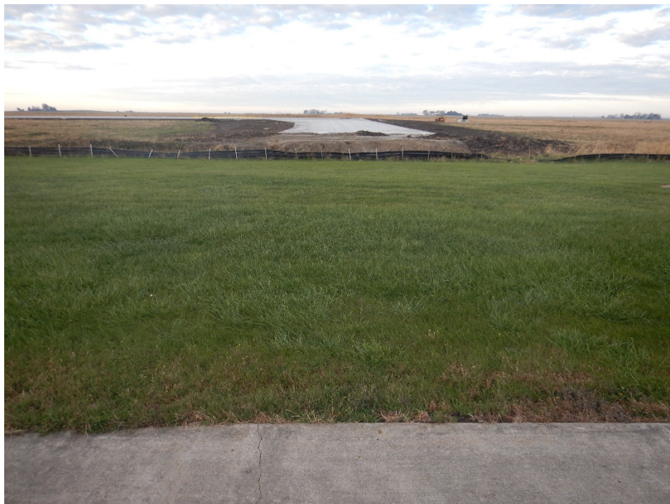
TA1PR-01. Overview (Under Construction).
