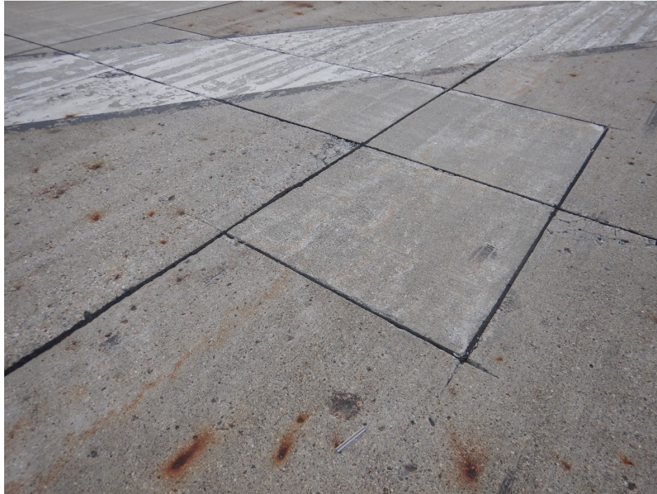
T02PR-02. Large Patching (Sample Unit No. 20).
