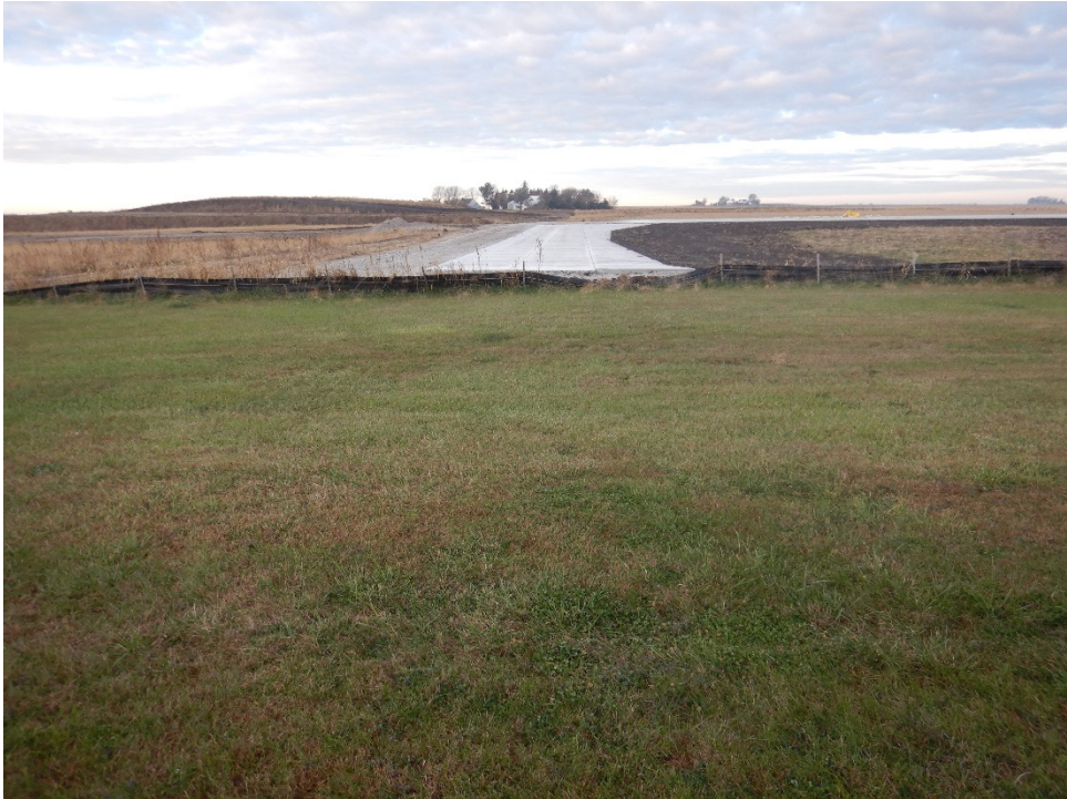
TA3PR-01. Overview (Under Construction).
