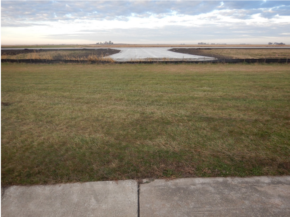
TA2PR-01. Overview (Under Construction).
