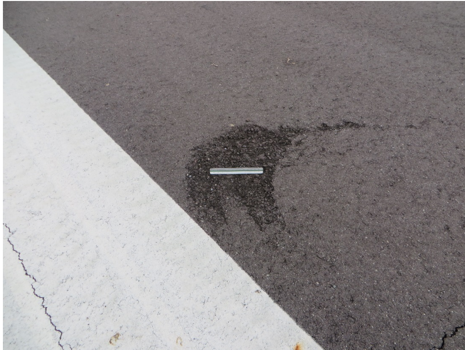
R16RR-02. Raveling (Sample Unit No. 07).
