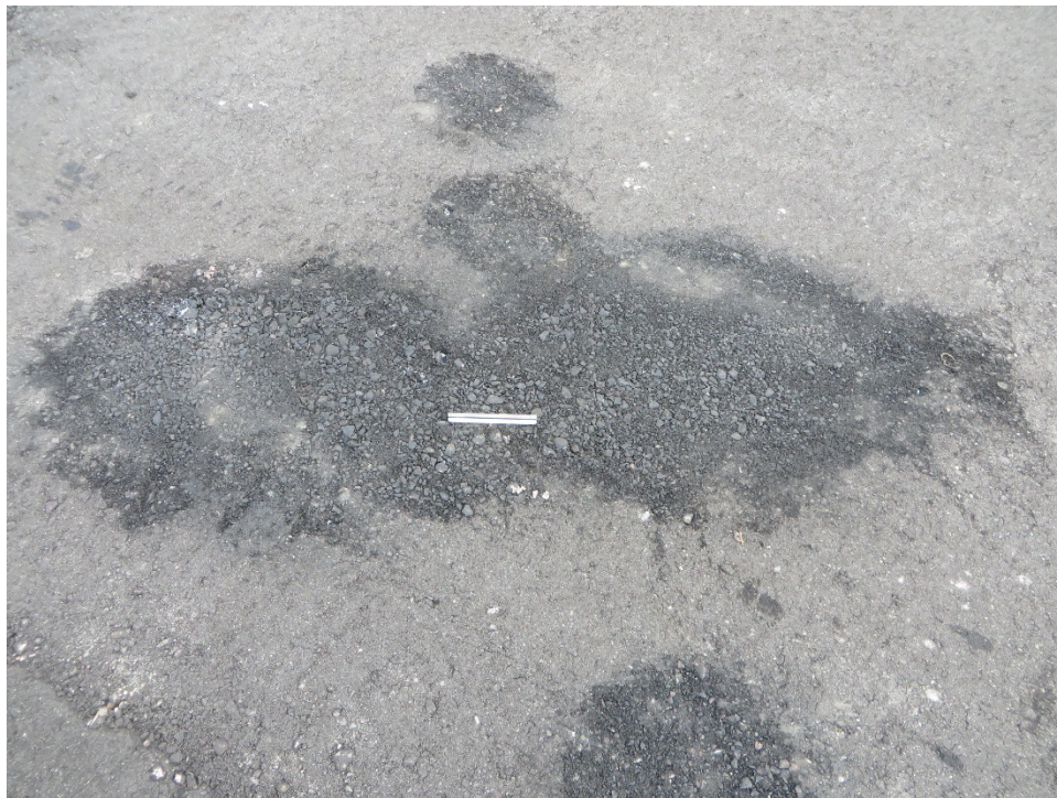
R16RR-01. Raveling (Sample Unit No. 01).
