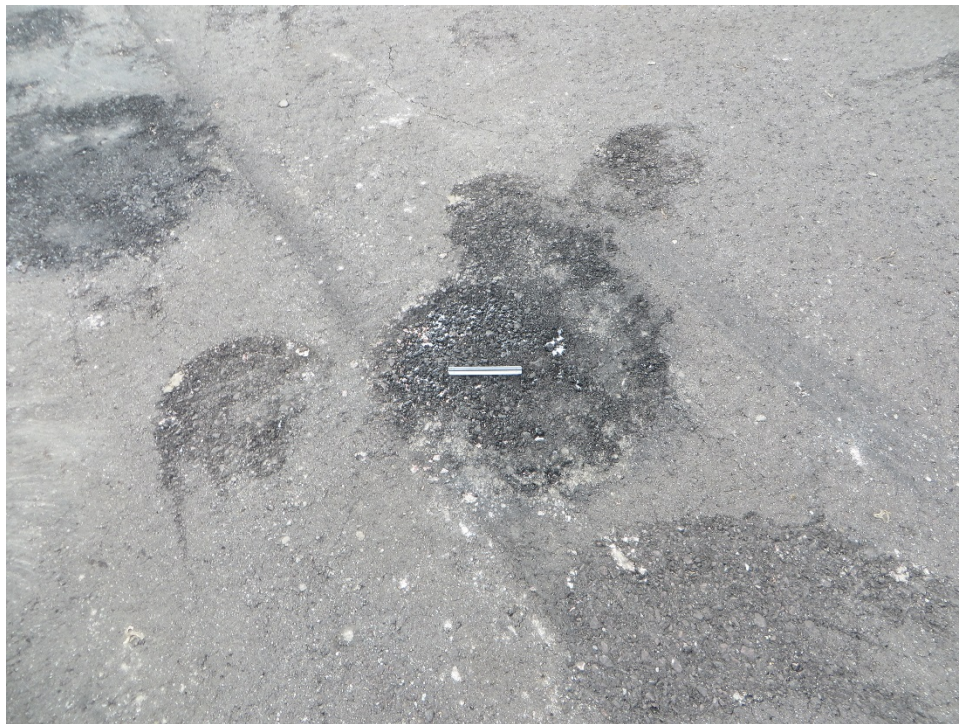
R16RR-03. Raveling (Sample Unit No. 03).
