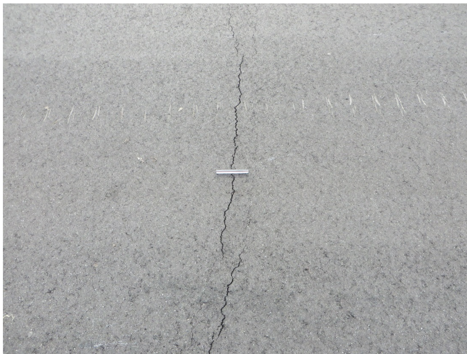
T01RR-01. L&T Cracking (Sample Unit No. 01).
