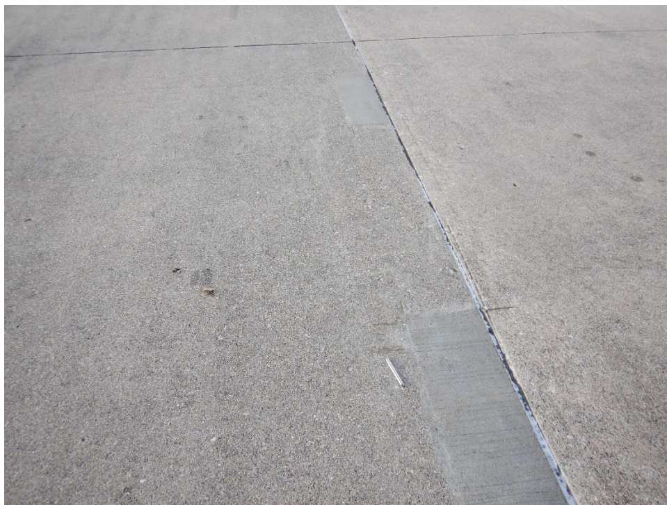
R13SL-01. Small Patching (Sample Unit No. 07).
