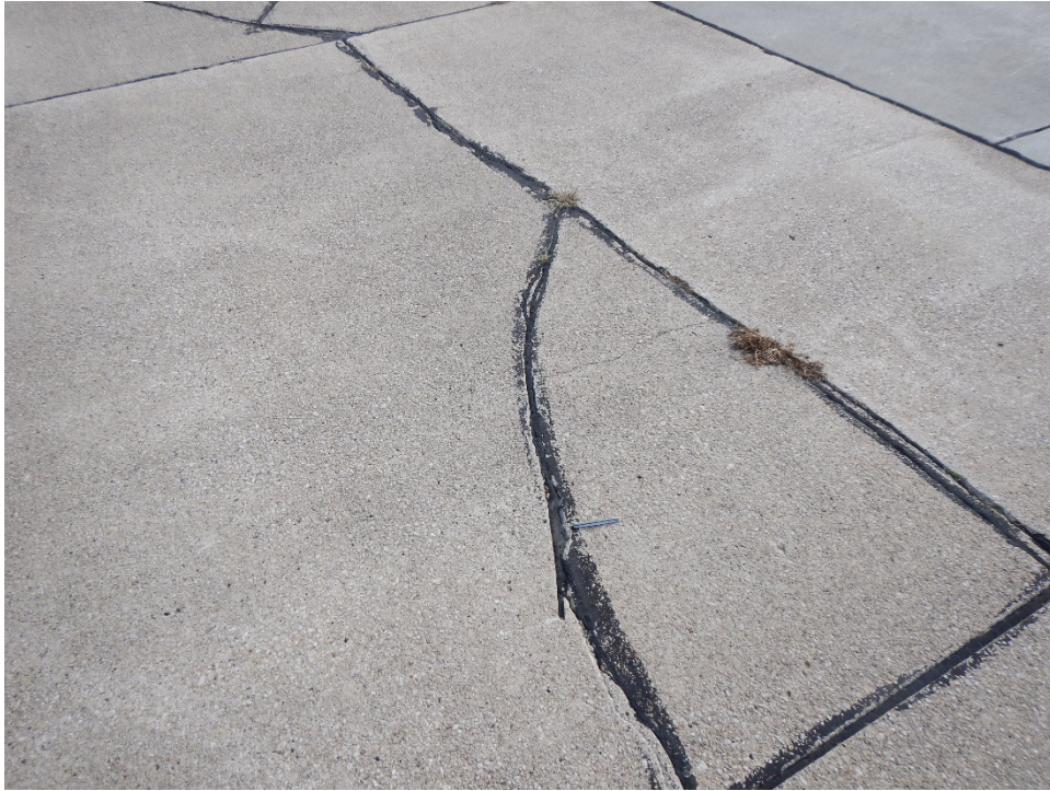
A01TI-01. Shattered Slab (Sample Unit No. 02).
