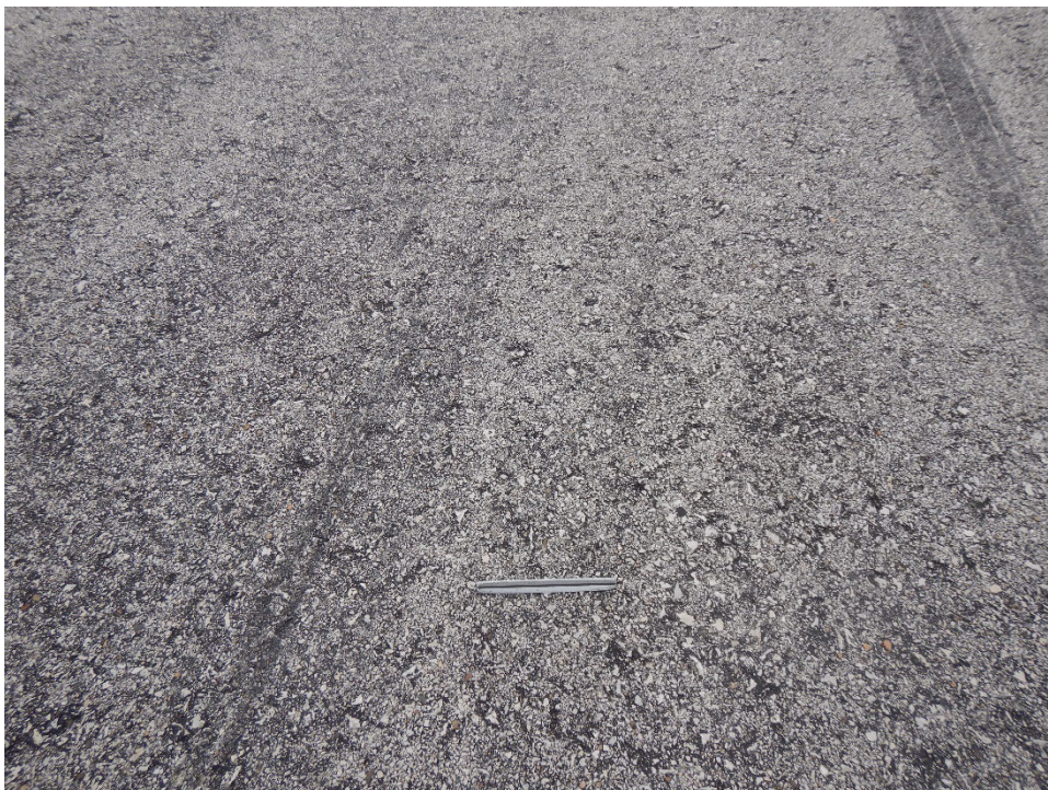
R16VI-03. Weathering (Sample Unit No. 01).
