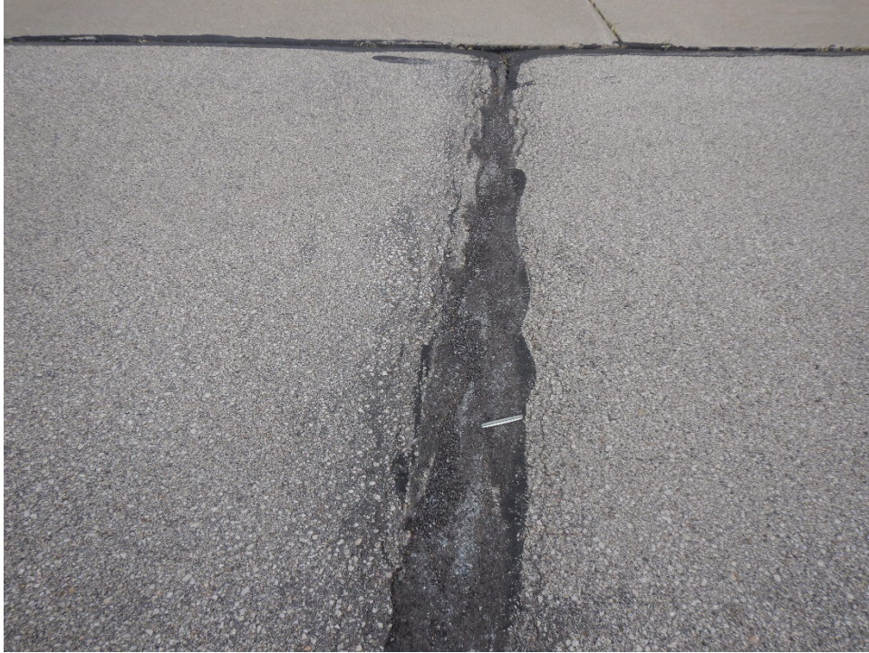
A01VI-05. Patching (Sample Unit No. 01).
