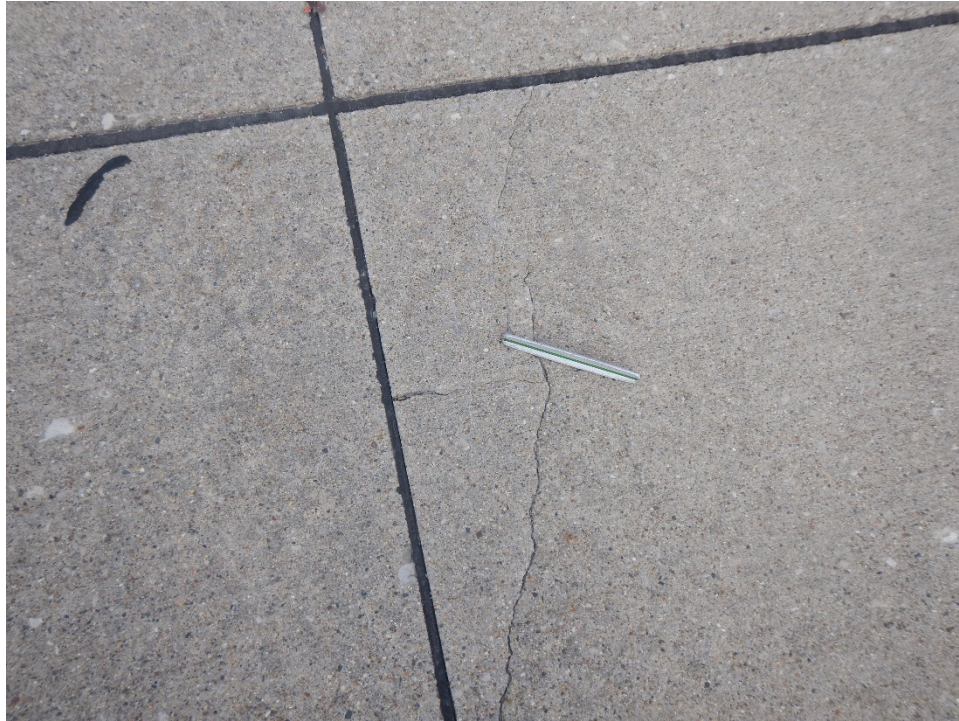
A01VI-04. ASR (Sample Unit No. 14).
