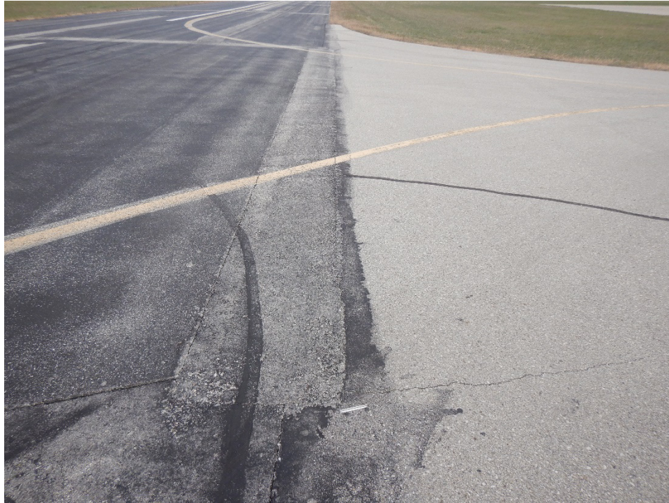
T01VI-01. Patching (Sample Unit No. 01).
