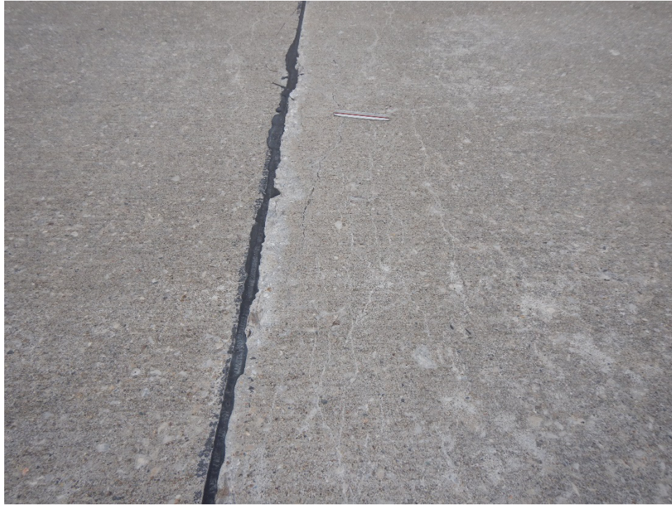
R09VI-01. ASR (Sample Unit No. 012).
