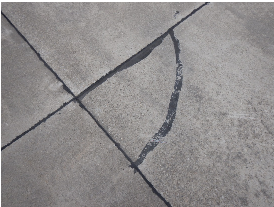
TH01VI-04. Corner Break (Sample Unit No. 01).
