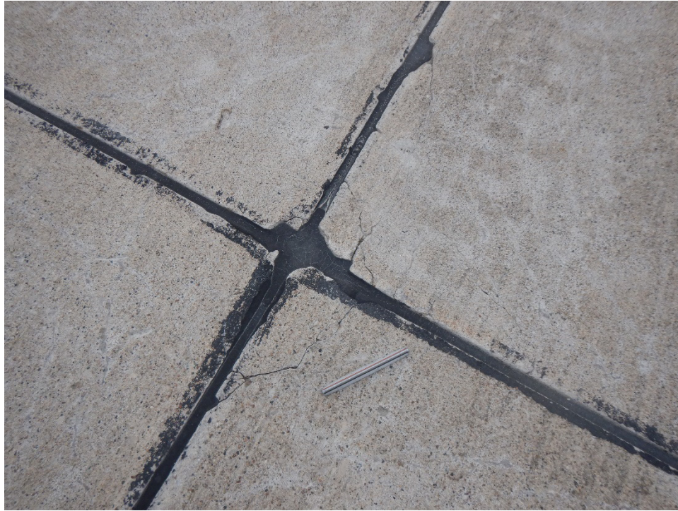
T02VI-01. ASR (Sample Unit No. 03).
