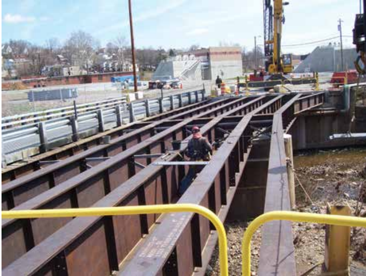
Coatesville steel mill Duracorr®/A1010 bridge.
