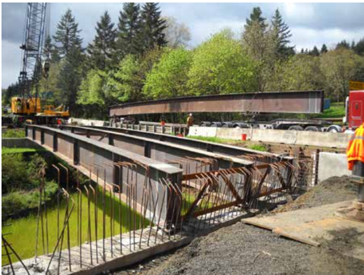
Oregon DOT Dodge Creek A1010 Bridge.
