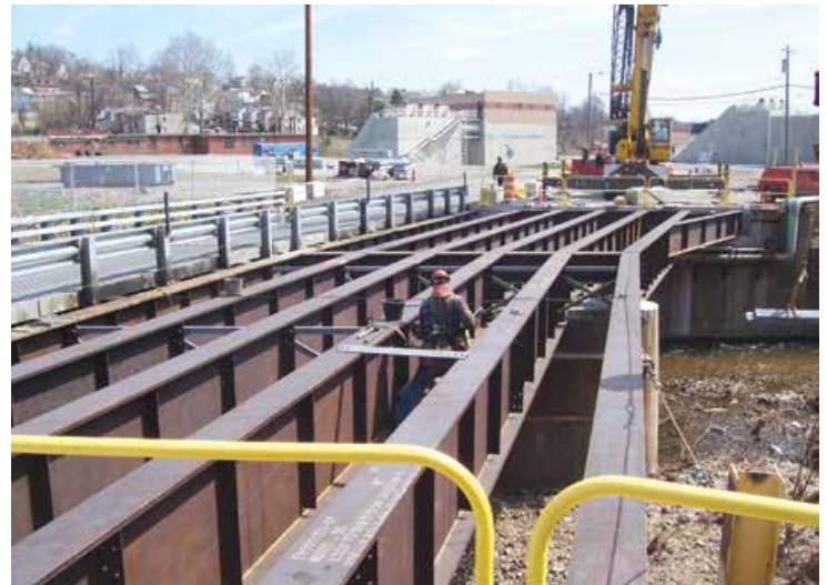
Bridge fabricated from A1010/Duracorr, Coatesville, PA
