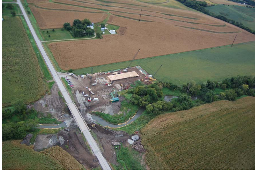
Figure 14 – Temporary Bridge Production Site.
