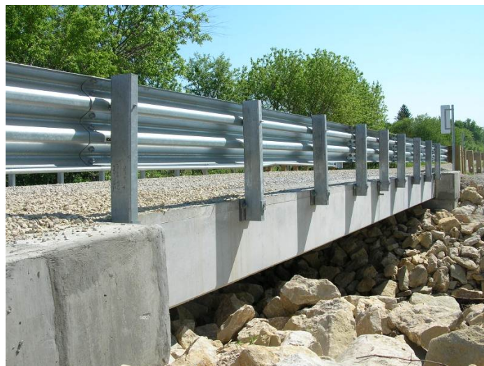
Figure 8 – Madison Completed Bridge
