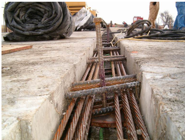
Figure 5 – Post-Tensioning Channel
