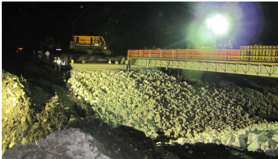
Figure 23 – Massena Bridge Slide 30% Complete
