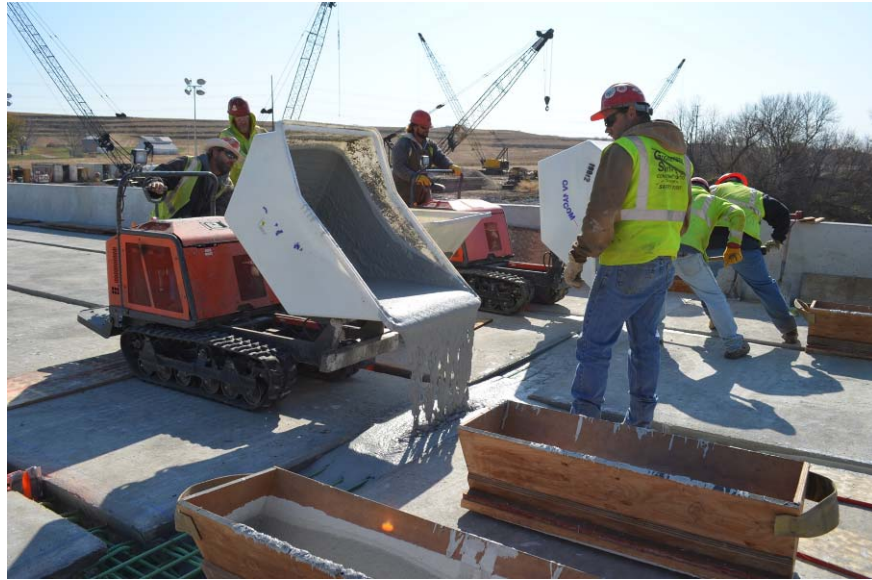
Figure 17 – Placement of UHPC
