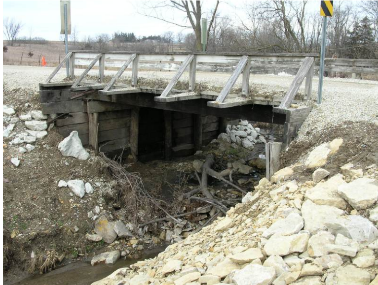
Figure 6 – Madison Timber Bridge
