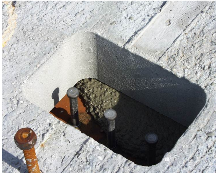
Figure 12 – Shear Stud Pocket
