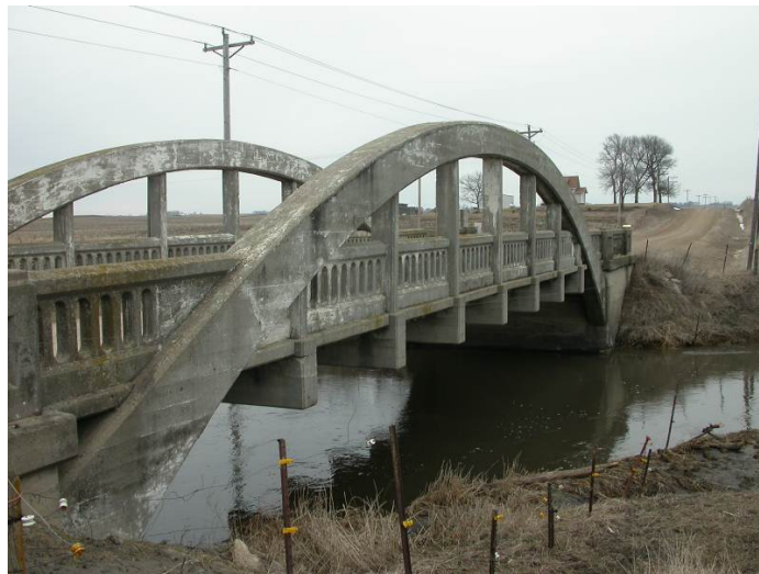
Figure 1 – Marsh Arch Bridge
