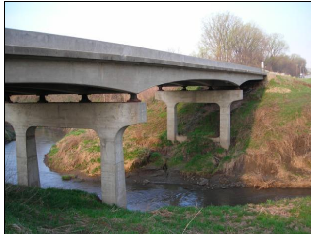
Figure 13 – Original US 6 over Keg Creek Bridge
