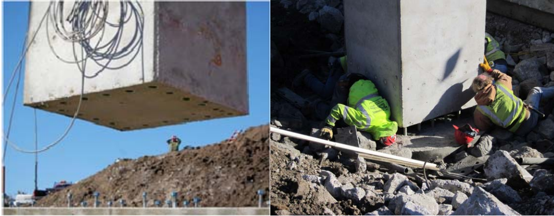
Figure 15 – Precast Column Installation (Grouted Splice Couplers)
