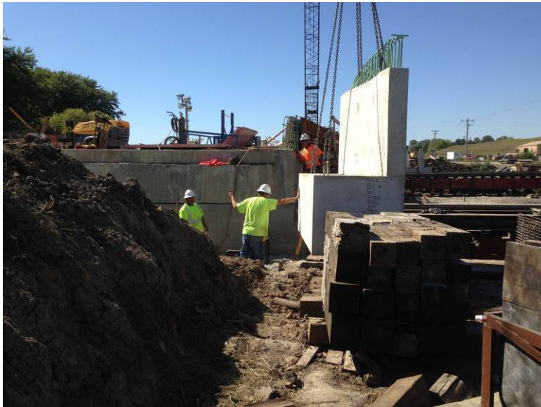
Figure 24 – Precast Wingwall Installation
