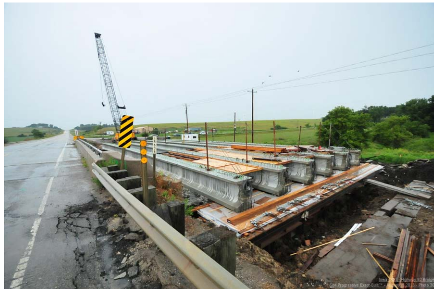
Figure 20 – PPC Beams on Falsework
