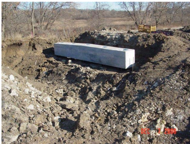
Figure 7 – Precast Abutment Footing
