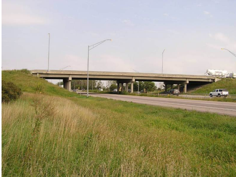
Figure 9 – Original 24 th Street over I-29/I-80 Bridge
