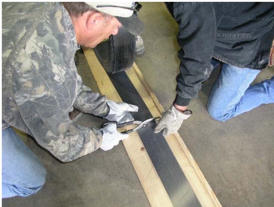
Figure 16. Cutting the CFRP plates.
