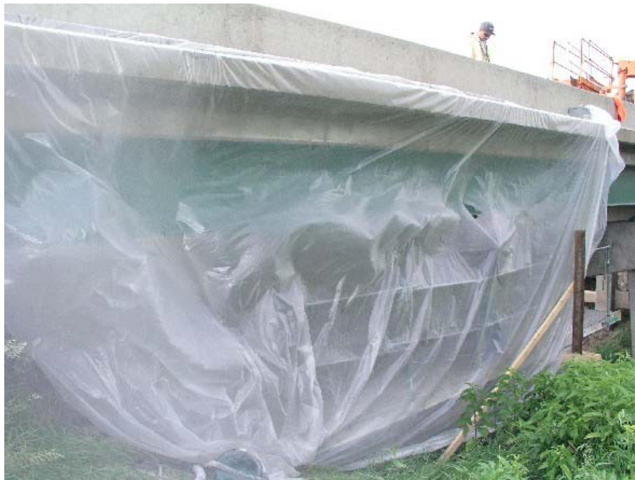
Figure 10. Confinement of work area during sandblasting.
