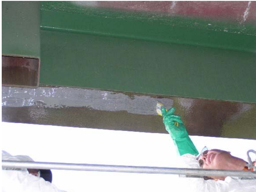
(b) Application of structural epoxy to bottom girder flange
