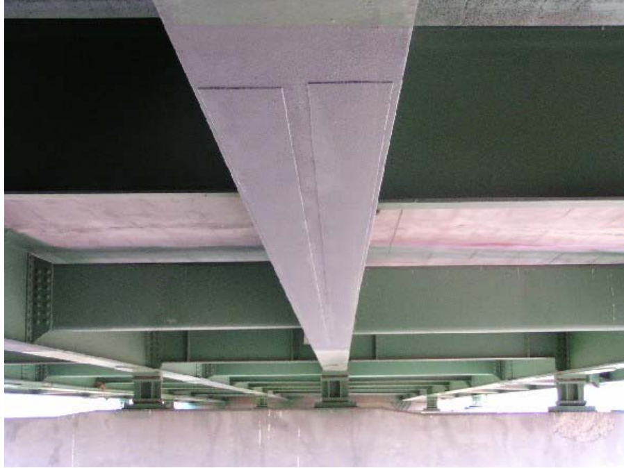
(b) Girder 3 in the west end span
