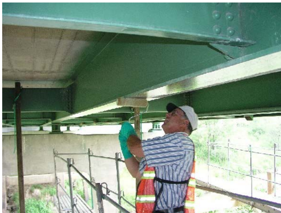
Figure 14. Applying FRS 1000 Primer to bottom girder flange.
