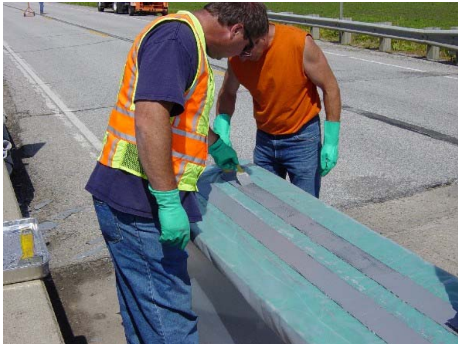
(a) Application of structural epoxy to CFRP plate.
