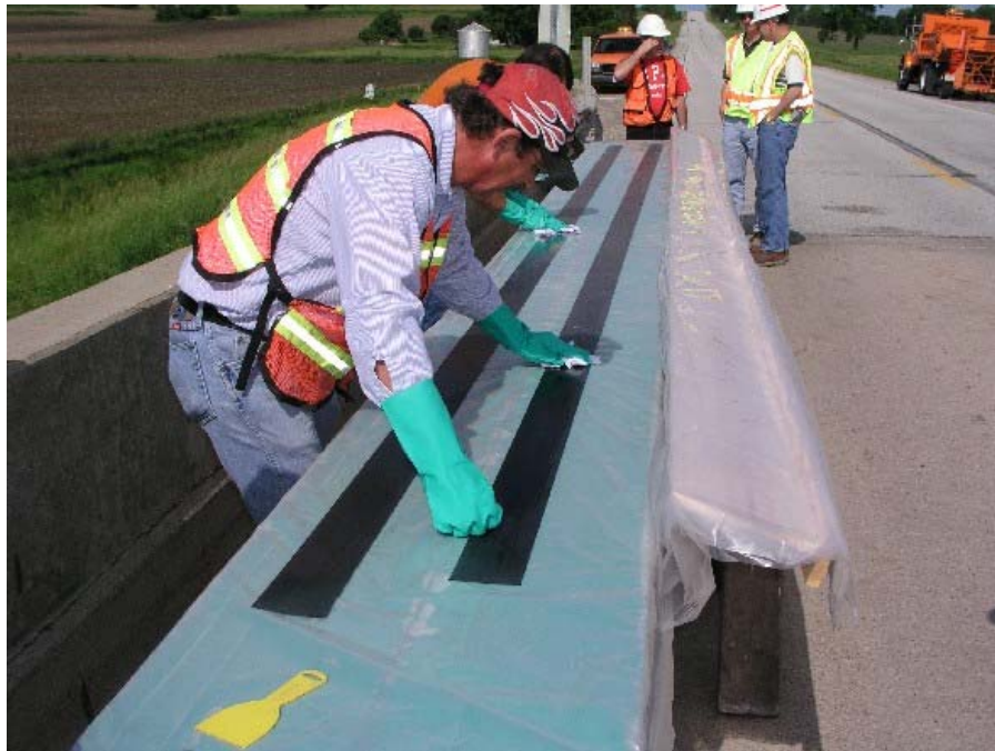
Figure 13. Cleaning the CFRP plate bonding surface.
