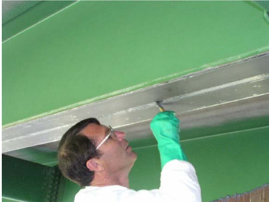
Figure 20. Removal of excess epoxy.
