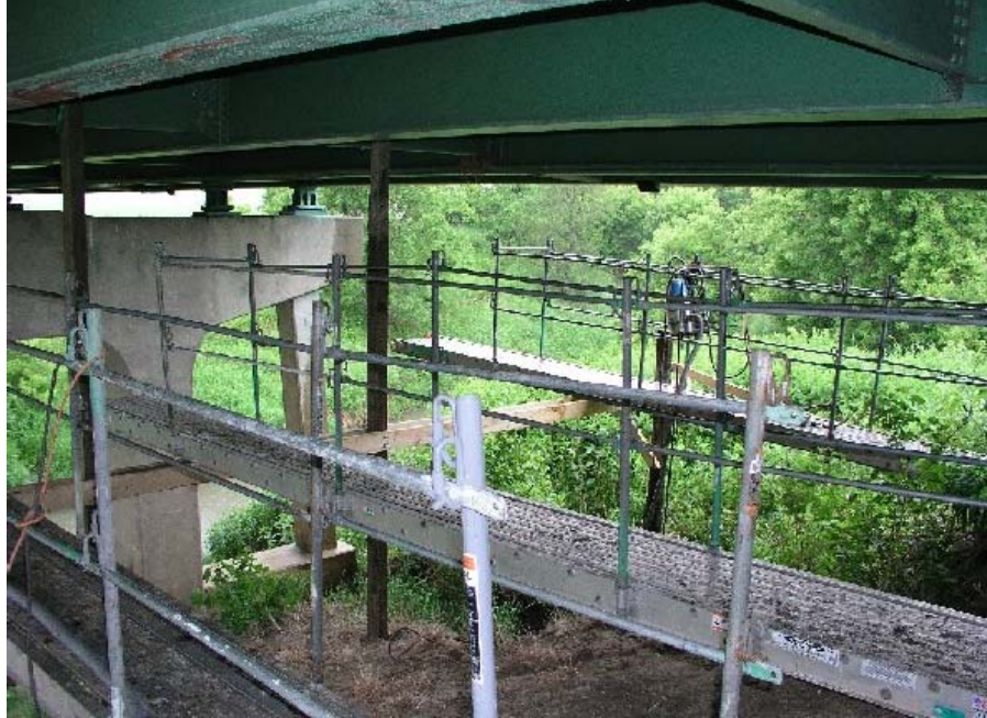
Figure 9. Temporary work scaffolding.
