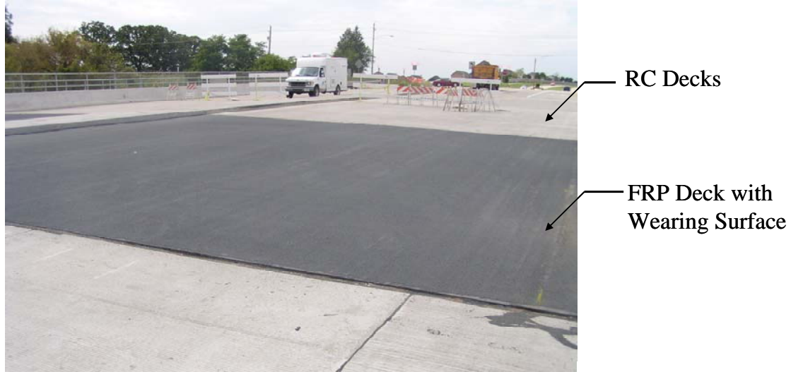
Figure 14. FRP Deck – May 2003
