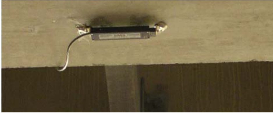
Figure 25. Close Up View of an Installed Peak Strain Sensor
