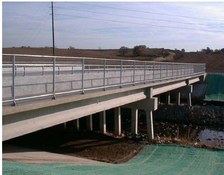
Figure 3. Bettendorf Bridge – Looking East
