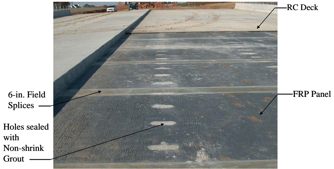
Figure 12. FRP Deck - Top Surface
