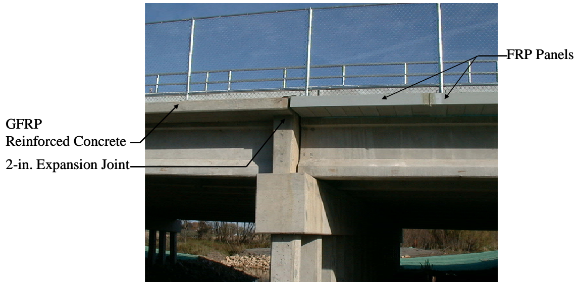
Figure 7. Expansion Joint Detail
