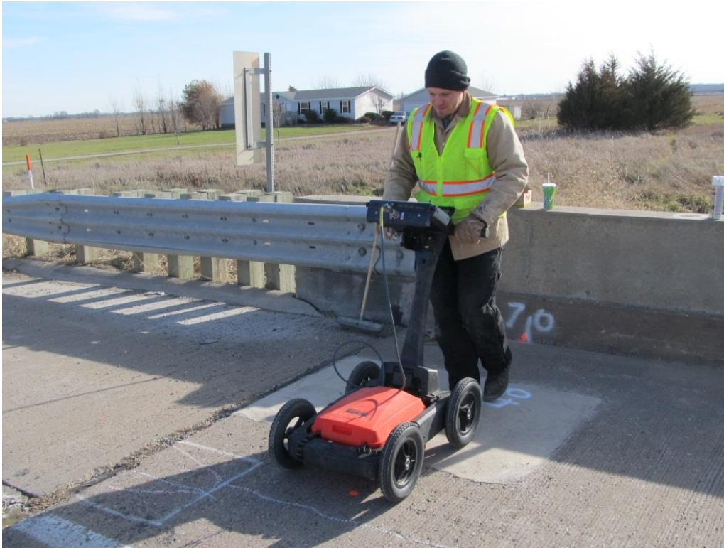
Figure 2.1. Measuring reinforcing cover depth with GPR.
