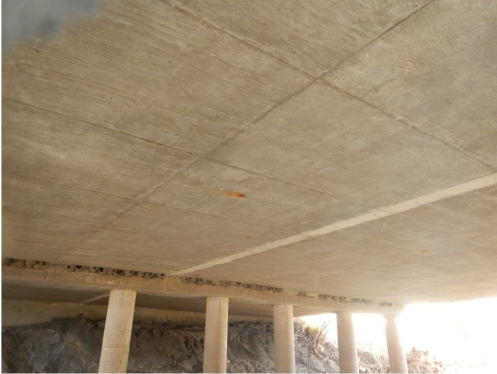
Figure 3.7. Deck underside center span.
