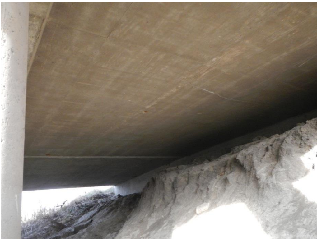
Figure 3.6. Deck underside east span.
