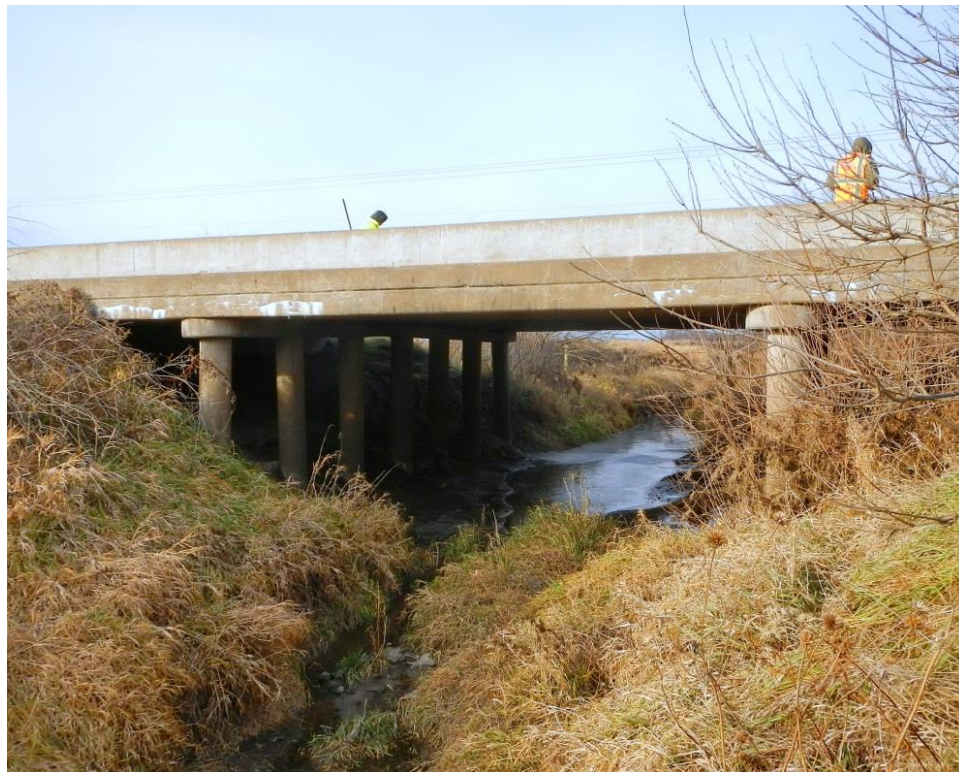
Figure 1.2. South elevation of subject bridge.
