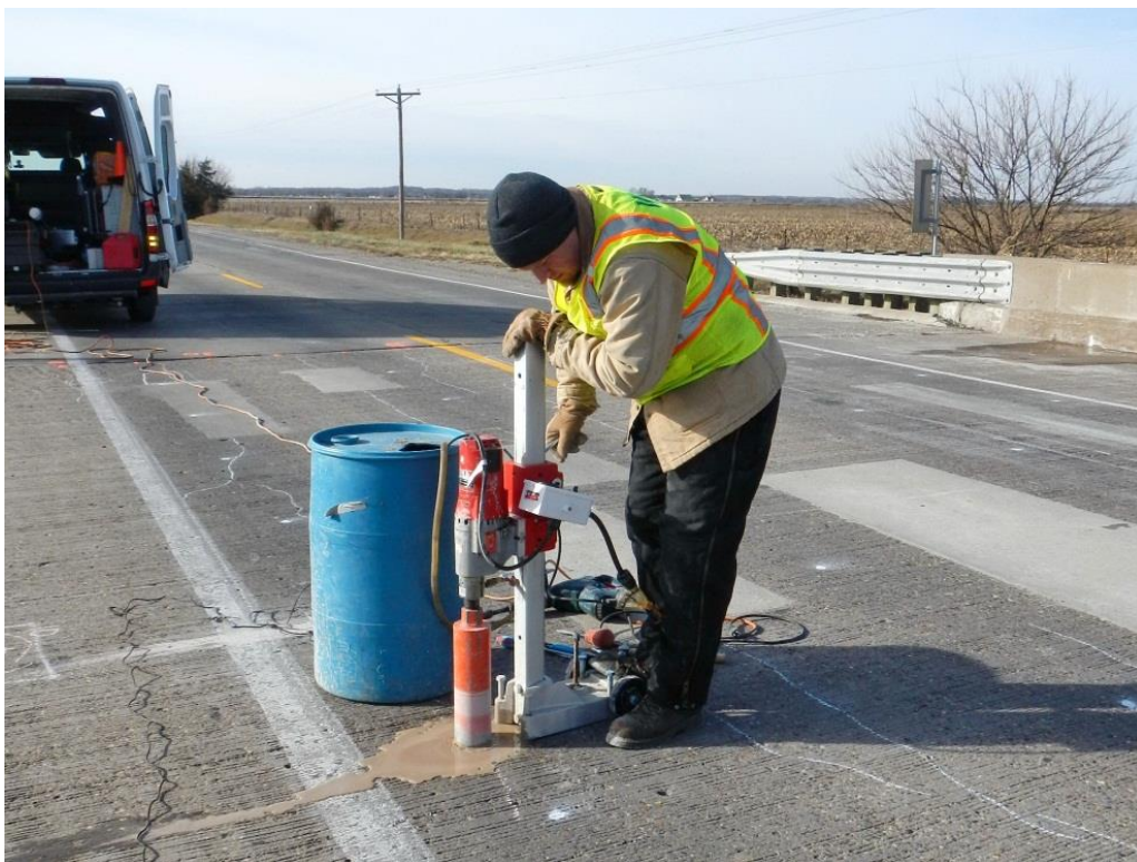
Figure 2.2. Drilling a core sample from the deck.
