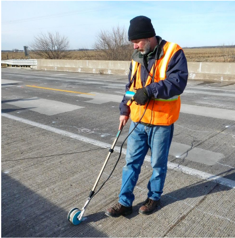
Figure 2.3. Measuring half-cell potentials with single rolling wheel equipment (Proceq Canin+).
