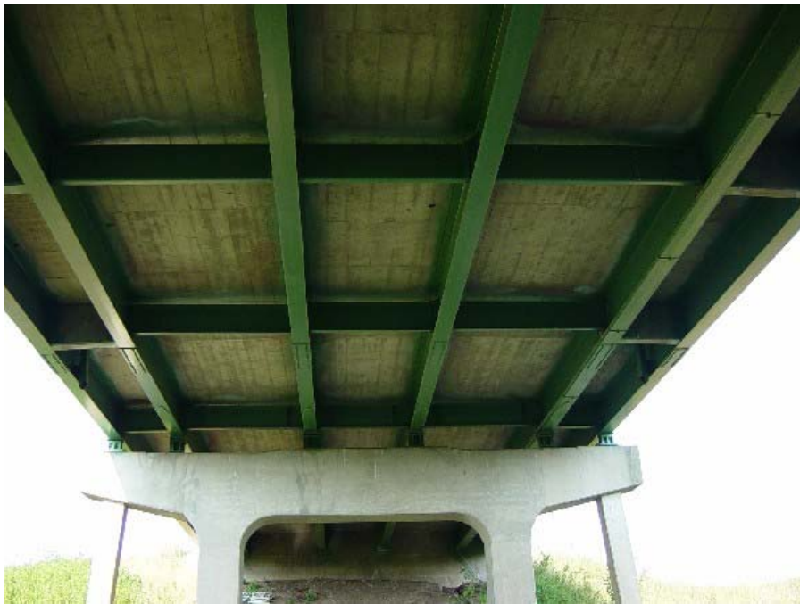
b. Bottom view – field bridge
