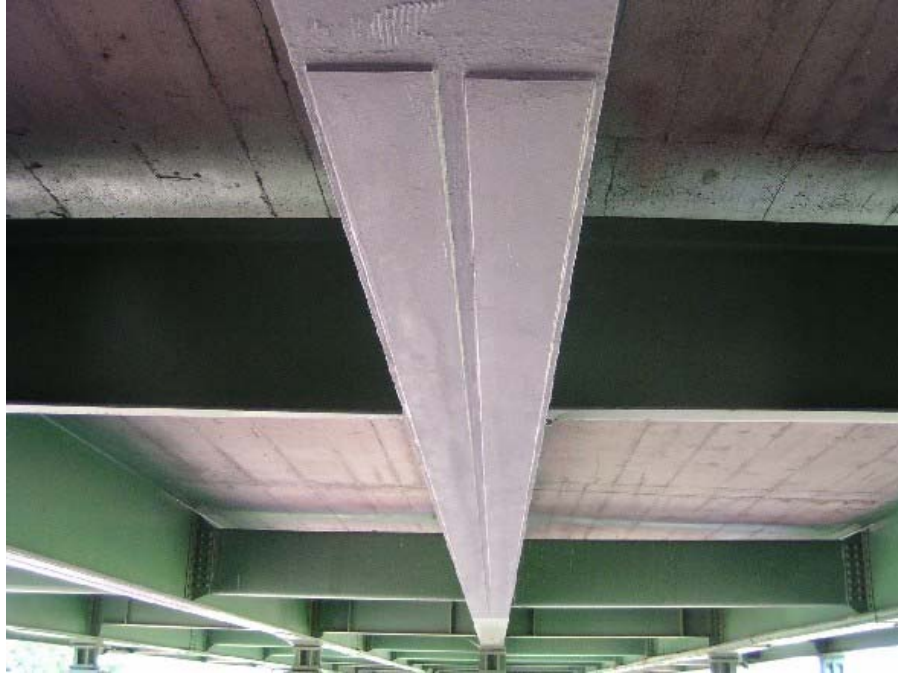
a. Beam 4 in the east end span
