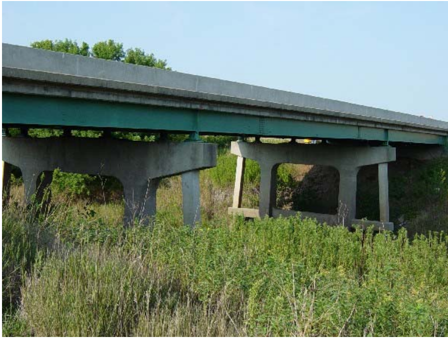
a. Side view – field bridge
