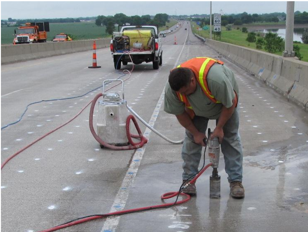
Figure 2.3. Removal of concrete core sample.
