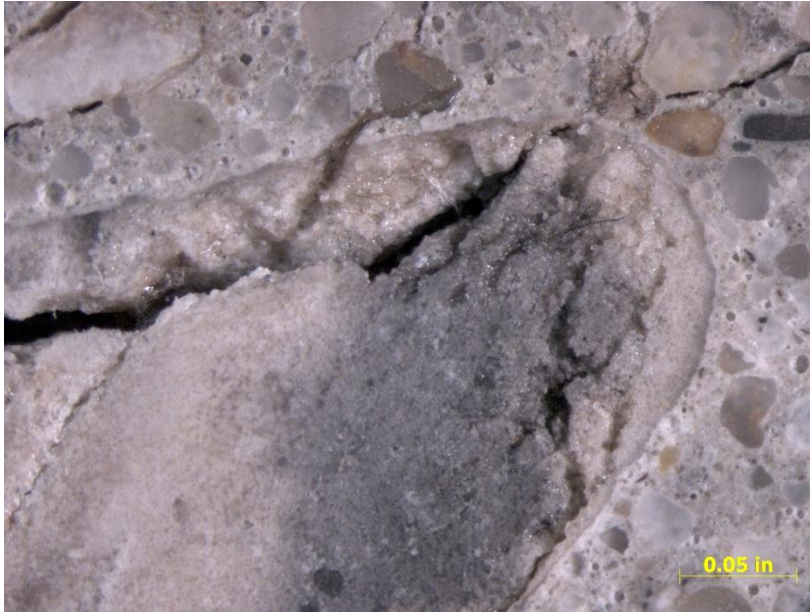
Figure 12. Core 42 base concrete; reactive sandstone particle, partially consumed in ASR; cracks extending into the surrounding cement paste.
