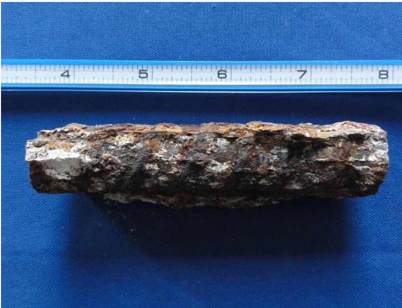
Figure 9. Core 42: corroded rebar taken out of base concrete at one of the cracks.
