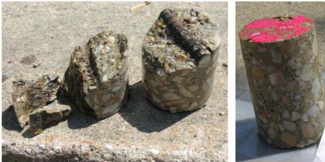
Figure 73. Cores #3 (left) and 4 (right), selected as “deteriorated” and “control” (sound) specimens for Deck O2.
