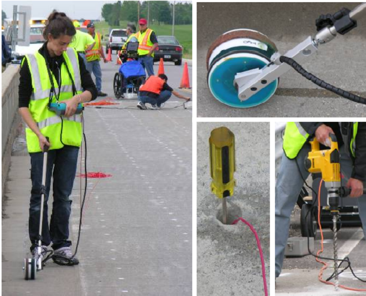
Figure 51. Half-cell (HC) potential measurement on deck; showing probe detail, drilled hole and wire lead connected electrically to the upper rebar mat.
