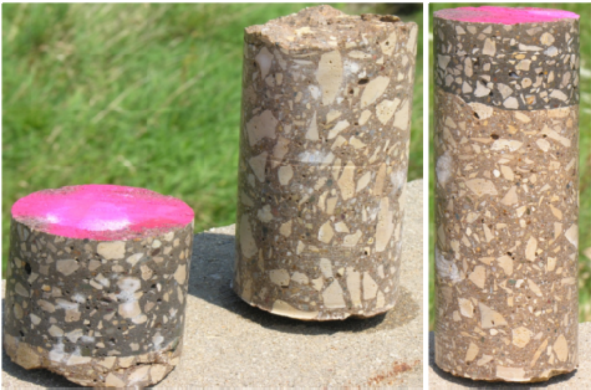
Figure 121. Cores 1 & 2 (left and right), graded “serious” (delaminated) and “good” (intact) using IE.
