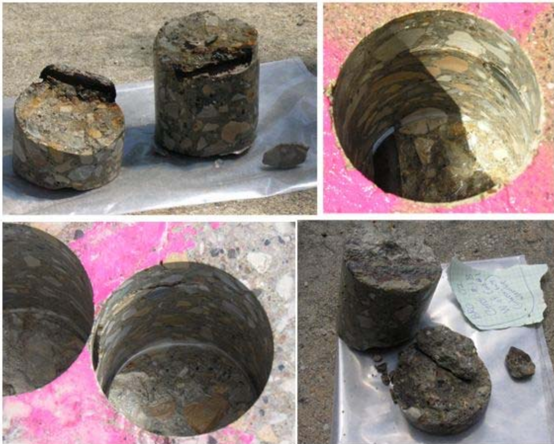
Figure 72. Core #2 and its hole (top) shown with Core #1b hole and its extracted core (bottom), immediately adjacent to the hole for Core #1a (half shown in photo).
