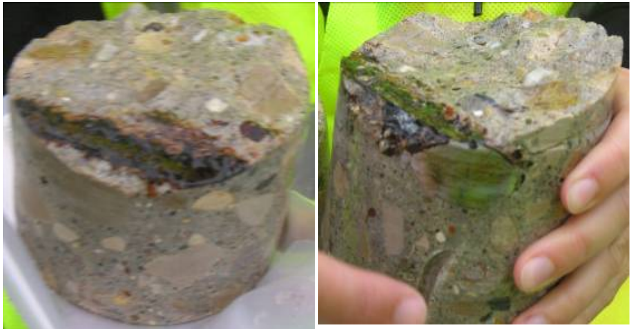
Figure 91. Top of Core #4 (inverted, left) reveals corrosion products above delamination; core bottom (right) with corrosion products on top and sides of rebar.
