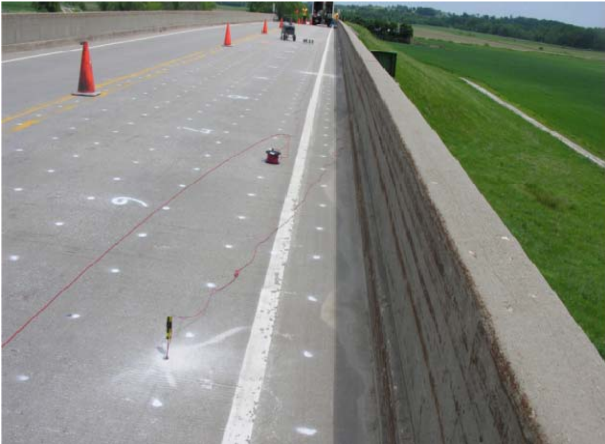
Figure 129. Grid on EBL, showing HC lead connected to rebar through small hole (foreground).
