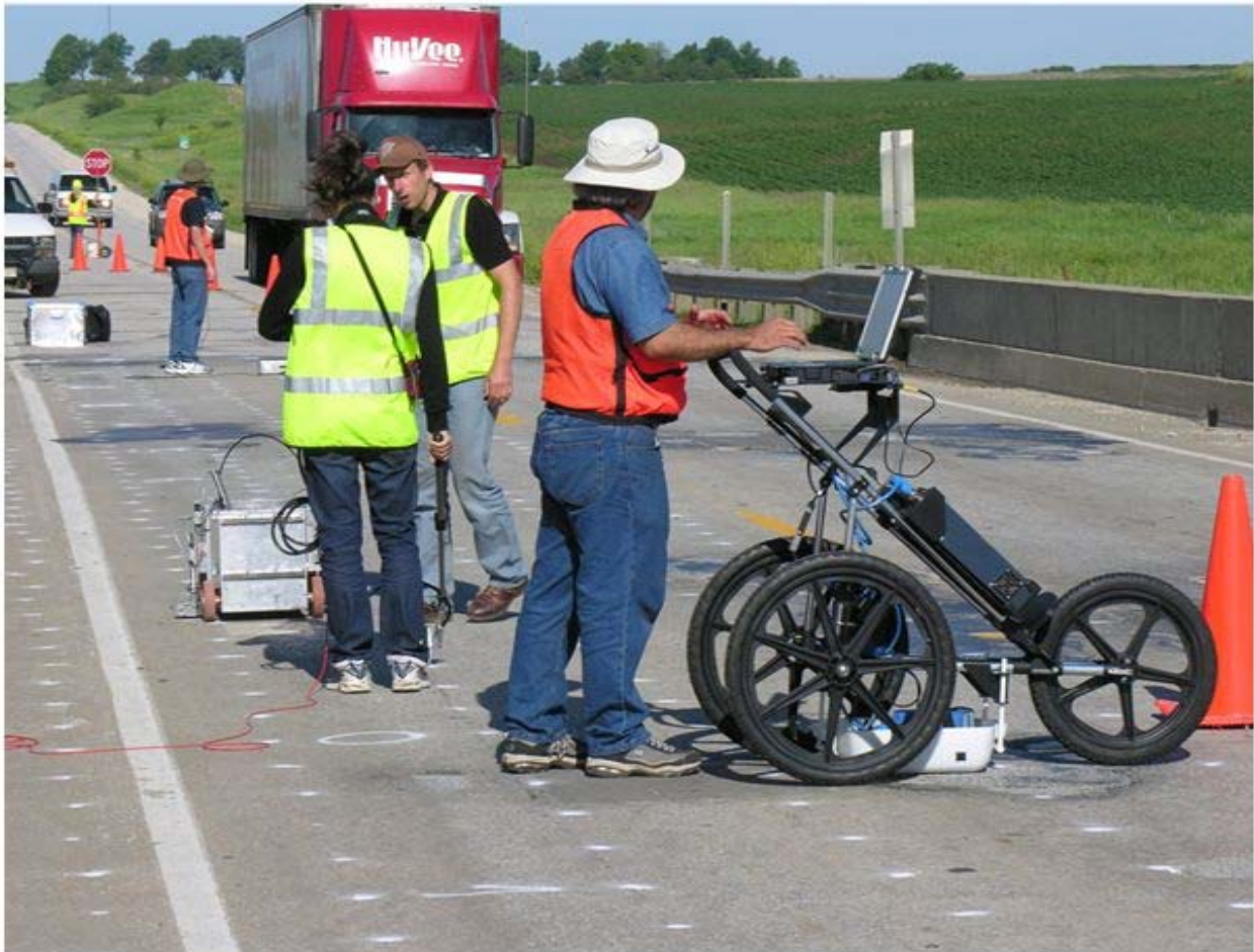
Figure 97. GPR data collection oriented perpendicular to traffic direction on slab decks, with other NDE methods unaffected by rebar orientation in upper mat.
