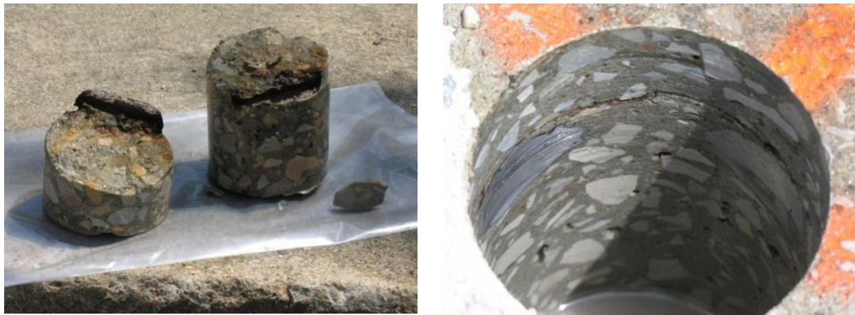
Figure 5: Corroded rebar in a deteriorated drill core (left) and delamination in a bore hole in a deck (right).
