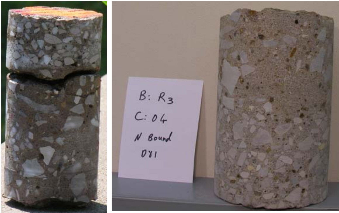
Figure 140. Cores 3 (left) and 4 (right), graded “serious” and “fair to poor” with IE.
