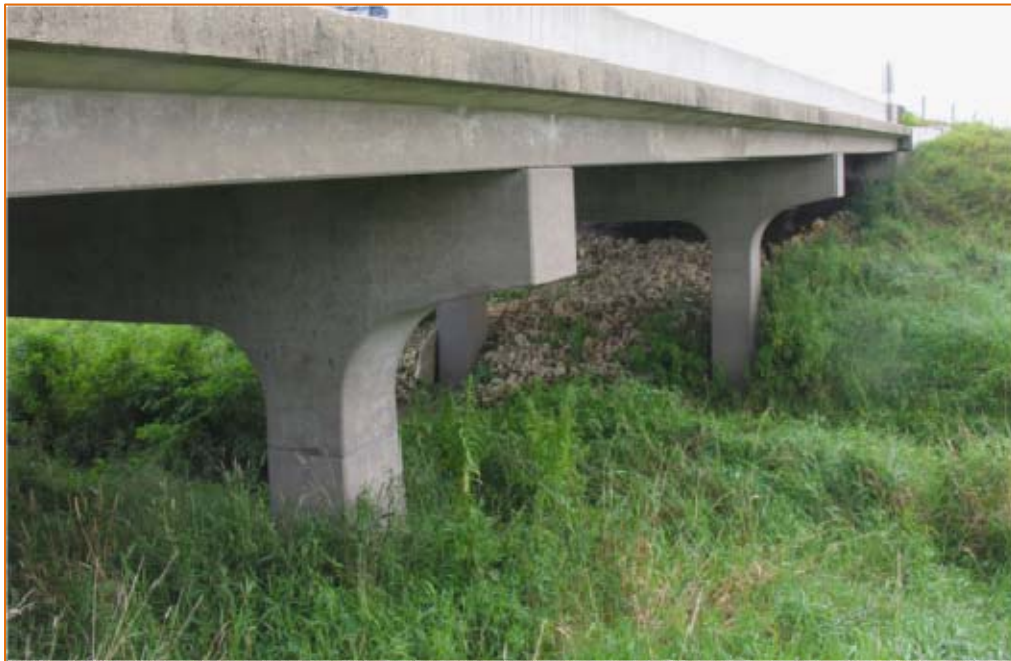
Figure 116. Side view of Deck R1 showing continuous slab construction on east face.
