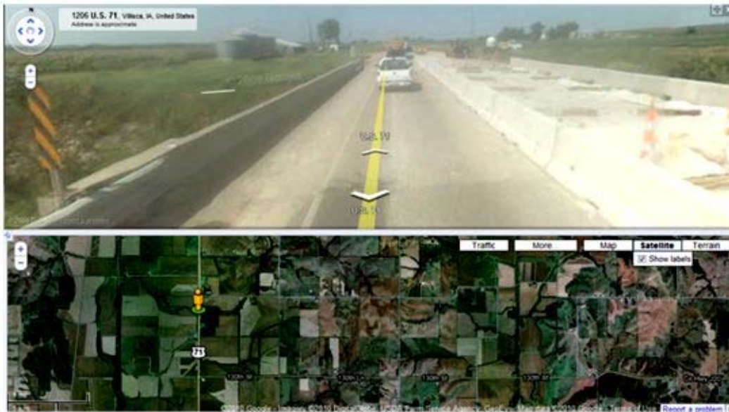
Figure 107. Google Map (photo taken in 2009) showing Deck O6 repairs underway on NB lanes, confirming negative deck skew.
