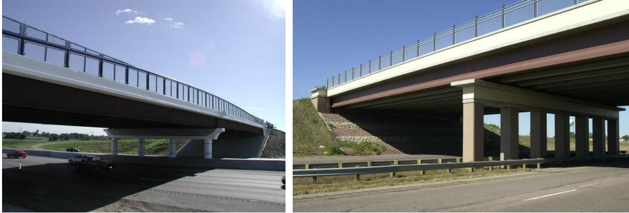
Figure 9.4.3. Level “B” bridge examples in Iowa
