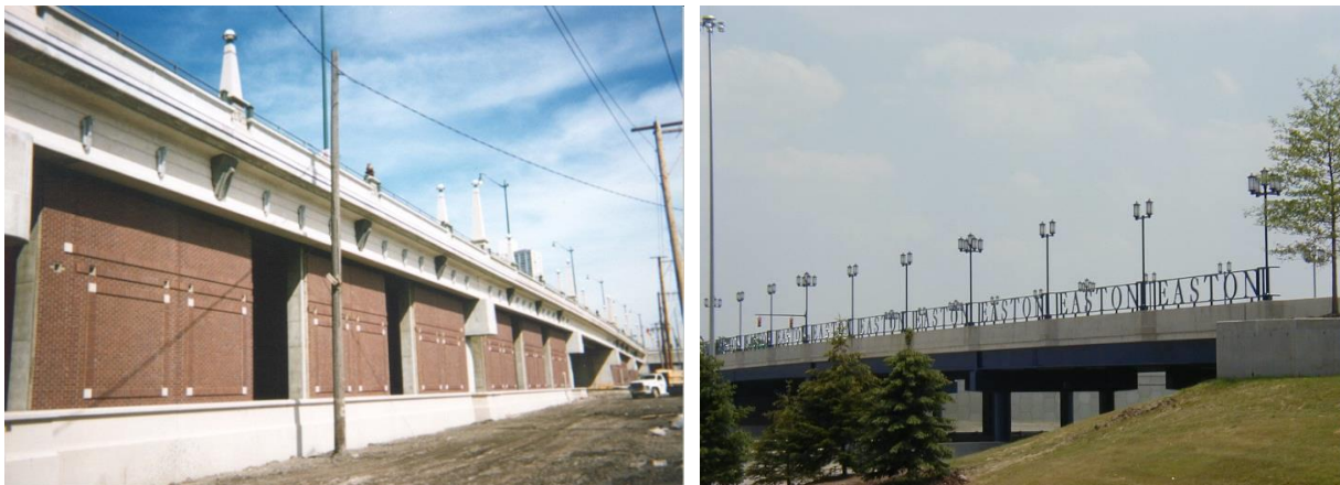
Figure 9.5.3.7-1. Bridges with ineffective bolt-on aesthetic details
