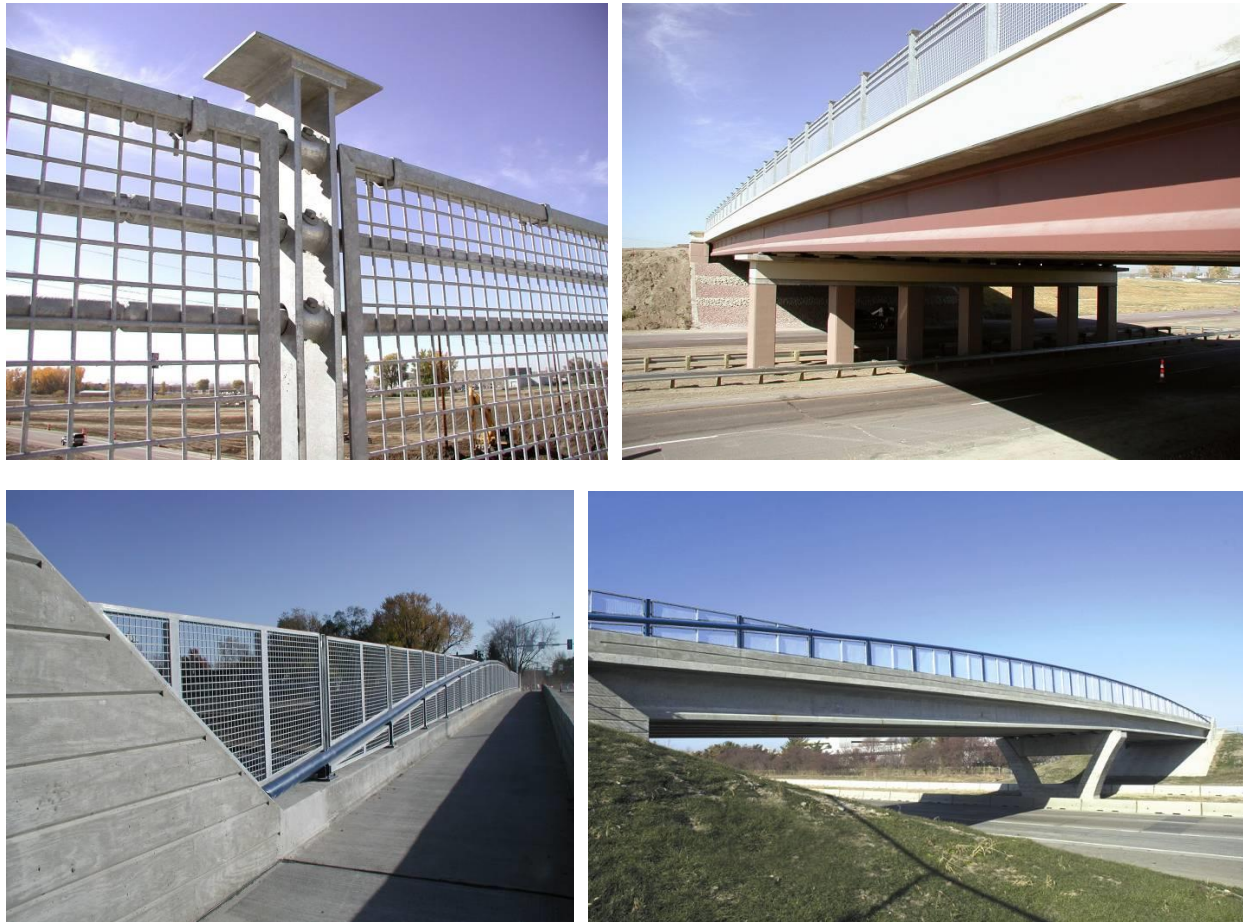
Figure 9.5.3.7-2. Bridges with complementary bolt-on aesthetic details
