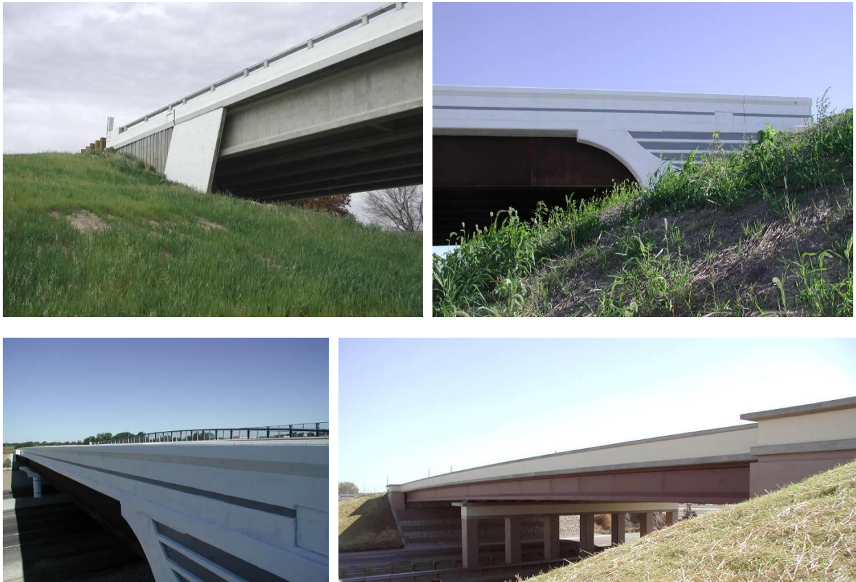
Figure 9.5.3.1. Bridges with long, slender appearance
