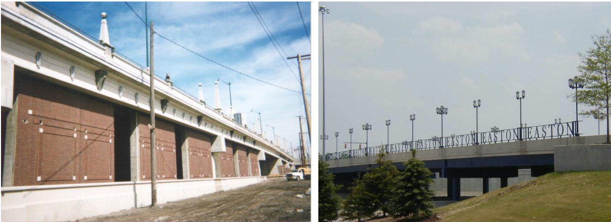
Figure 9.5.3.7-1. Bridges with ineffective bolt-on aesthetic details
