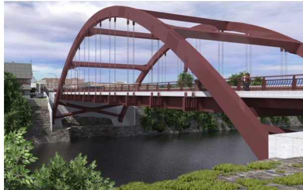
Figure 2.3.1-2 Replacement Steel Arch Bridge
