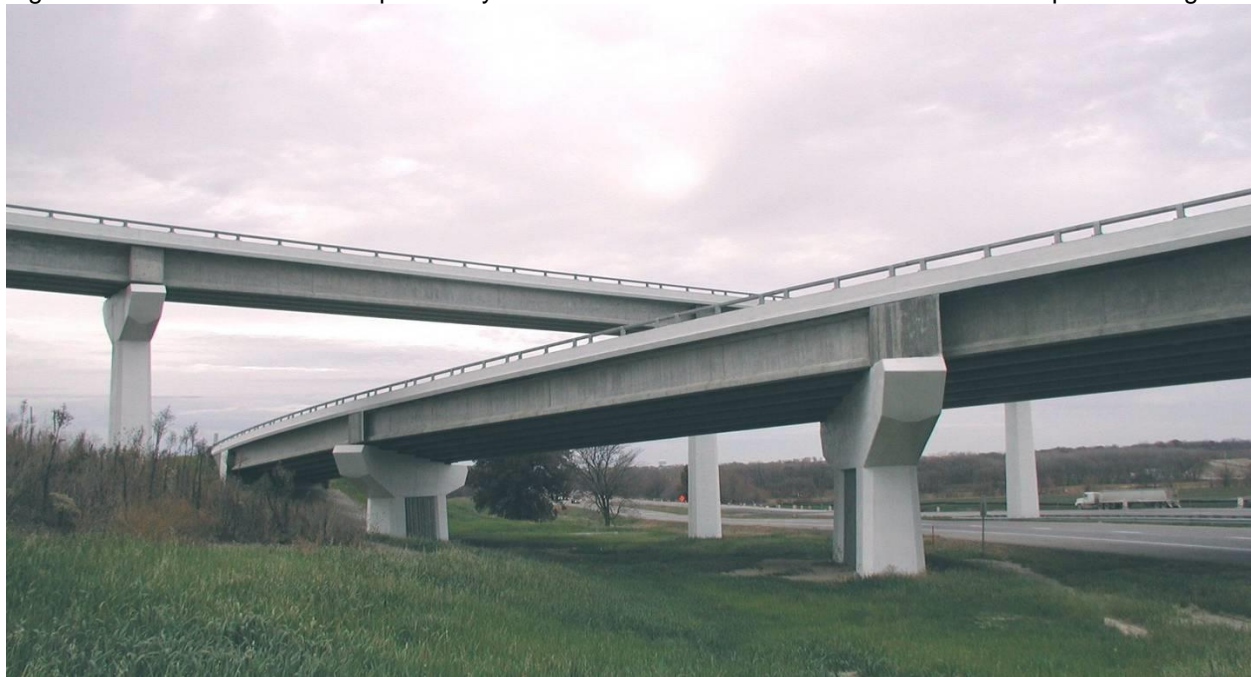
Figure 9.5.3.4. Bridges with minimal column count
