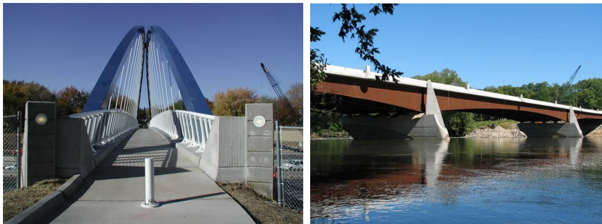
Figure 9.4.4. Level “A” bridge examples in Iowa
