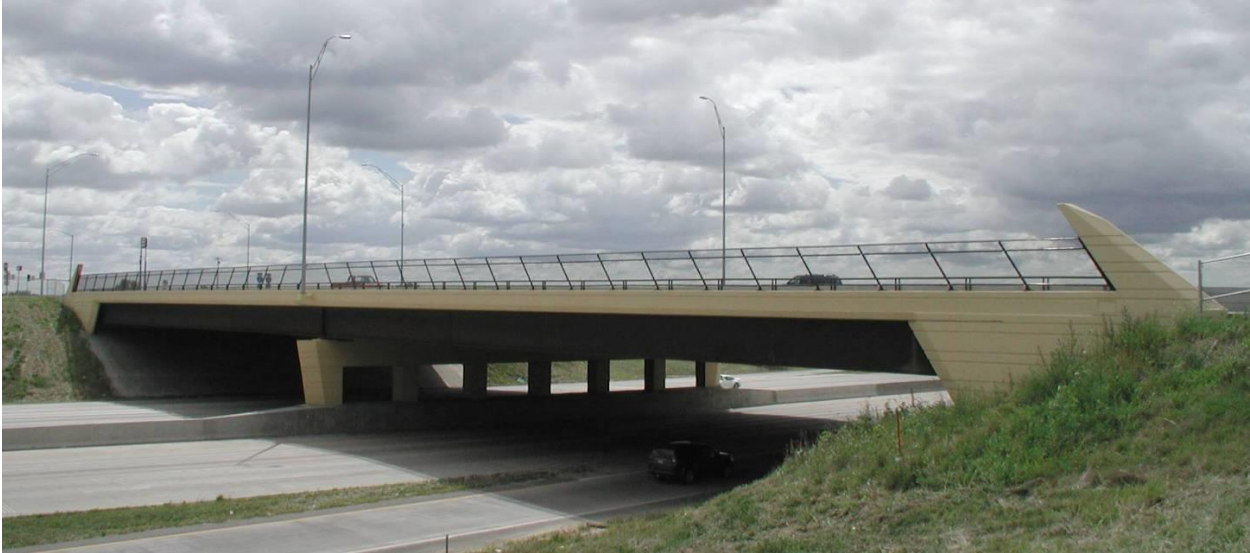
Figure 9.5.3.6. Bridge with sloping mask wall
