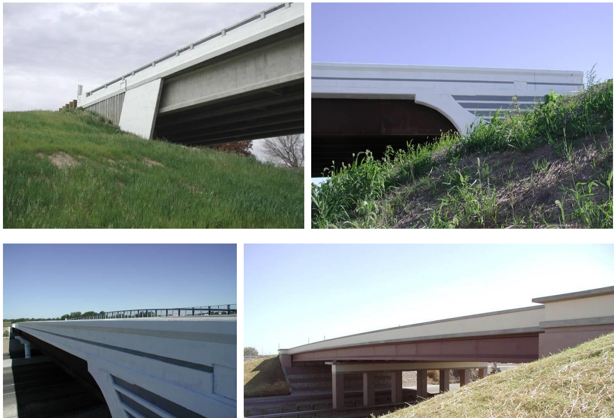
Figure 9.5.3.1. Bridges with long, slender appearance
