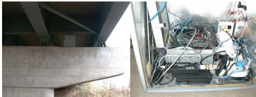
FIGURE 5. Photographs of Environmental Enclosure and CR 9000
