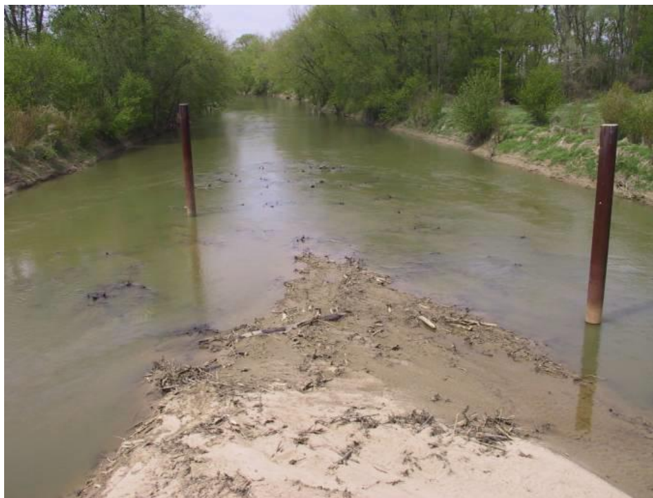
Figure 13. Single column debris deflectors (Lyn et al. 2003)
