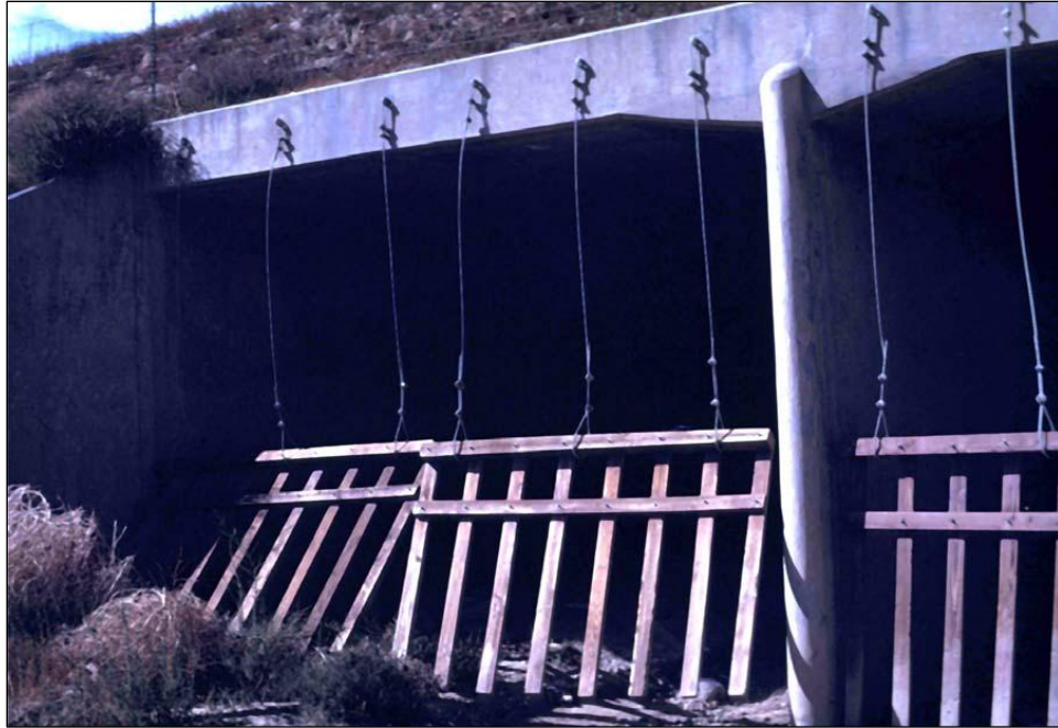
Figure 21. Timber debris rack (Bradley et al. 2005)
