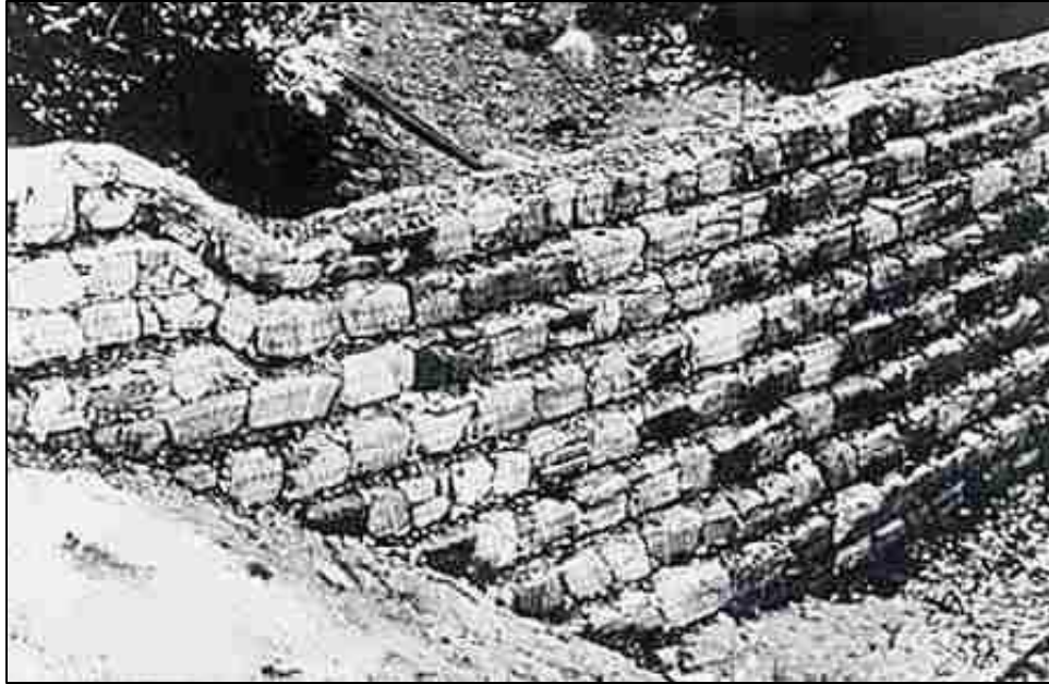
Figure 6. Debris basin constructed from gabions (Bradley et al. 2005)
