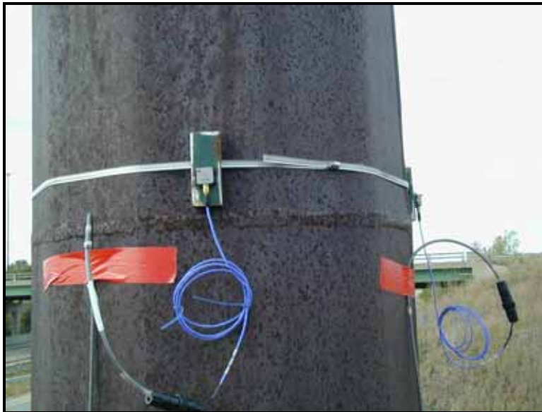
Figure 2.2 – Temporary accelerometer mounting used for the dynamic tests
