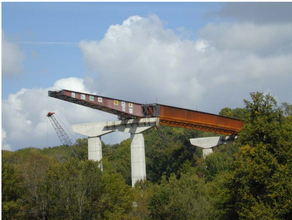
Figure 3.5. Launching nose cantilevered beyond Pier 4 (Eastbound bridge shown).
