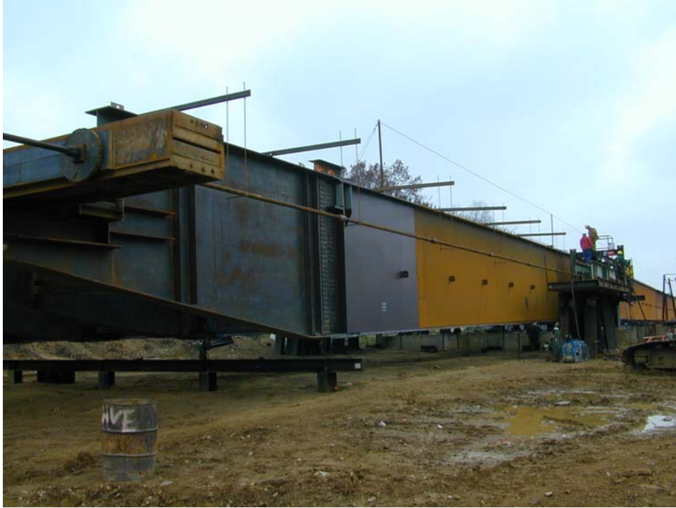
Figure 3.10. Complete jacking system.
