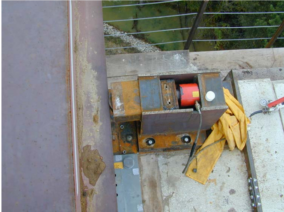
Figure 3.4. Guide roller equipped with 50-ton hydraulic jack.
