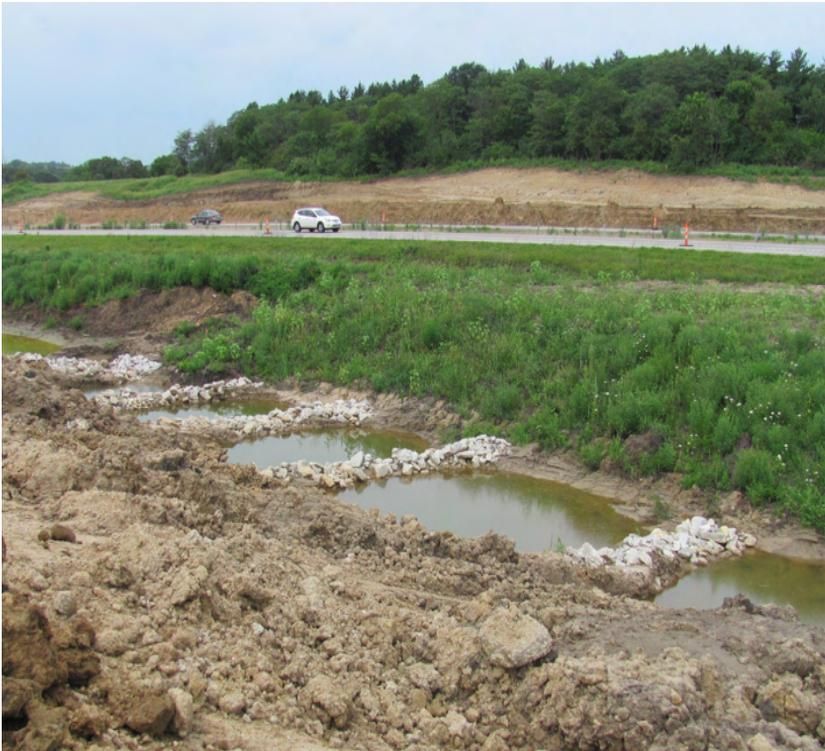
**Rock is used as a temporary sediment control in these Rock Check Dams.**
