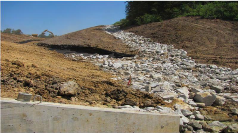
**These rock ditches were included in the design of the project due to the steep slopes and potential for erosion.**
