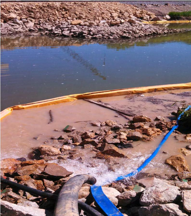
**Silt curtain used as a separation barrier to keep turbid water from entering the flowing water body. Additionally, the dewatering hose is outletted onto rock.**
