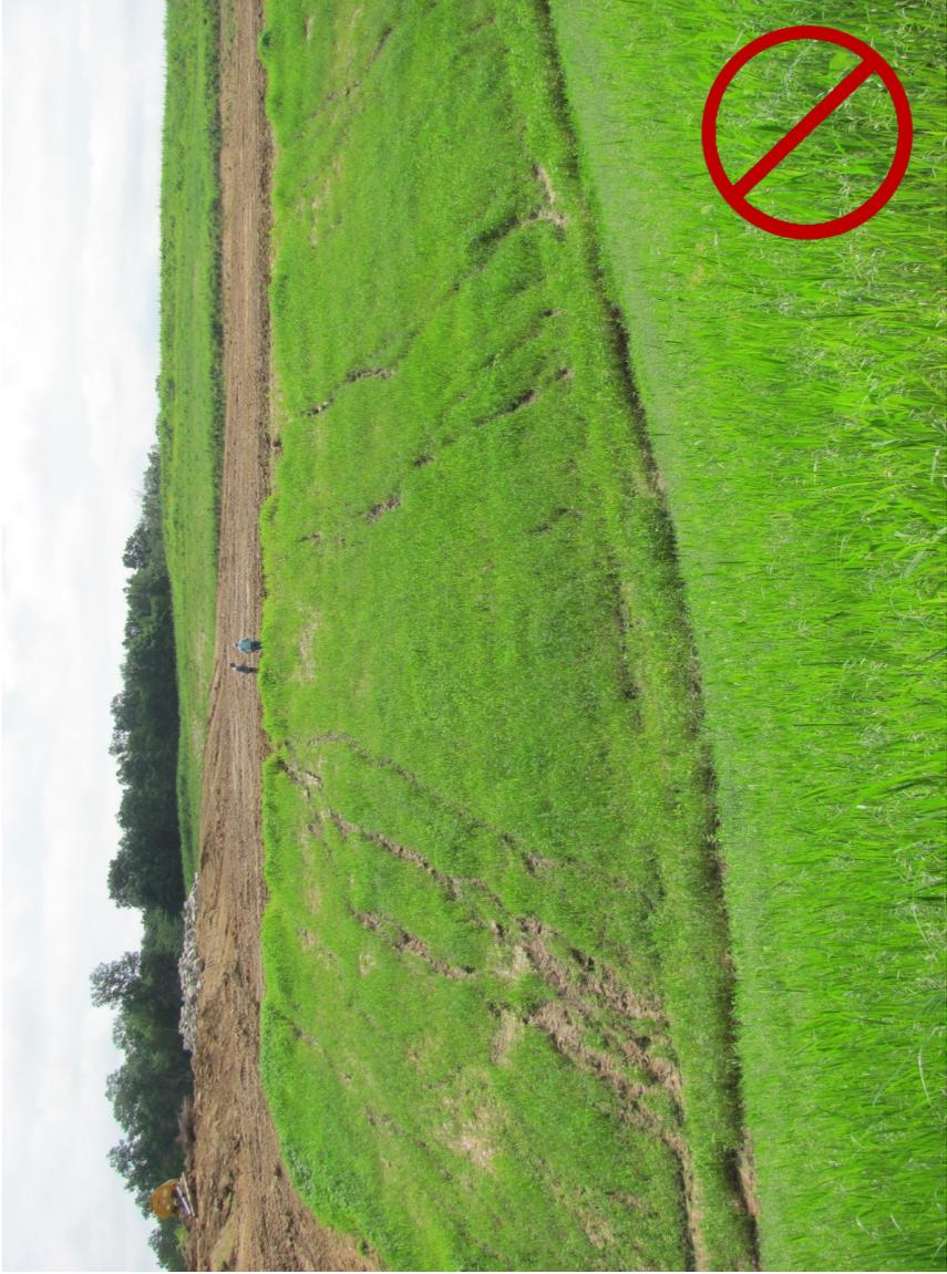
This trench was dug to divert flows down a rock flume and allow vegetation to grow on the slope.
