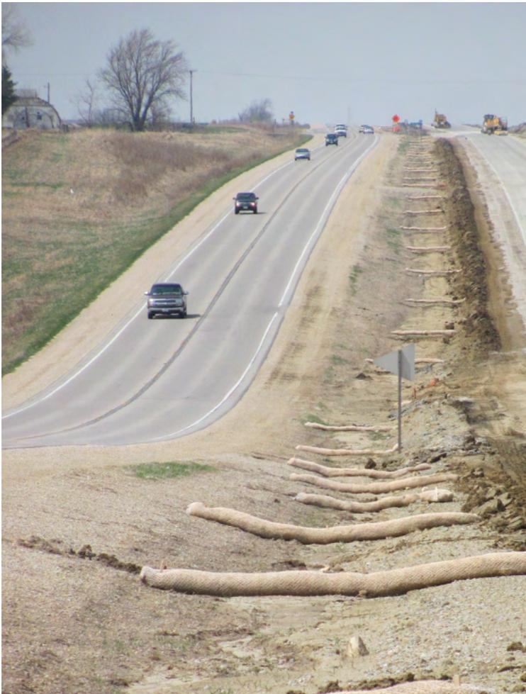
**Here logs worked well as ditch checks in a shallow median.**
