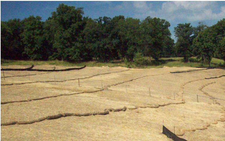
**Combining stabilization measures with structural measures is more effective than structural measures alone.**
