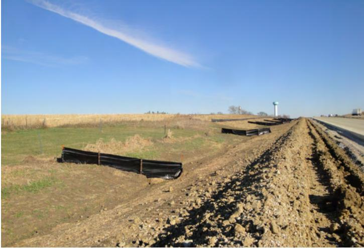
**This silt fence ditch check has been improperly installed. The end should extend into the slope on the right, otherwise storm water will just flow around the side.**
