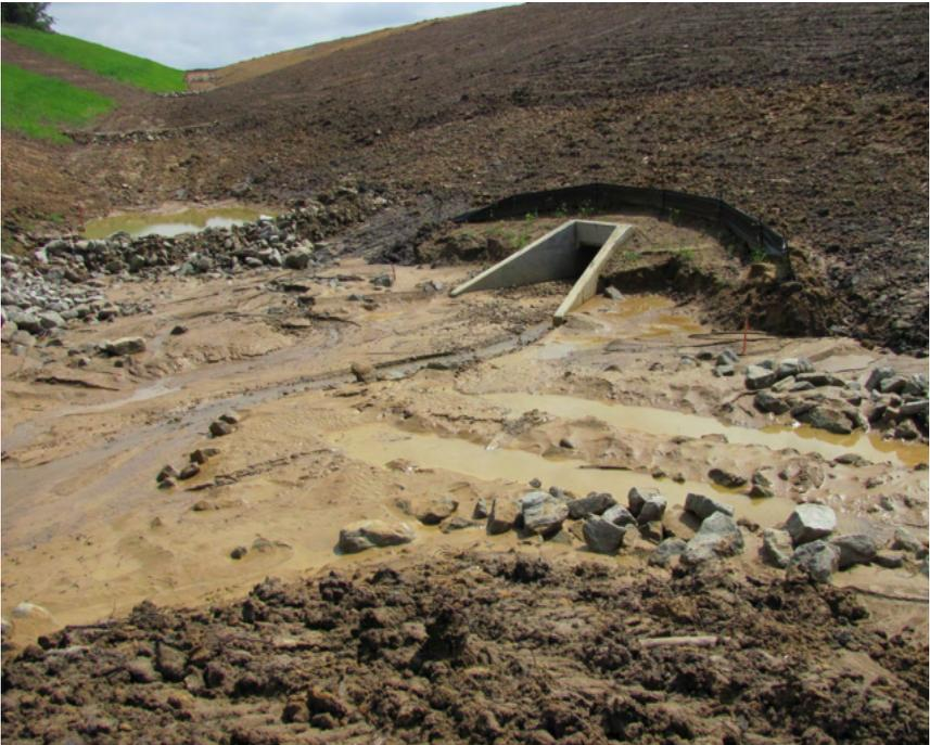
**The controls in this area are inadequate. This culvert and basin must be cleaned out, and the slopes need seeding, mulching, and additional silt fence.**
