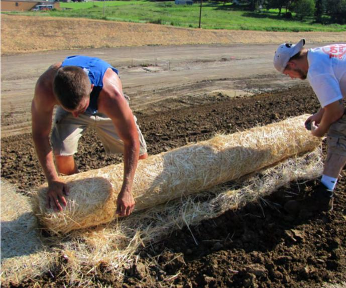
**This contractor is installing staples near the anchor slot.**
