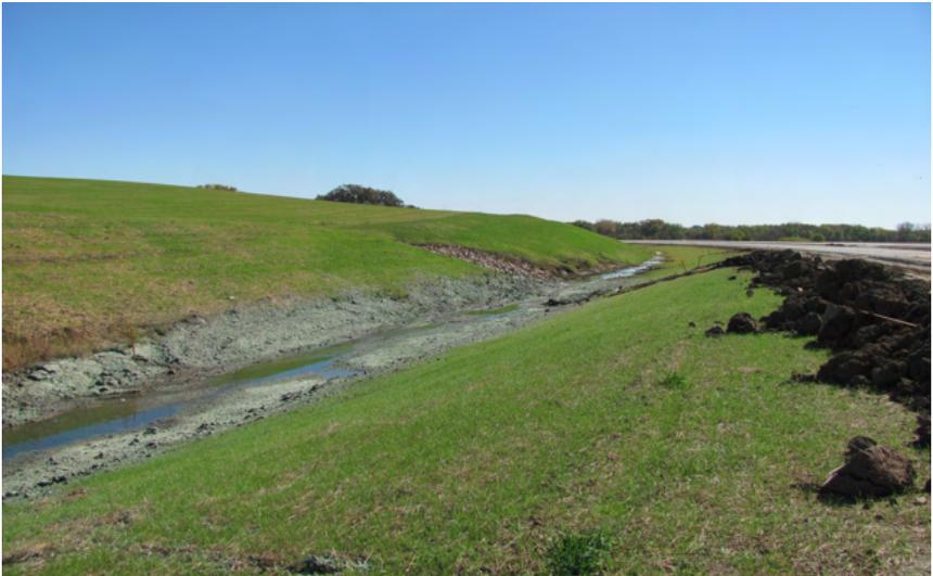
**An example of an area where the contractor used hydraulic seeding and mulching to reseed an area that was wet and would have been difficult to access.**
