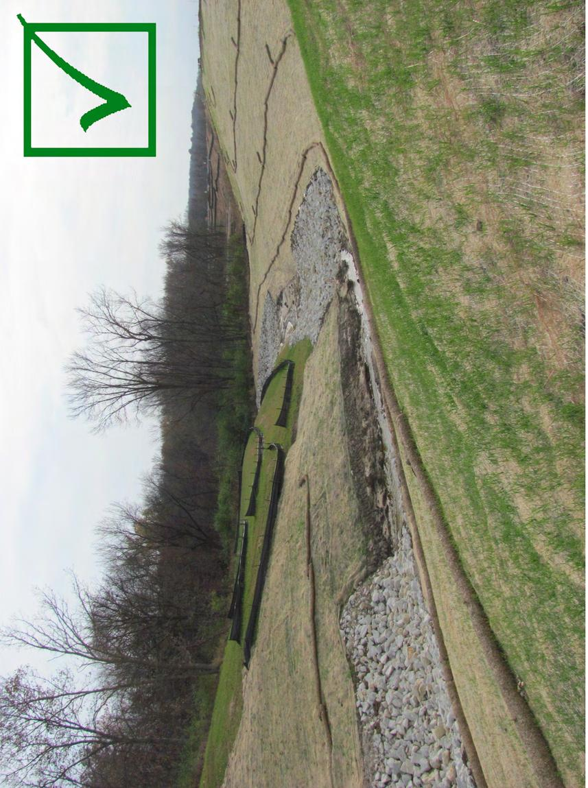
This is an example of a good temporary stream crossing per EW-401. Clean fill was used in the creek, and the crossing was topped with aggregate.
