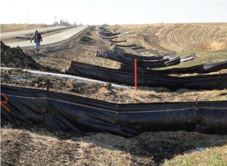
**This photo shows a chain of silt fence ditch checks installed to slow velocity of water and collect sediment from flowing downstream.**
