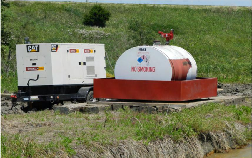
**Fuel tanks should have a secondary containment area large enough to handle a potential spill in locations that have potential to discharge to storm drain systems and waters of the state.**
