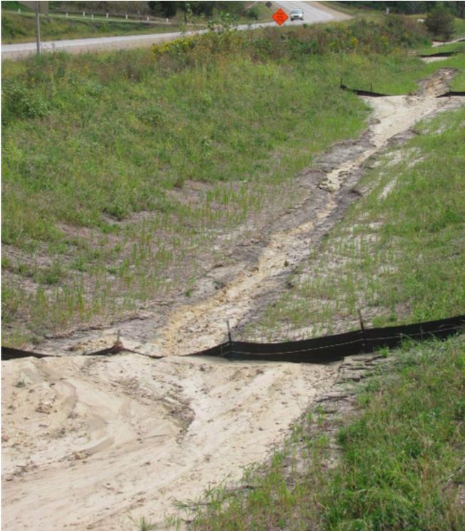
**Silt fence ditch checks at capacity require removal and replacement or clean-out.**
