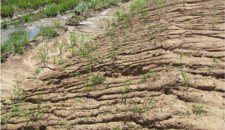
**Rill erosion should be repaired prior to seeding.**
