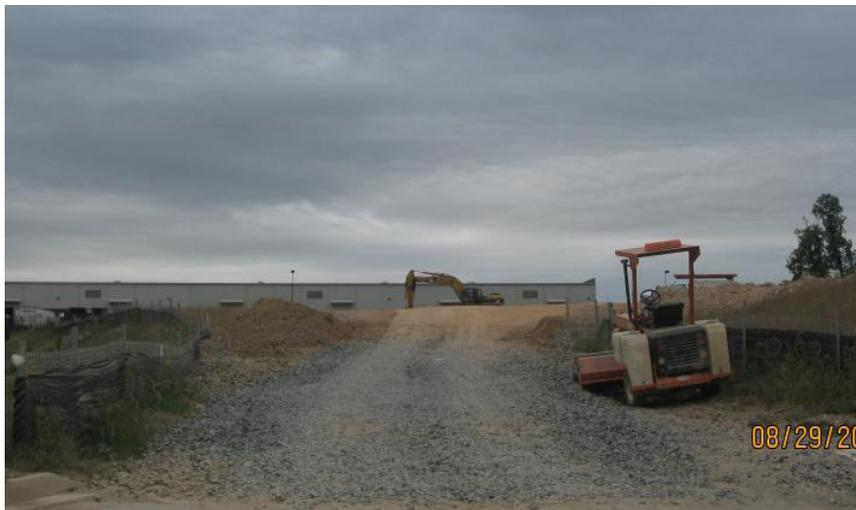
**This is an example of a stabilized construction entrance. This is one type of control to prevent tracking onto a roadway.**
