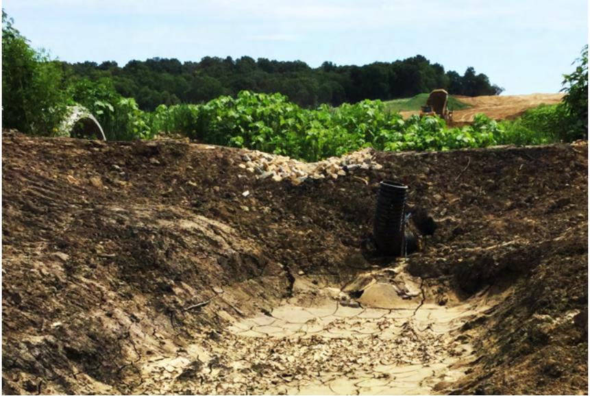
**Above, inlet of riser pipe and berm with rock overflow.**
