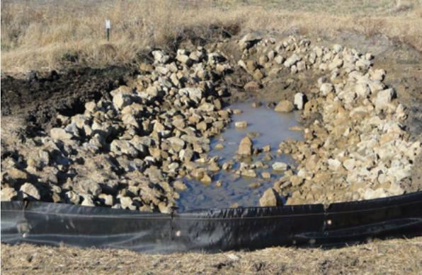
**Riprap has been placed around this inlet to prevent erosion. Silt fence has been placed to prevent sediment from entering the inlet.**
