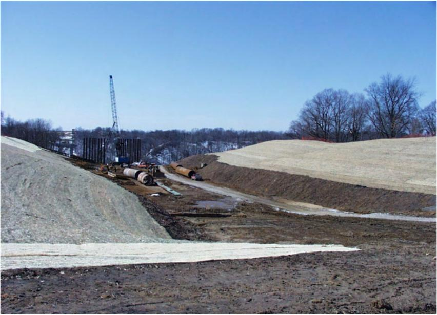
**Slope protection slows run-off and keeps the soil moist while seed germinates.**
