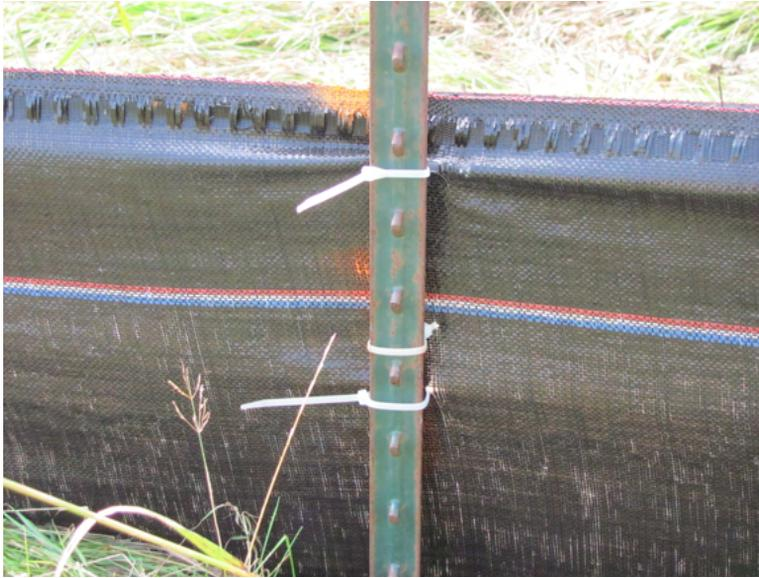
**This silt fence was tied with the correct number of ties, but the top tie does not encompass the belt and the bottom tie should be about 4" from the ground.**
