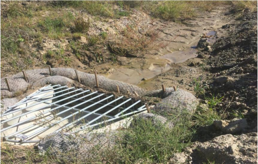
**Logs/wattles/socks are good controls for culvert inlet protection.**
