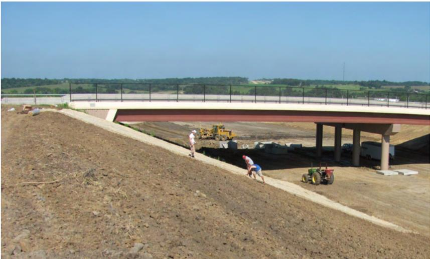
**Installation of slope protection on a slope near a bridge.**
