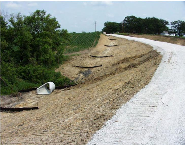
**The steeper the ditch grade, the closer silt fence ditch checks should be installed.**
