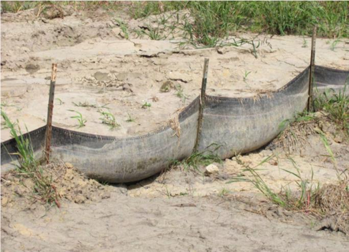
**Silt fences at capacity should be noted on the weekly inspection report as a deficiency.**
