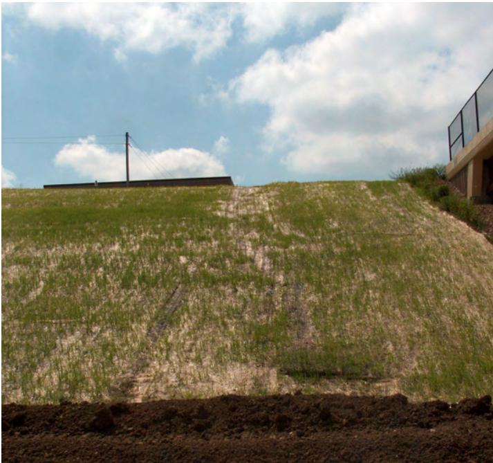
**Speed of growth depends on temperature and rainfall. This photo was taken three weeks after installation of the blanket.**
