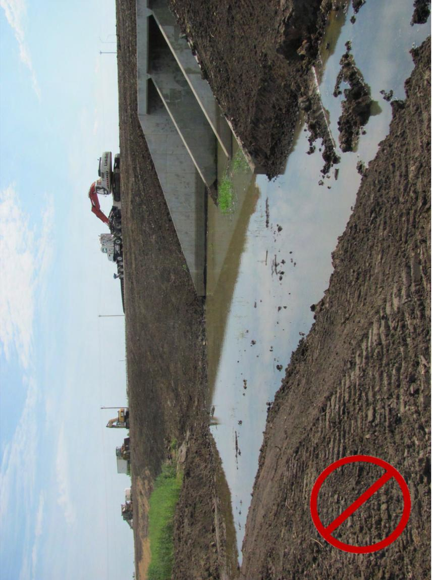
This box culvert has multiple controls installed, including slope protection, multiple rows of silt fence, and rock.
