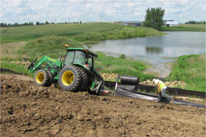
**This silt fence installation machine is trenching in the fabric. Following this step, posts will be installed and the fabric attached to the posts.**
