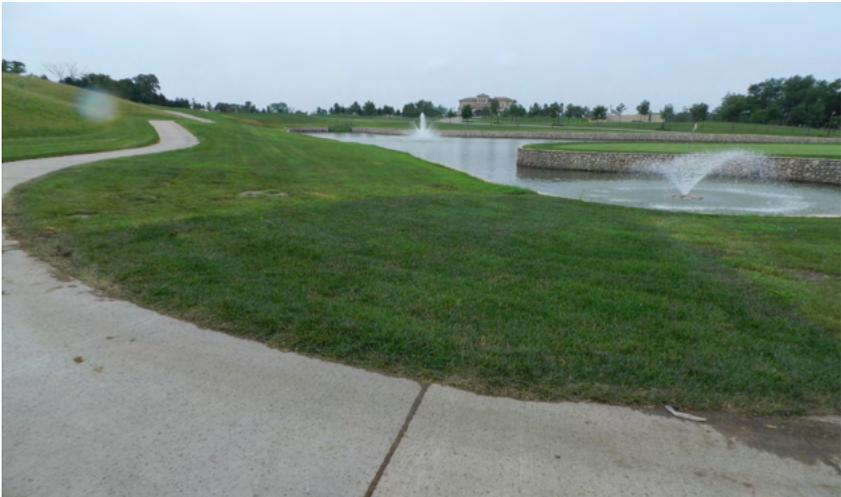
**On Iowa DOT projects, sod might be used to establish vegetation in commercial or residential areas. Following the requirements for watering and sod application are important to keep the sod healthy.**
