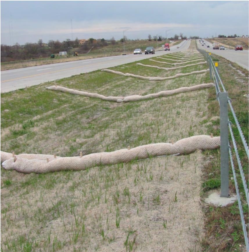
**Use of sediment logs as ditch checks over special ditch control.**
