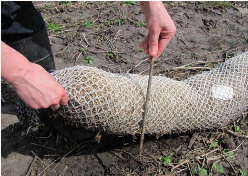
**Devices should be installed with proper staking. This photo shows improper staking using a metal nail.**
