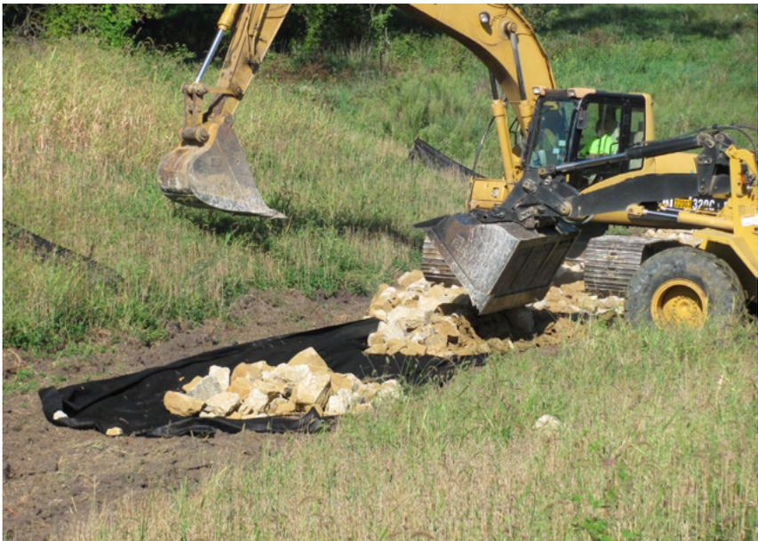
**A contractor is installing riprap on top of engineering fabric to create a rock ditch.**
