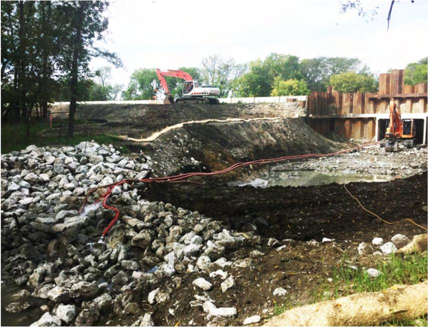
**Example of a temporary stream diversion using bypass pumping.**
