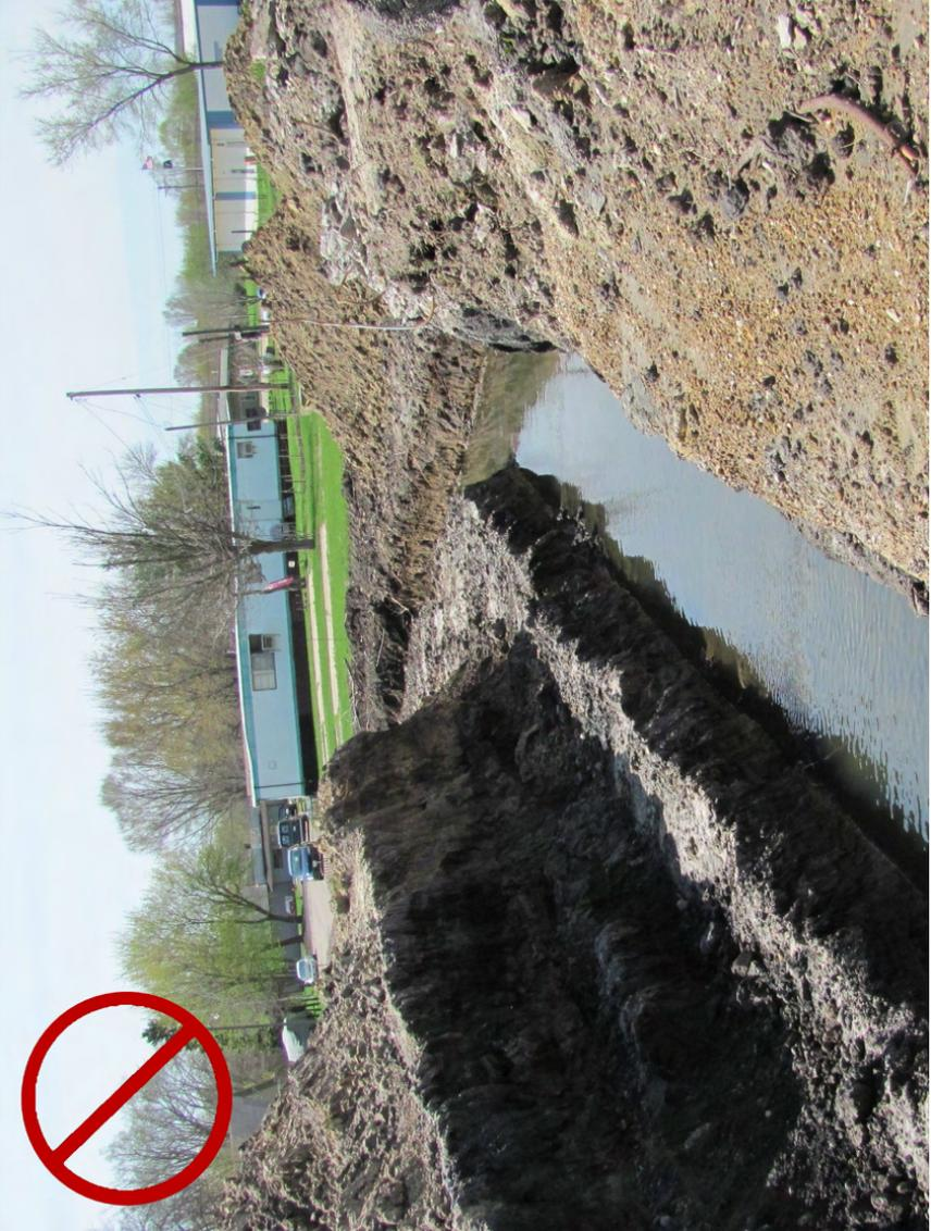
This shows a good example of a temporary stream diversion installed per EW-402.
