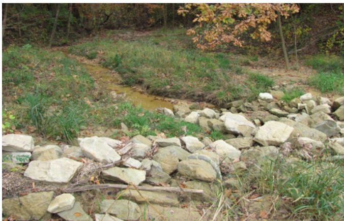
**This rock ditch and ditch check are the last line of defense to prevent sediment from entering the stream.**
