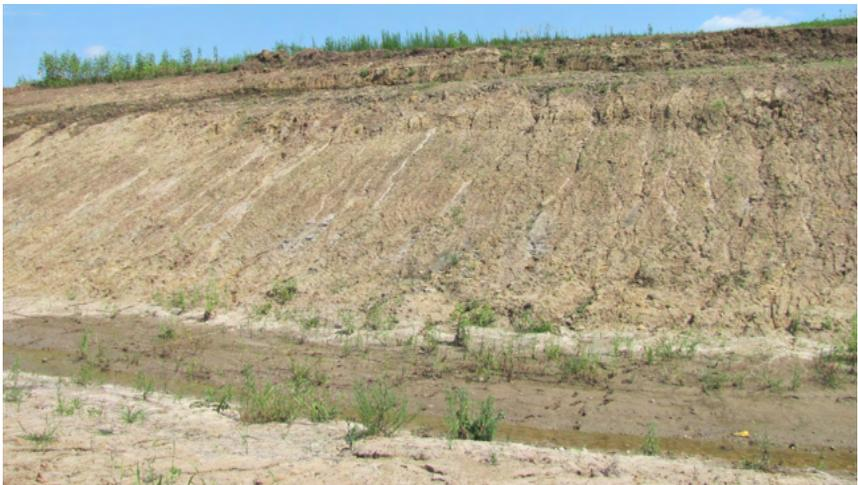
**Rills are an indication that this area has not been worked on for an extended period of time. This area should be repaired by harrowing and deeper gullies may need additional repair. The area should be seeded and mulched or possibly matted.**
