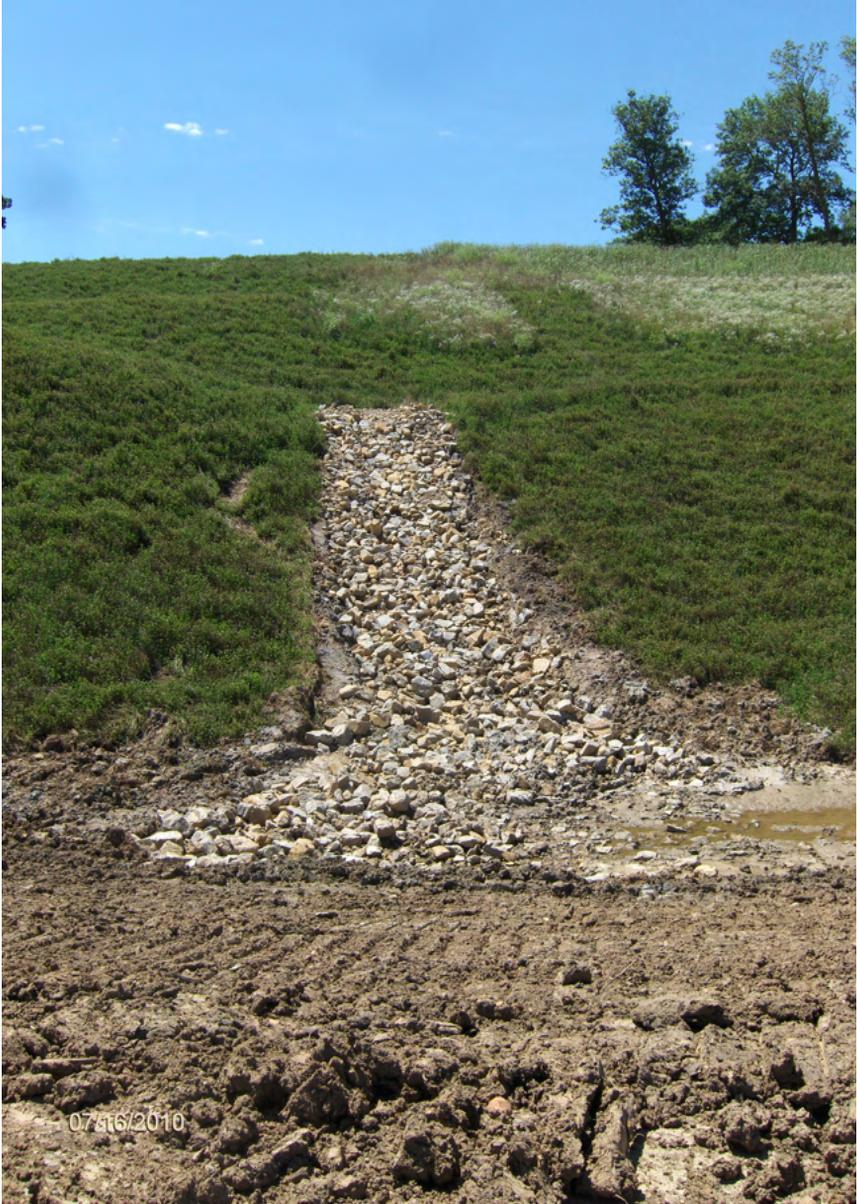
**Rock flume installed to convey flows from a backslope bench.**
