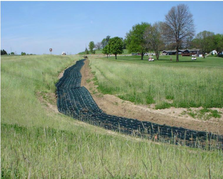
**Here TRM was used in a ditch that has potential for high velocity flows.**
