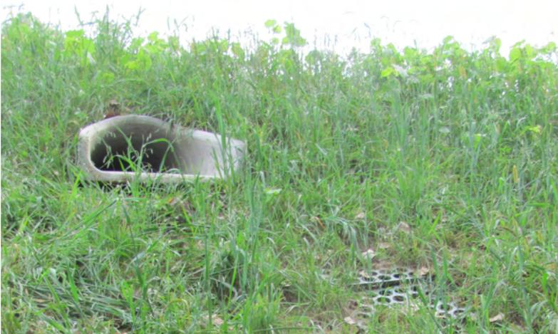
**Transition Mat used at a pipe culvert outlet.**
