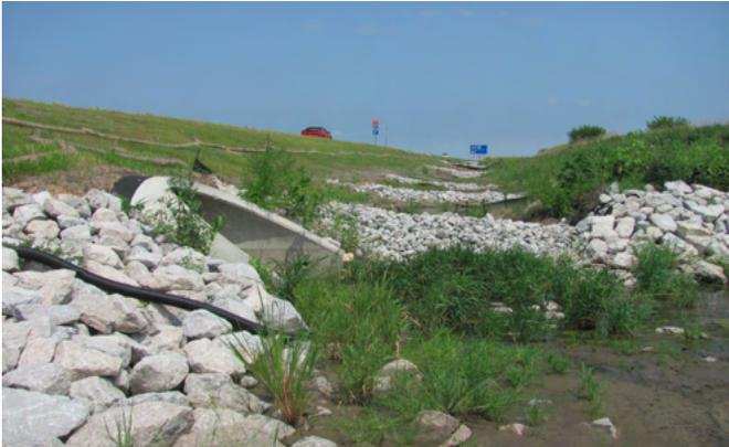
**This photo shows rock ditch checks, silt basins, silt fence, logs, and temporary vegetation used to protect a discharge point.**
