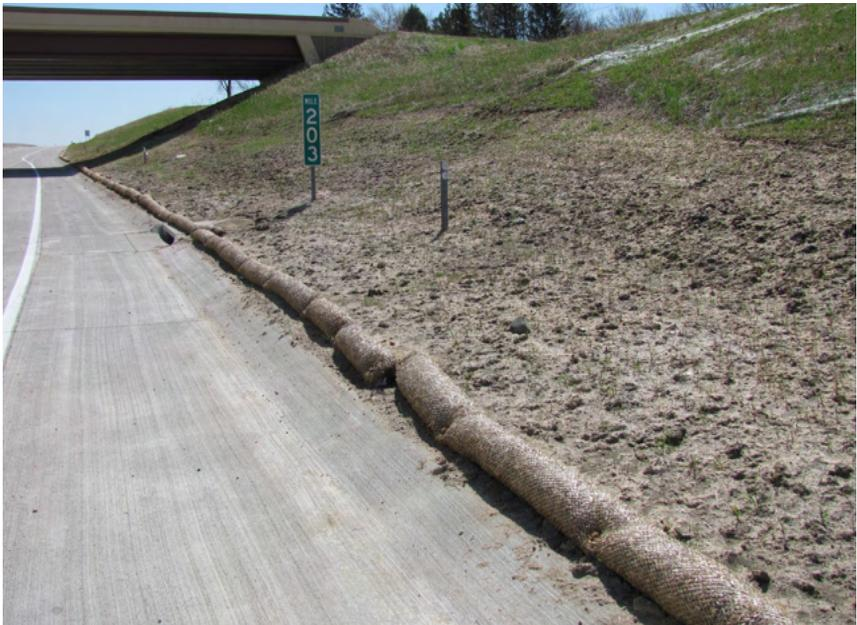
**Wattles installed at back of curb to prevent sediment from washing onto the road.**
