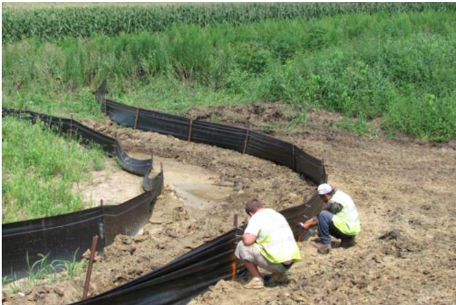
**This is an example of a second silt fence being placed as a replacement where the existing fence was blown out. To be more effective, the new fence should have been installed downstream of the existing fence.**
