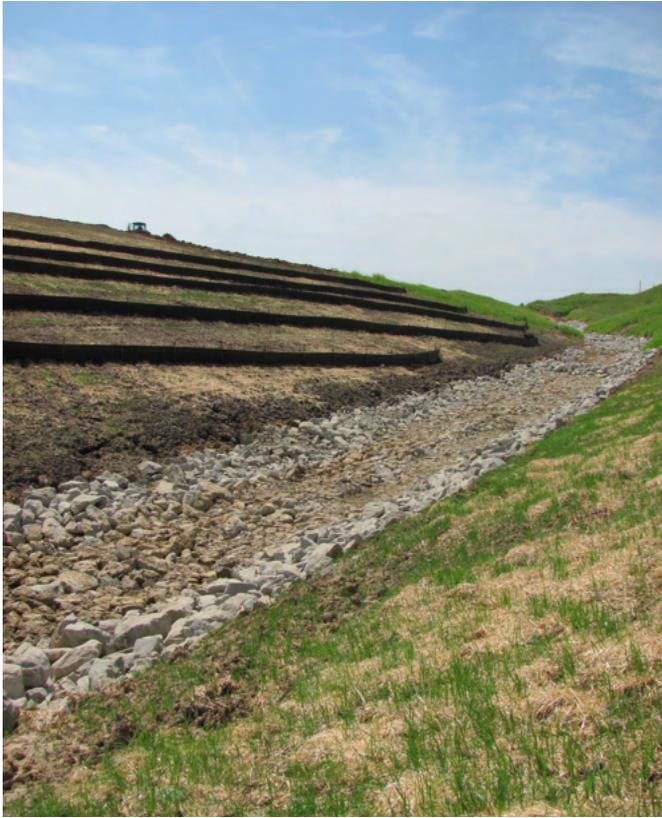
**Multiple rows of silt fence installed along the contour of this foreslope.**
