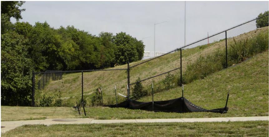
**Don't forget to remove the old silt fence and posts once the area has reached a density of 70%. Posts should be pulled and silt fence should be cut off at ground level or completely removed.**
