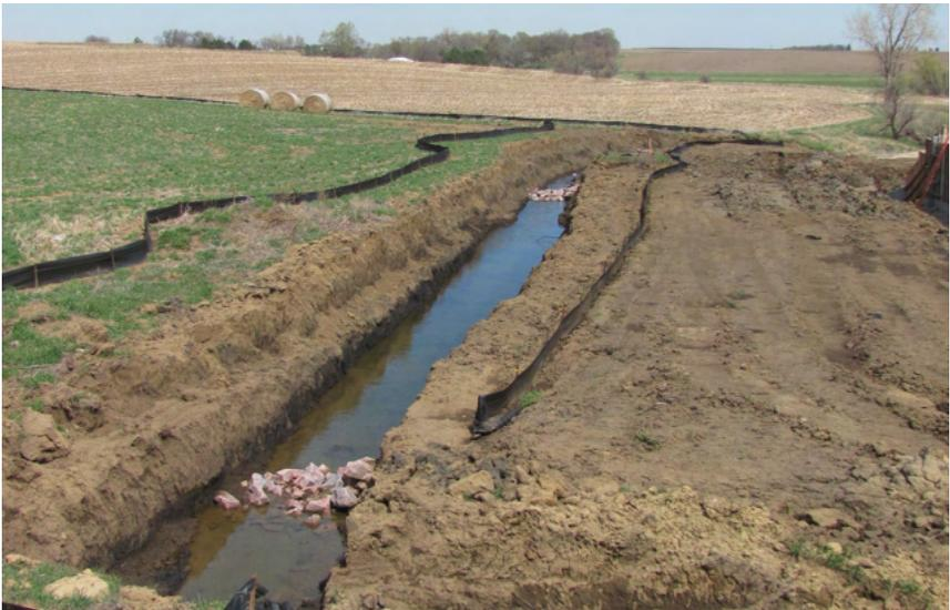
**Temporary stream diversion showing a diversion channel and upland sediment controls.**
