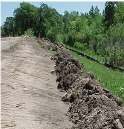
**Vegetated buffer used with silt fence and topsoil berm.**
