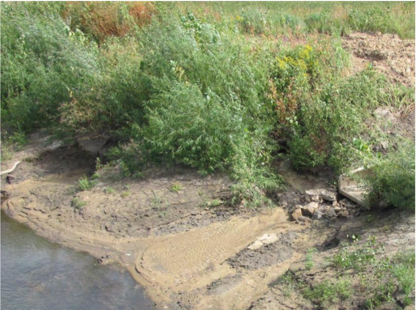
**This pipe outlet does not have a splash basin, and erosion is occurring.**
