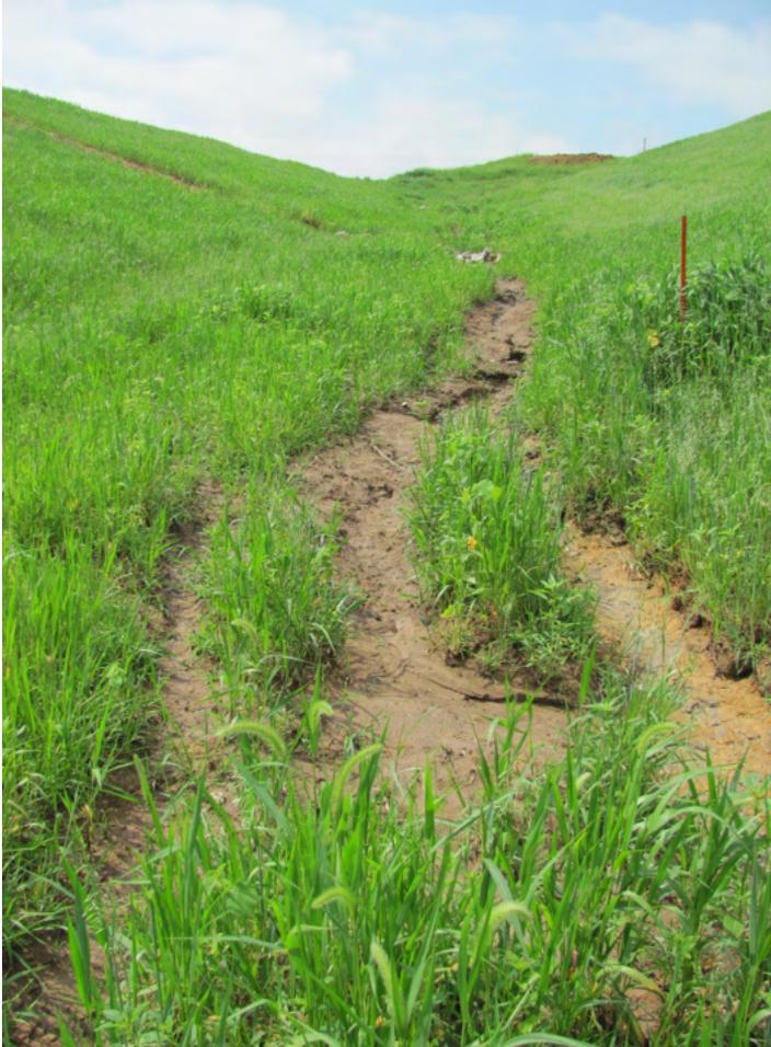
**Erosion can occur in vegetated areas, such as this ditch which was seeded and mulched.**
