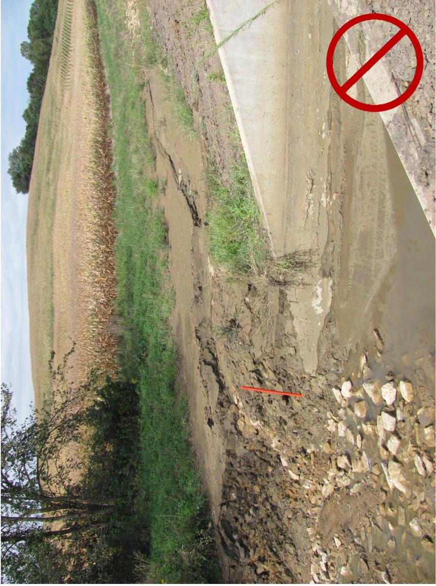
This site used multiple controls, including silt fence with J-hooks, mat, staged seeding, logs and rock.
