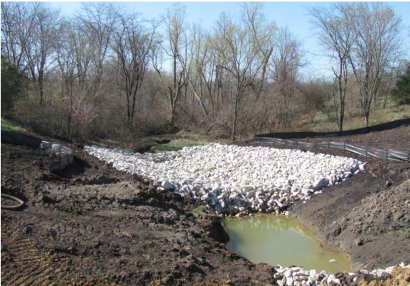
**This is a silt basin and rock used together as sediment controls prior to water discharging offsite.**
