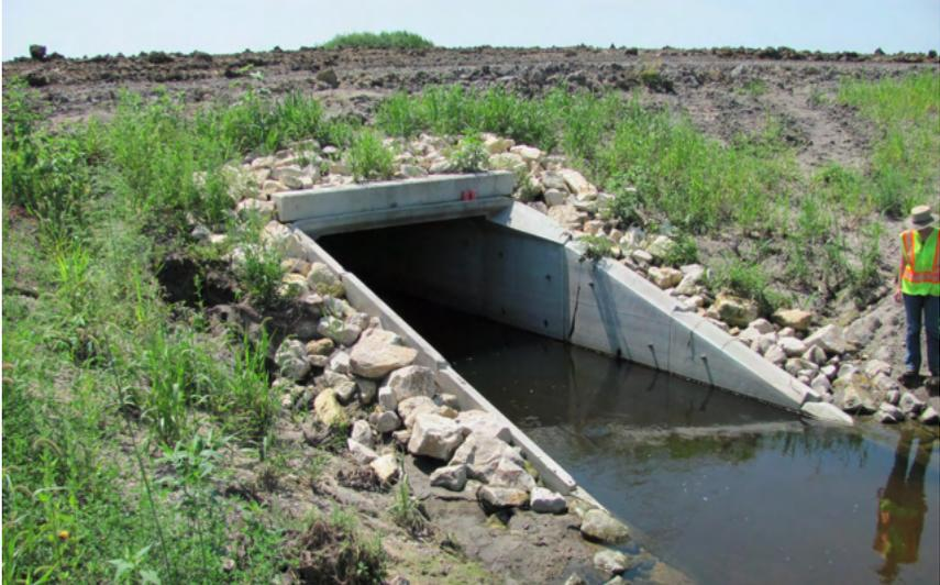
**Washouts along culverts and bridges should be repaired before they turn into gullies, such as shown in the photo. The slope should be repaired and seeded.**
