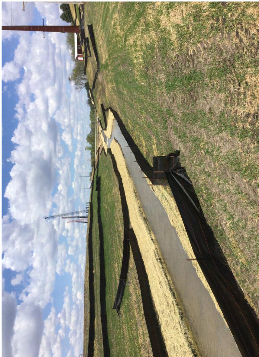
**This is a great example of erosion and sediment control used in combination to protect a stream.**
