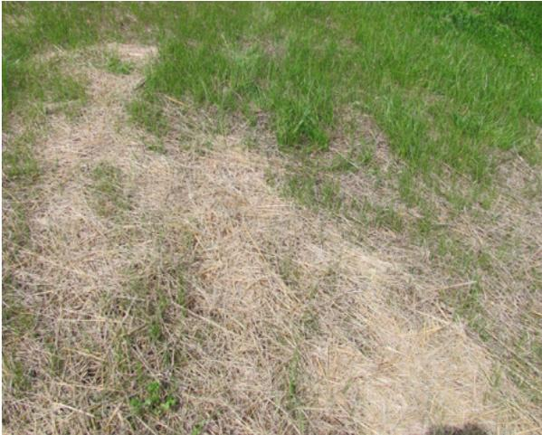
Mulch should be anchored a minimum of two inches into the ground surface with two passes of the mulch anchoring equipment. If not anchored, the mulch will blow or wash away easily.
