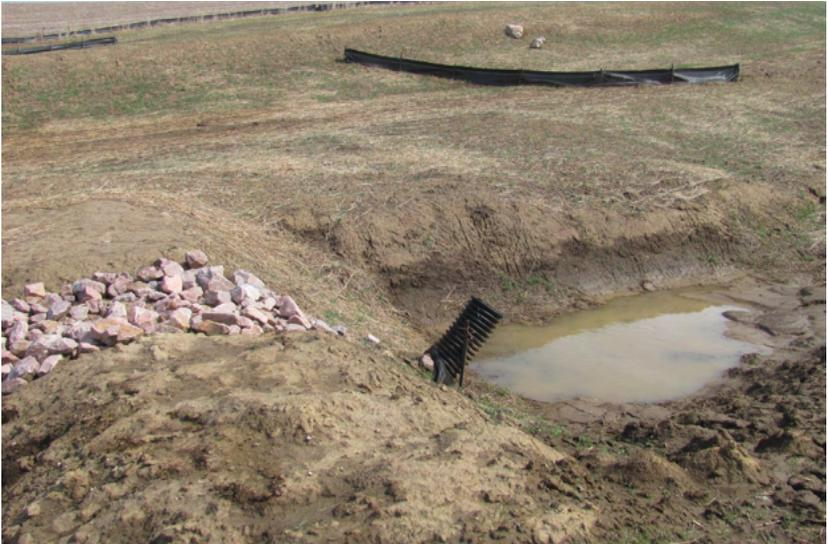
**Temporary sediment control basin showing the upstream riser pipe and erosion stone overflow.**
