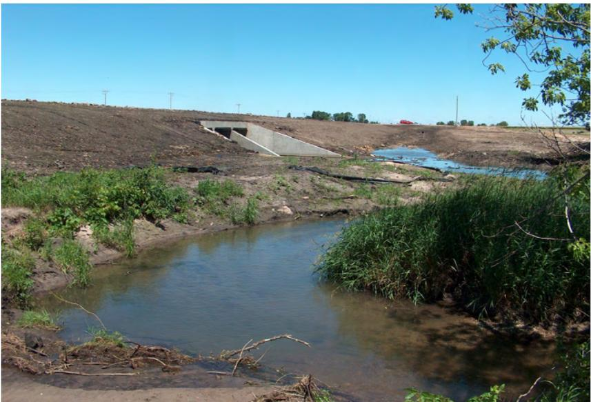
**Failure to install proper erosion and sediment controls in a timely manner can result in damage to the environment and costly fines.**
