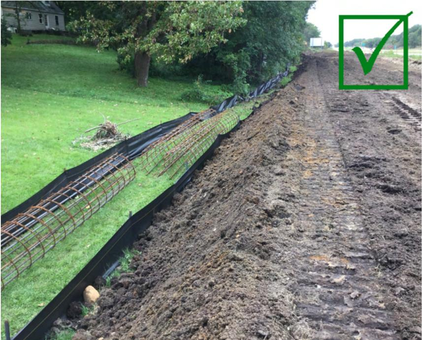
Two rows of silt fence were installed at this location because the project site was adjacent to a residential area.
