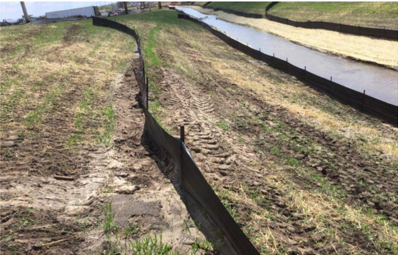
**This photo shows a silt fence that was cleaned out. However, the removed silt was incorrectly placed in front of the silt fence.**
