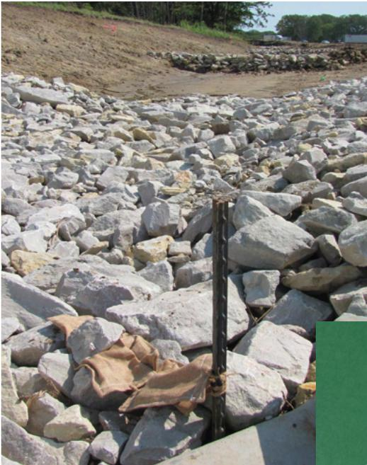
**Left, flocculant bag used upstream of Rock Check Dams.**
