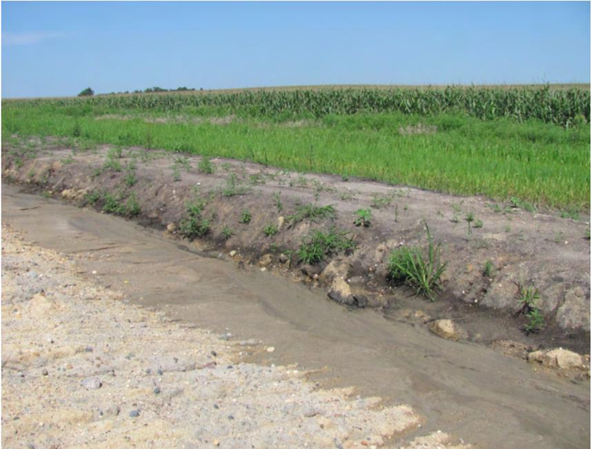
**Example of silt dike used on a grading project. This silt dike should also have temporary stabilization.**
