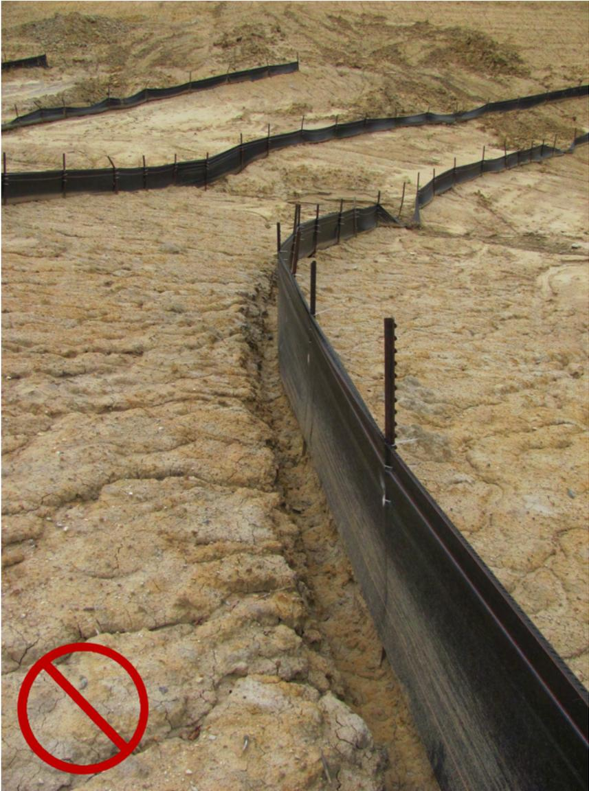
Water ran along the silt fence, down the slope, and created a channel. The silt fence was then overwhelmed at one location, and a blow out occurred. Silt fence was also installed in too large of a span and should have been broken up into smaller sections with J-hooks. This would have created multiple storage areas and prevented a channel from forming along the side of the fence.
