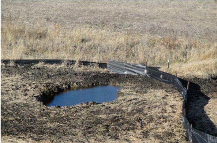
**This is an improperly sized silt basin and will not function as required, because it will not provide time for sediment to settle.**
