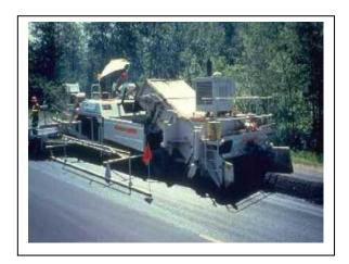
pavement surface and not allow the windrow to extend more than two truckloads in front of the paver to avoid excessive cooling of the mix.
