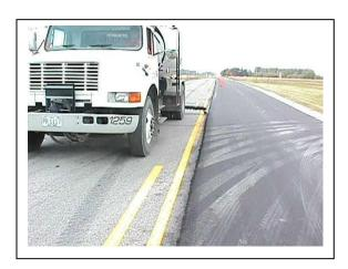
The spray bars must be adjustable for the widths of application required by the work.
