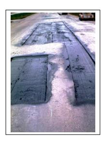
inch but less than the total thickness of the old pavement. The areas are cleaned, tack coated and filled with hot mix in lifts not to exceed three inches. A weighted pneumatic tire or mechanical tamper may be used to compact the mix. The final compacted surface shall be level with to ½" above the surrounding surface.
