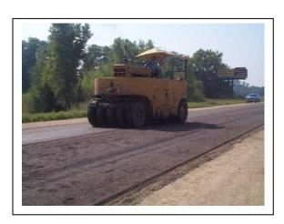
CIR is typically performed between May 1 and October 1, followed by an overlay or surface treatment. Any subsequent treatment or HMA overlay placement cannot occur until the in-place recycled pavement meets applicable moisture content and/or drying period criteria listed in Specification 2318.
