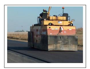
Intermediate rolling is commonly seen on interstate and higher volume primary paving projects, which typically use stiffer mixes and higher crushed aggregate contents.
