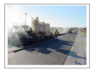
Increasing plant mix temperature, covering hauling units, minimizing haul length, and shortening windrows in front of pickup machines can all minimize the effects of the environment on HMA paving.
