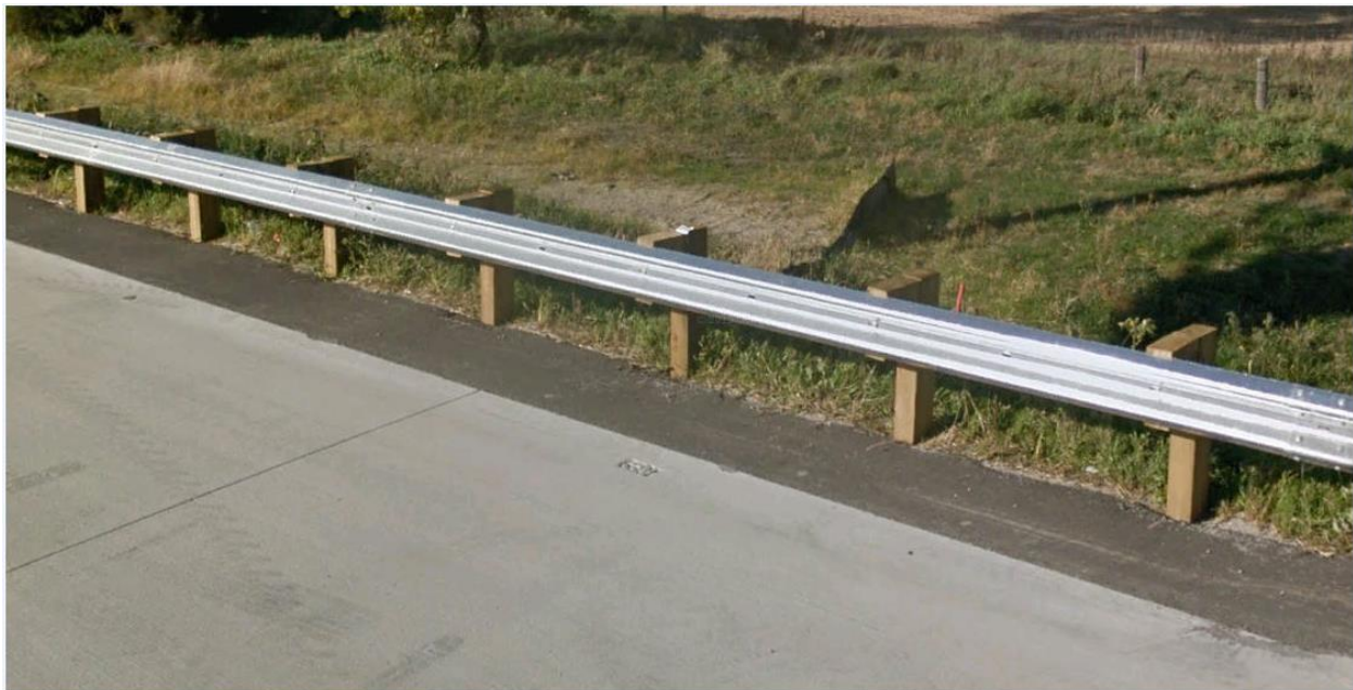
Figure 1: Steel beam guardrail.
