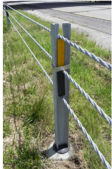
High tension cable guardrail example
