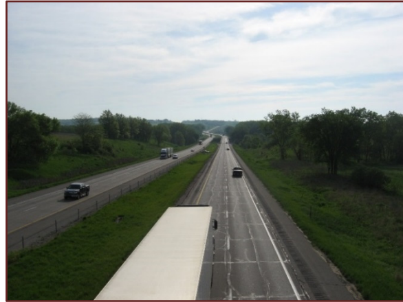
Photo 11. DALLAS COUNTY NEAR MP 112/NORTH RACCOON RIVER (FLOODING, HIGH TEMPERATURE CHANGE) – LOOKING EAST FROM OLD PORTLAND ROAD
