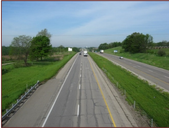
Photo 10. DALLAS COUNTY NEAR MP 111/SOUTH RACCOON RIVER (HIGH TEMPERATURE CHANGE) – LOOKING WEST FROM OLD PORTLAND ROAD
