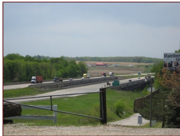
Photo 18. CEDAR COUNTY NEAR MP 266/CEDAR RIVER (FLOODING) – LOOKING WEST FROM 306 STREET
