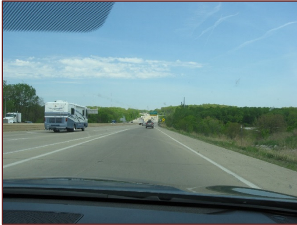
Photo 156. JOHNSON COUNTY NEAR MP 245 (BLIZZARD, ICING) – I-80 EASTBOUND LOOKING EAST
