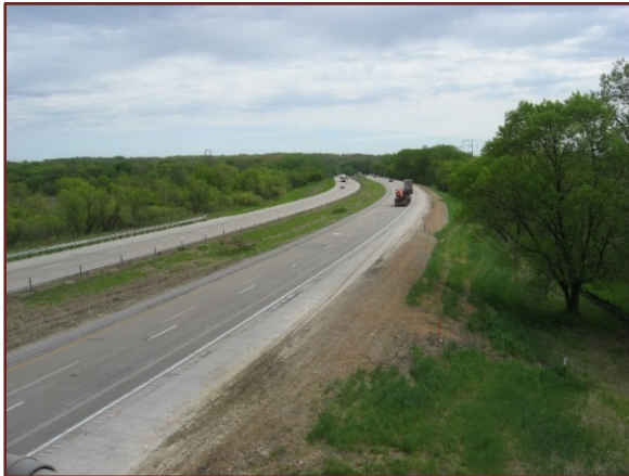
Photo 12. JASPER COUNTY NEAR MP 153/SOUTH SKUNK RIVER (FLOODING) – LOOKING EAST FROM W. 128 STREET OVERPASS
