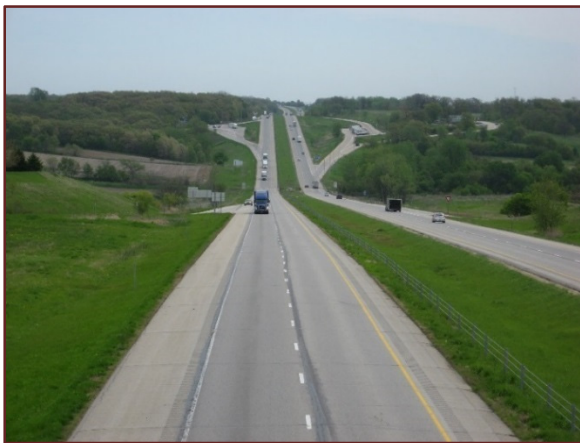
Photo 145. JASPER/POWESHIEK COUNTY NEAR MP 180 (BLIZZARD, ICING) - LOOKING EAST FROM T-39N OVERPASS
