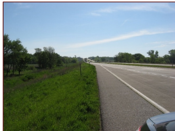
Photo 7. CASS COUNTY NEAR MP 61/EAST NISHNABOTNA RIVER (FLOODING, HIGH TEMPERATURE CHANGE) – LOOKING EAST FROM US 6/US 71 WESTBOUND EXIT RAMP
