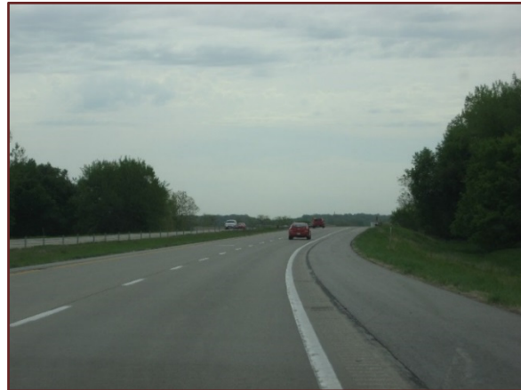
Photo 13. JASPER COUNTY NEAR MP 158/INDIAN CREEK (FLOODING) – I-80 EASTBOUND LOOKING EAST
