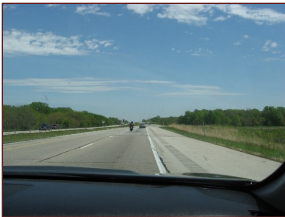
Photo 167. CEDAR COUNTY NEAR MP 266/CEDAR RIVER (FLOODING) – I-80 EASTBOUND LOOKING EAST
