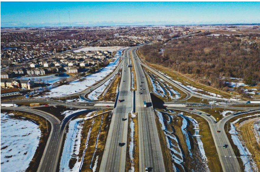
Diverging diamond interchange at I-35 and 1st Ave. in Ankeny. (Source: Iowa DOT)
