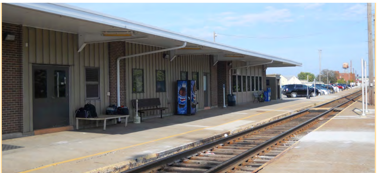
Figure 2.10: Fort Madison Station
